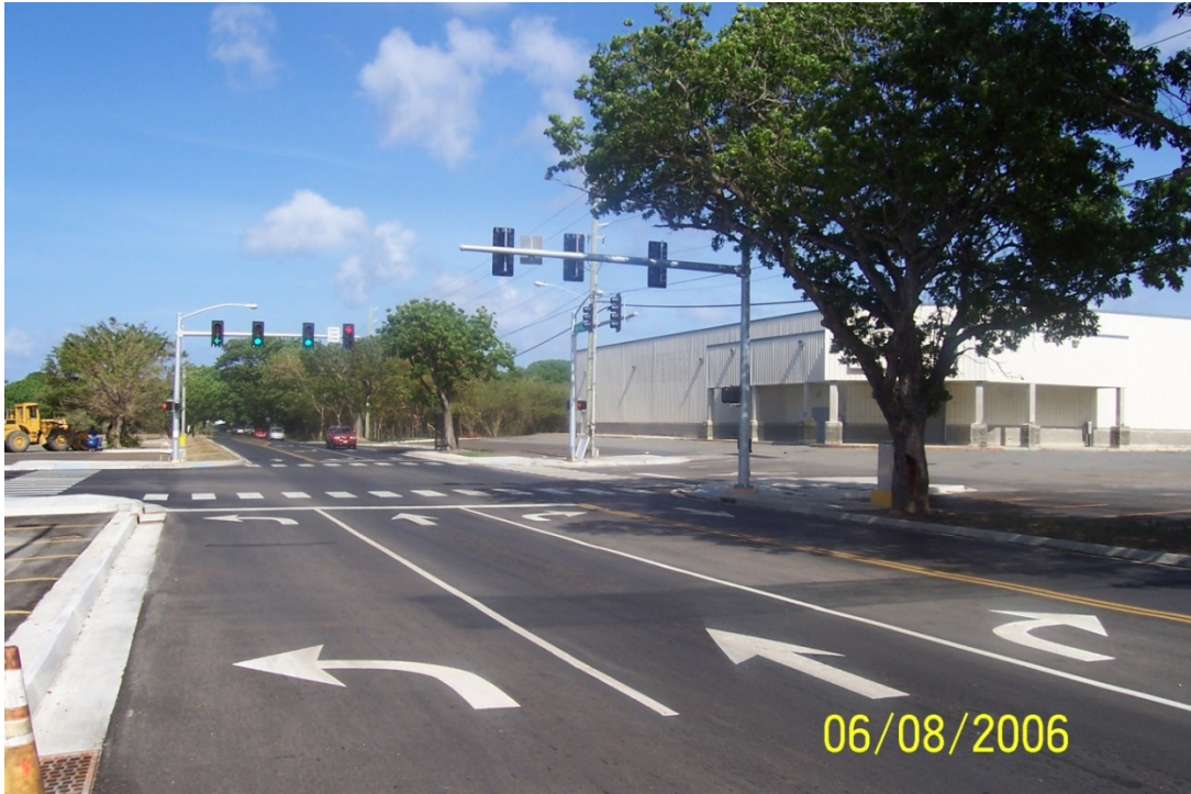
Queen Mary Highway, Station 19+50 Rt. (West Bound) – After
