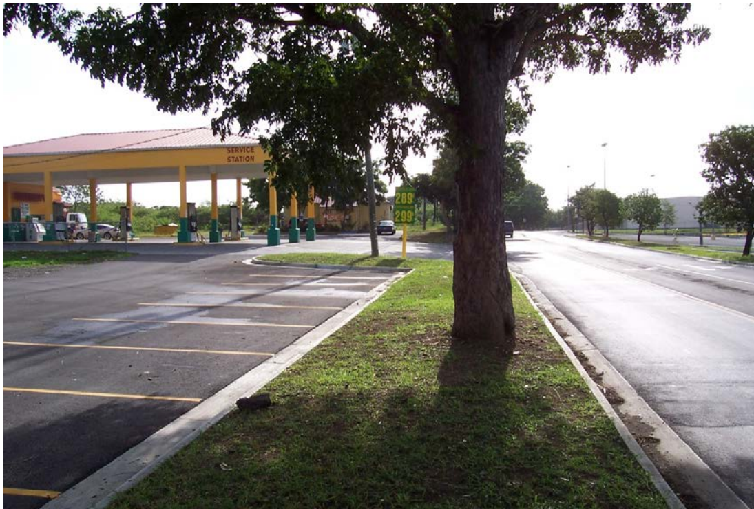
Queen Mary Highway, Island at Station 18+75 Lt. (East Bound) - After
