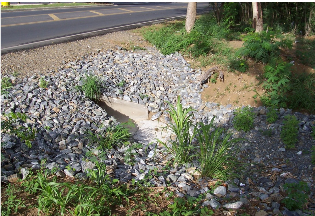
Queen Mary Highway, New 24" Pipe Culvert and End Section at Station 18+00 Rt. (West Bound) - After
