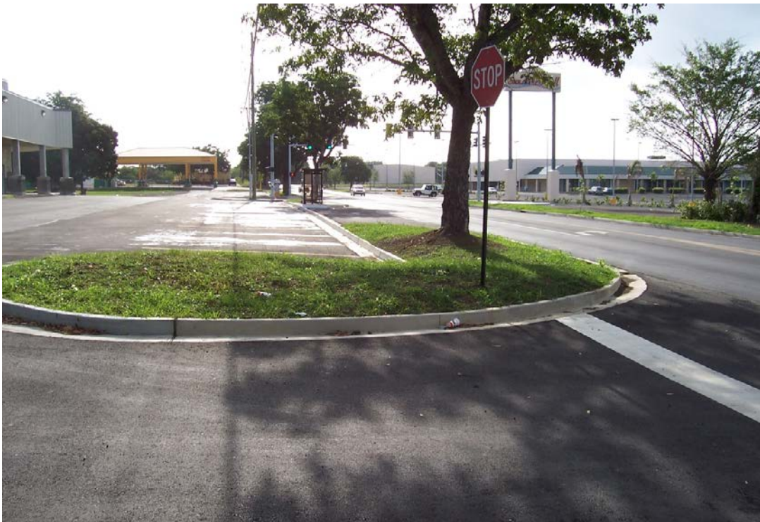
Queen Mary Highway, Island at Station 15+50 Lt. (East Bound) - After
