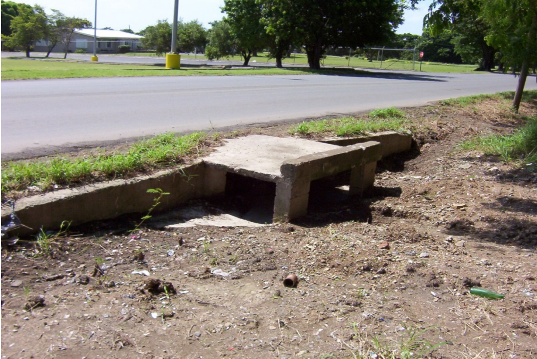
Queen Mary Highway, Existing Culvert at Station 14+75 Rt. (West Bound) – Before
