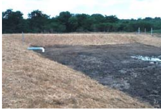
New pond, spillway, embankments and fencing on December 28, 2005.
