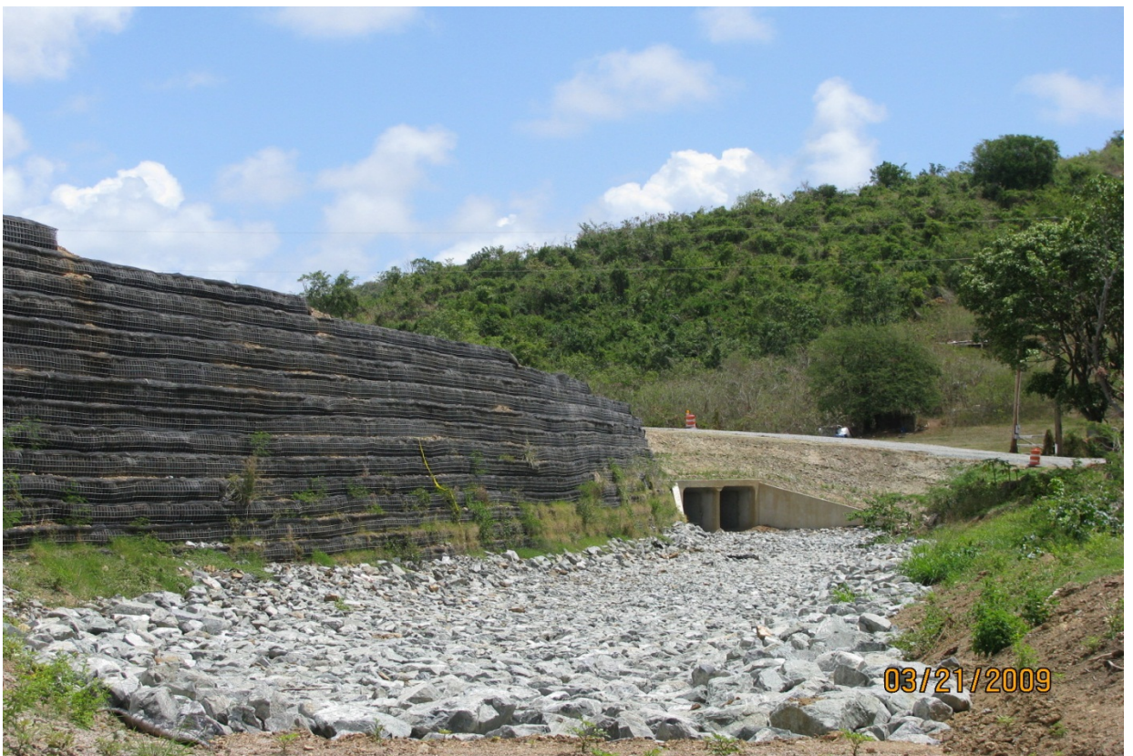
MECHANICALLY STABILIZED EARTH WALL COMPLETE
