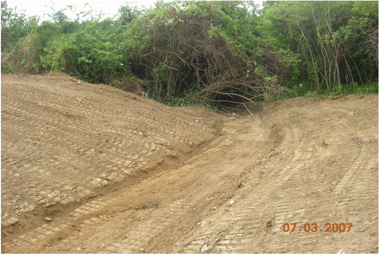
PREPARING DIVERSION CHANNEL
