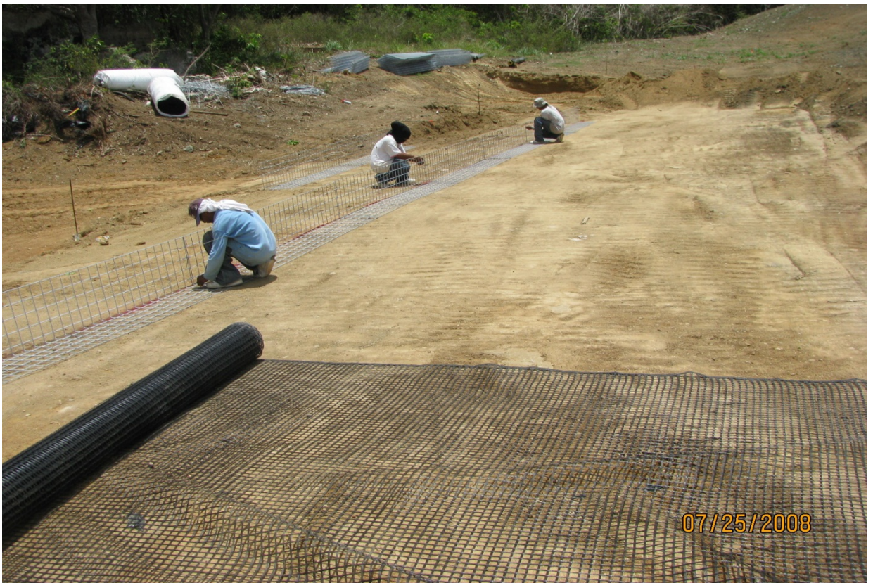
MECHANICALLY STABILIZED EARTH WALL PREPARATION
