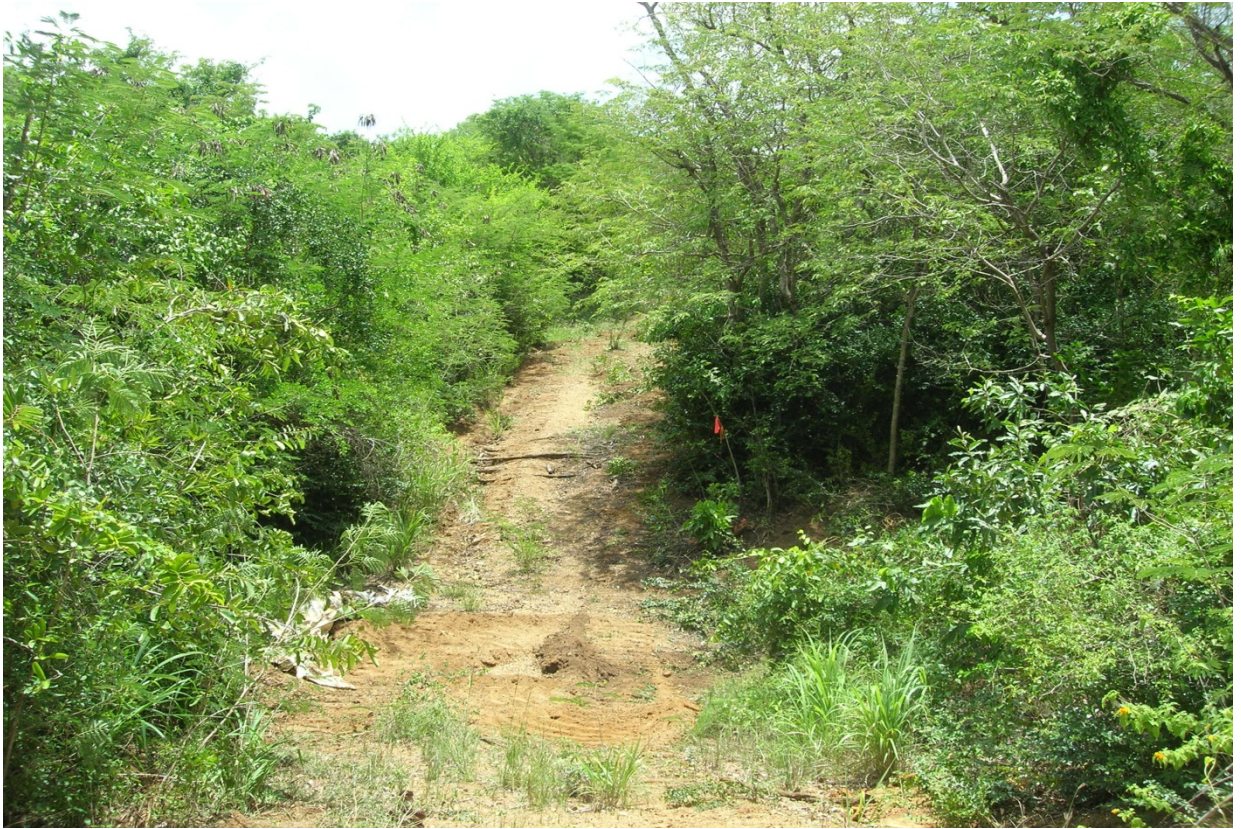
STATION 48+50 PRIOR TO CONSTRUCTION
