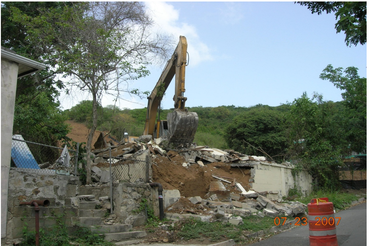
STATION 60+00 BUILDING DEMOLITION
