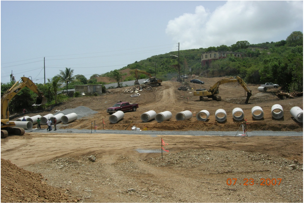
STATION 53+09 STAGING FOR 42-INCH REINFORCED CONCRETE PIPE
