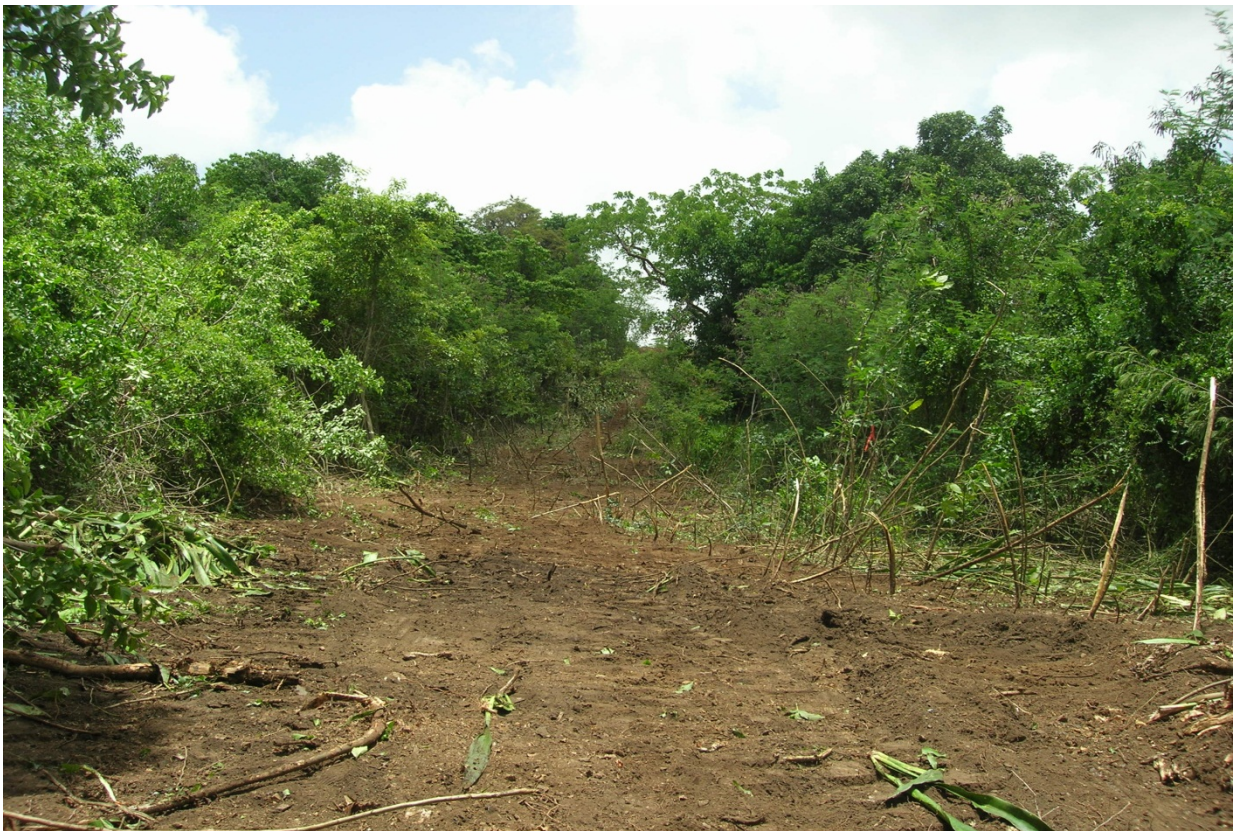
STATION 53+00 WEST PRIOR TO CONSTRUCTION
