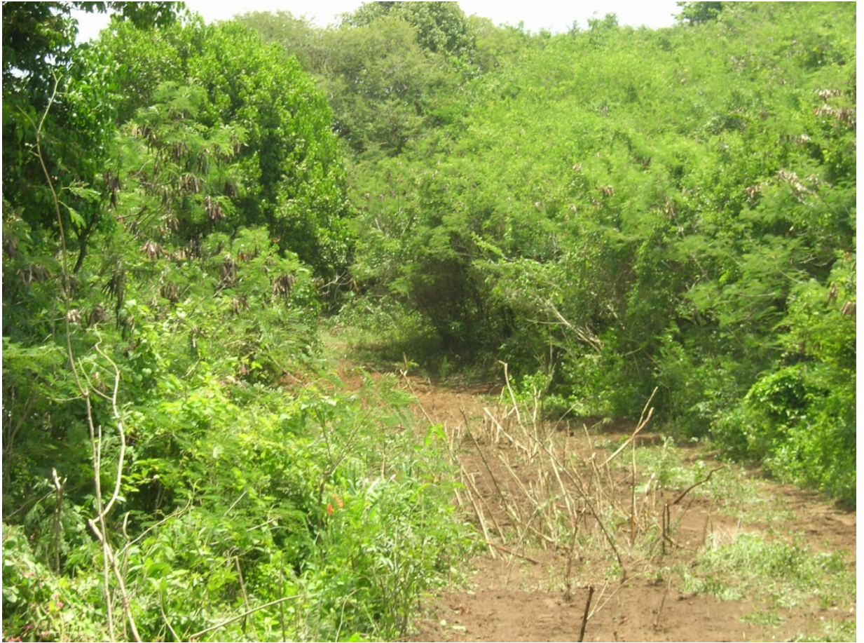
STATION 42+00 PRIOR TO CONSTRUCTION
