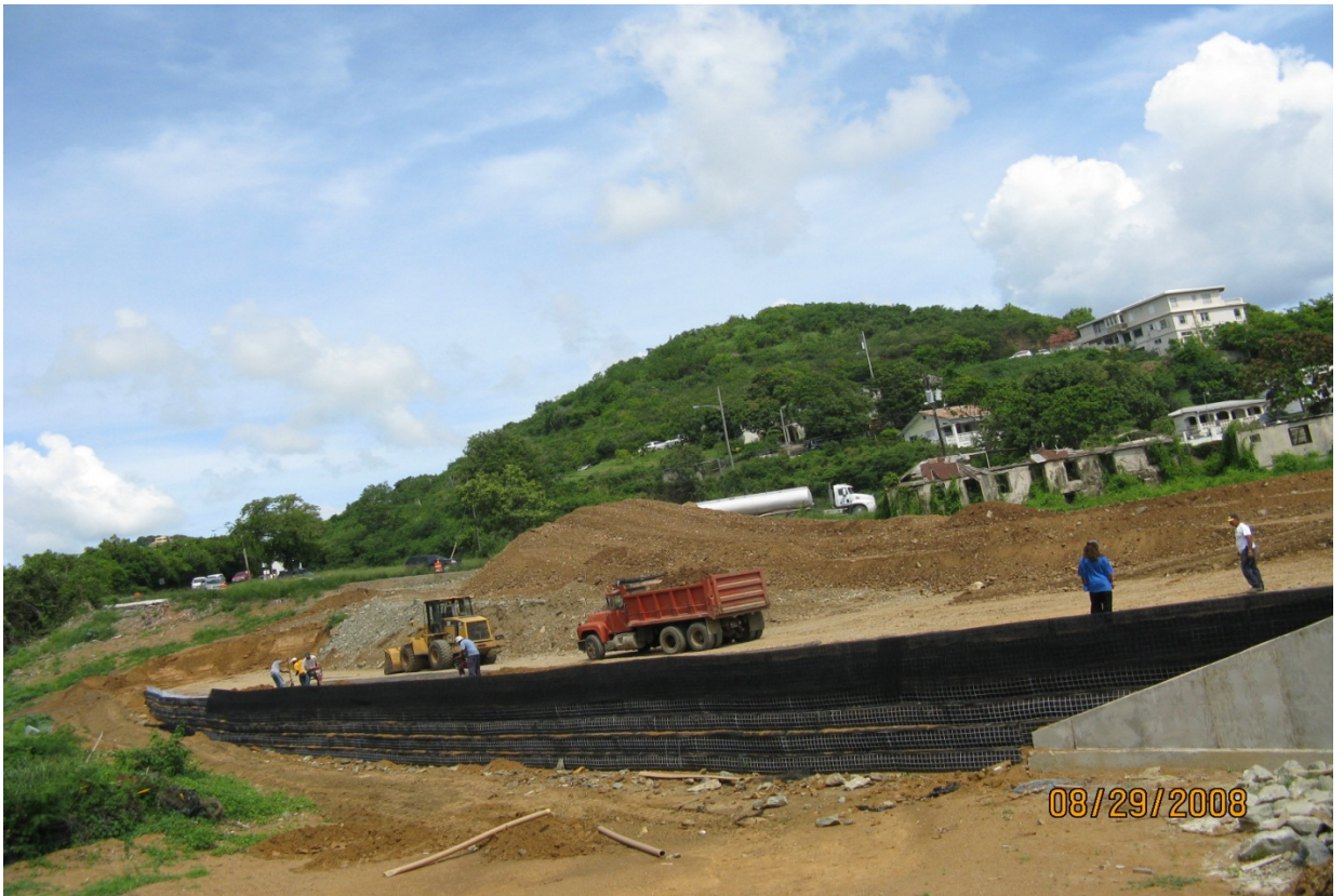
MECHANICALLY STABILIZED EARTH WALL IN PROGRESS
