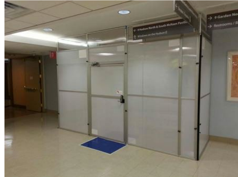
ICRA Containment Barriers
