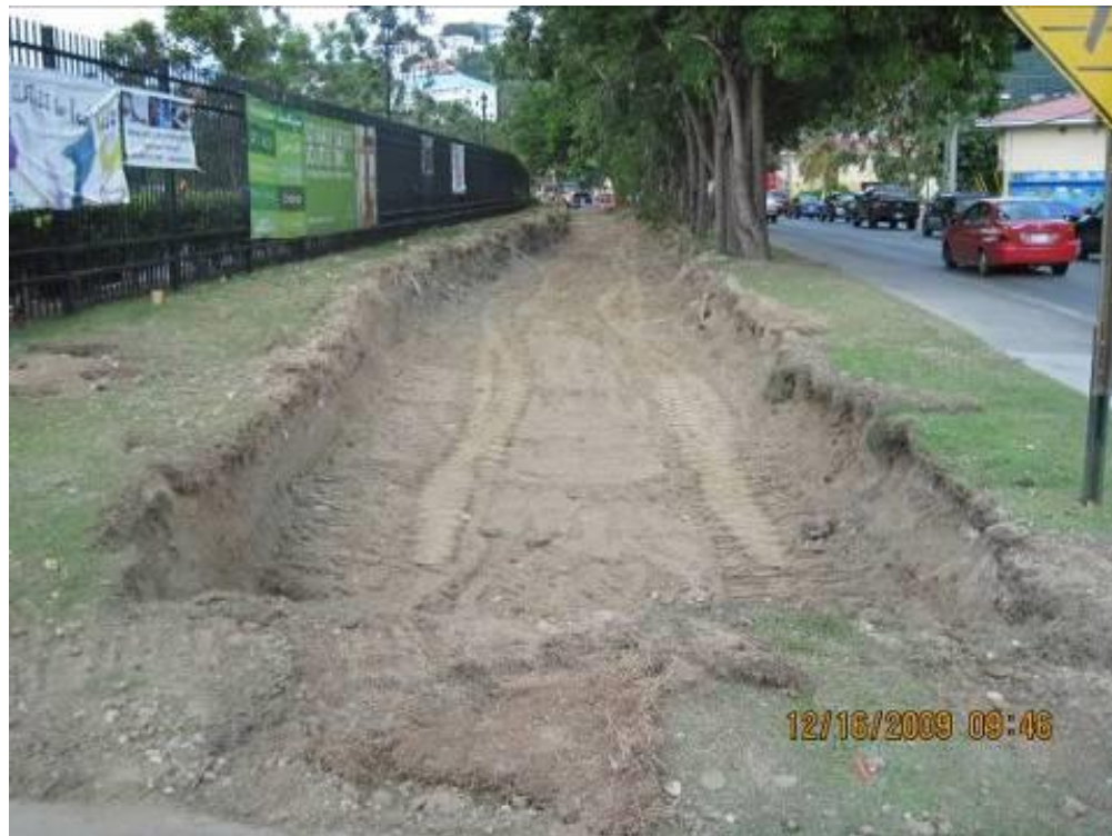
Picture 2. Contractor, Island Roads Corporation (IRC) begins project construction with roadway excavation on South side of Long Bay Road (LBR) in front of Yacht Heaven Grande (YHG). Two new paved lanes (on South side of existing roadway), re-route traffic through new lanes, removal and reconstruction of two existing lanes, curb and sidewalk on North side, new concrete curb, sidewalk, bus shelters, landscaped median, underground drainage system, underground utilities relocation, concrete box culvert, traffic signal and street lights systems are to be constructed as part of the Long Bay Road Improvements Project.
