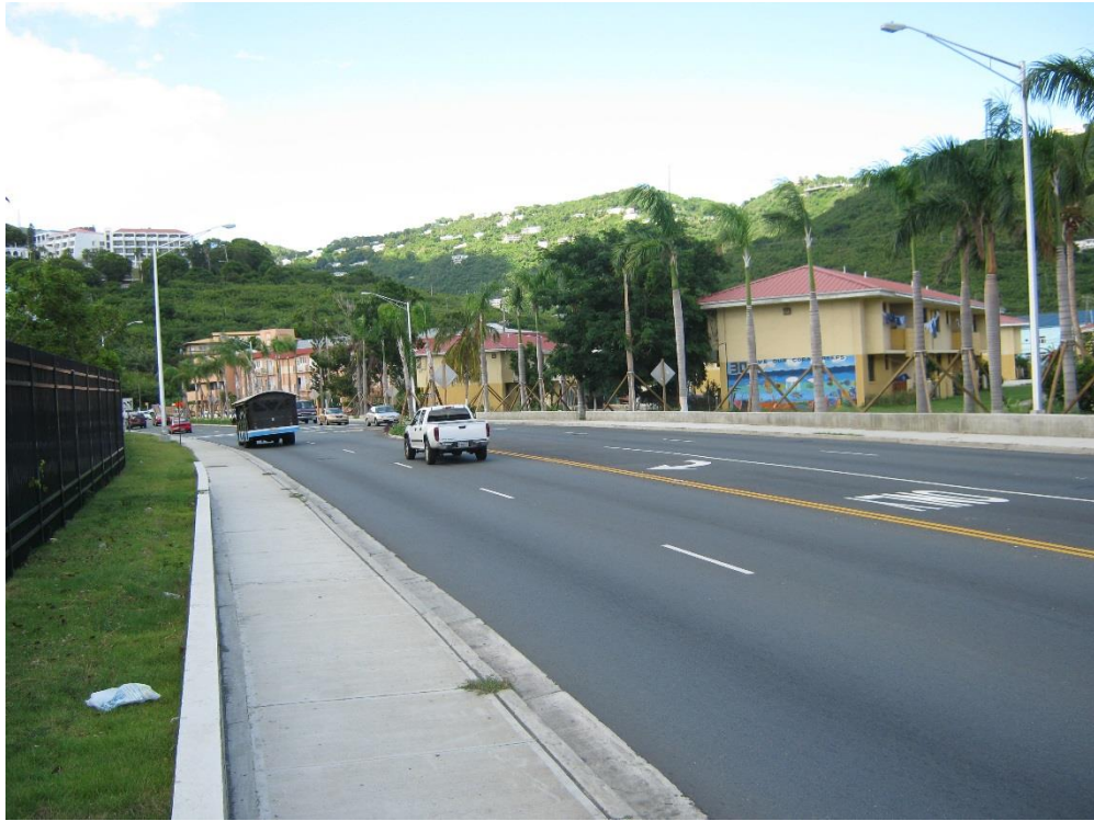
Picture 31. Completed project. View from the Right (South) side of LBR at station 25+00R looking West
