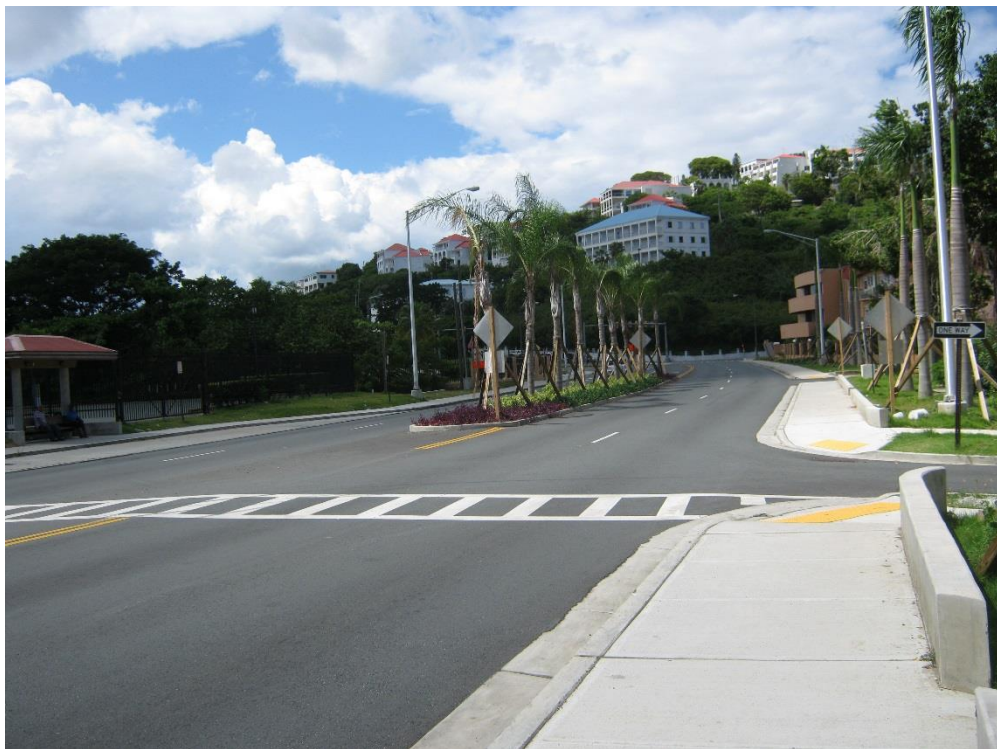
Picture 32. Completed project. View from the Left (North) side of LBR at station 23+00L looking West
