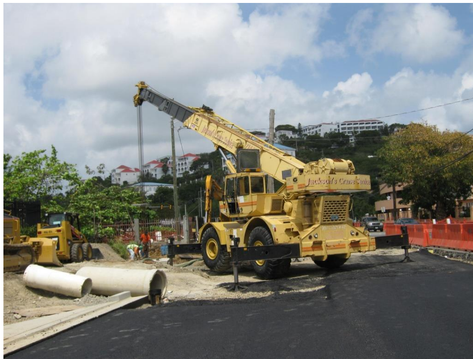
Picture 8. Station 20+50R (South side of LBR) Contractor, IRC, after removing existing concrete box culvert proceeded to install new precast 8'x3' reinforced concrete box culvert on the South side of LBR
