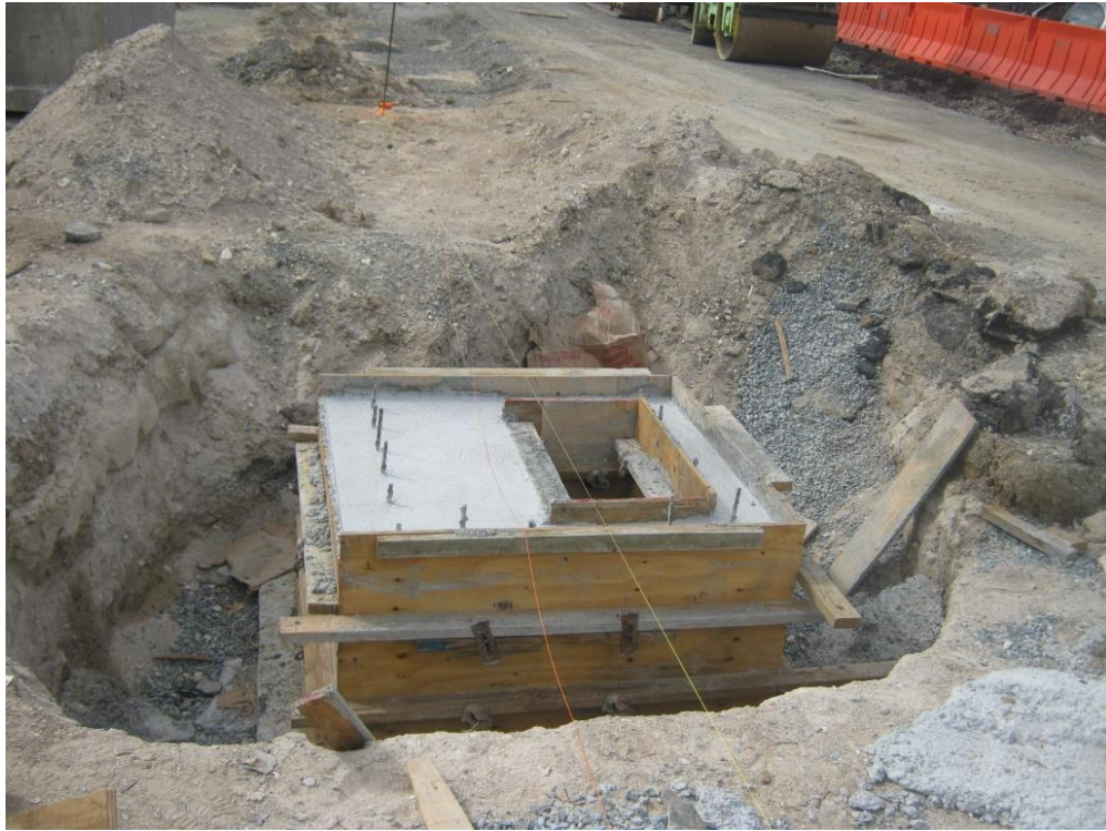
Picture 11. Subcontractor, Ri-Tech Inc works on underground drainage and Utility systems along the South side of LBR.
