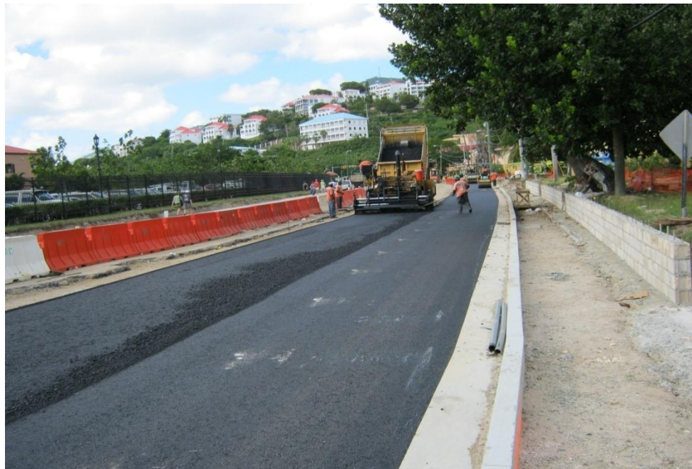
Figure 28. Contractor, IRC, seeing placing Hot Asphalt Concrete Pavement, Marshall Test, Class B, Grading A, (HACP) Binder Course, first 3-inch layer (total 6-inch), on the north lanes (eastbound) of LBR. View from station 24+50L looking West
