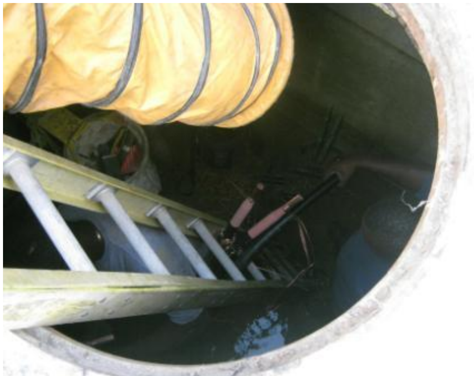
Picture 12, Utility Owners work on underground utilites connecting cables, Swith boxes, risers, service, manholes, etc.
