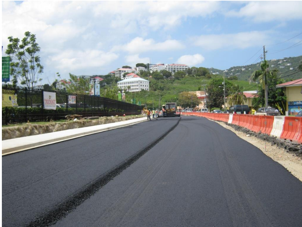
Picture 19. Contractor, IRC seeing placing base asphalt pavement along the Right (South) two lanes of LBR in order to relocate traffic to the two new lanes and begin work on the median and Left (North) side of LBR
