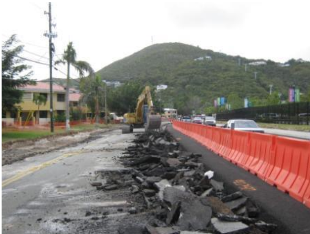
Picture 20. After relocating traffic to the Right (South) two lanes, Contractor proceeded to remove asphalt pavement, sidewalk, curb and gutter along the Left (North) side of LBR in front of YHG. View from about station 23+00L looking East
