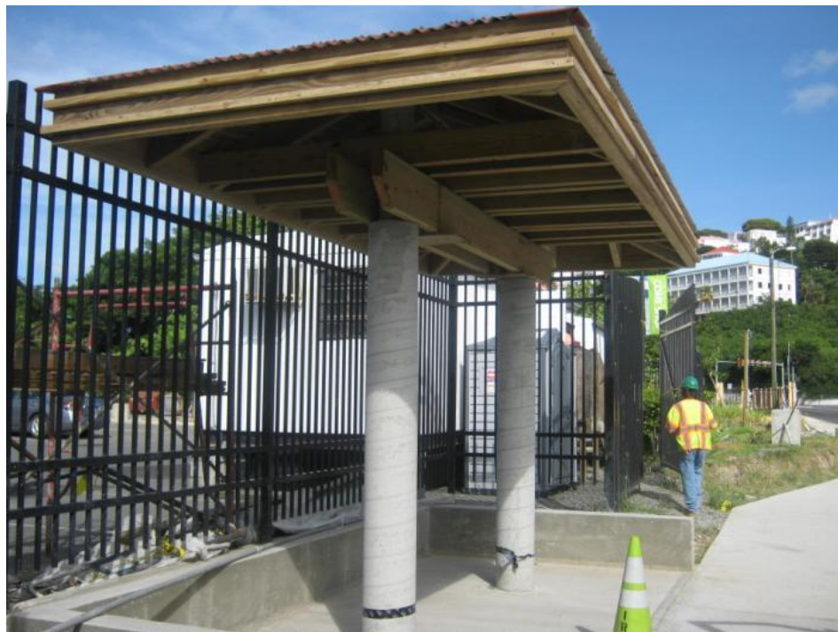
Picture 30. Contractor completed bus shelters along the Right (South) side of LBR view at station 21+50R
