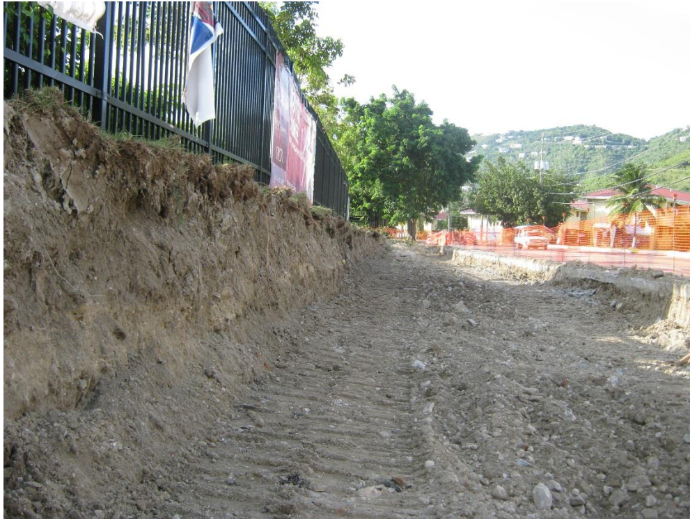
Picture 5. Contractor, IRC, begins project construction with roadway excavation on South side of LBR in front of YHG. View from about station 28+00R looking West
