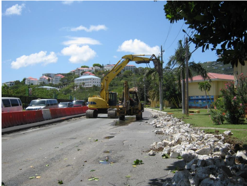
Picture 21. After relocating traffic to the Right (South) two lanes, Contractor proceeded to remove asphalt pavement, sidewalk, curb and gutter along the Left (North) side of LBR in front of Pearson Gardens Housing Authority Property. View from about station 25+00L looking West
