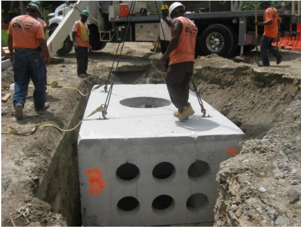
Picture 15. Contractor, IRC seeing installing precast reinforced concrete utilities manholes
