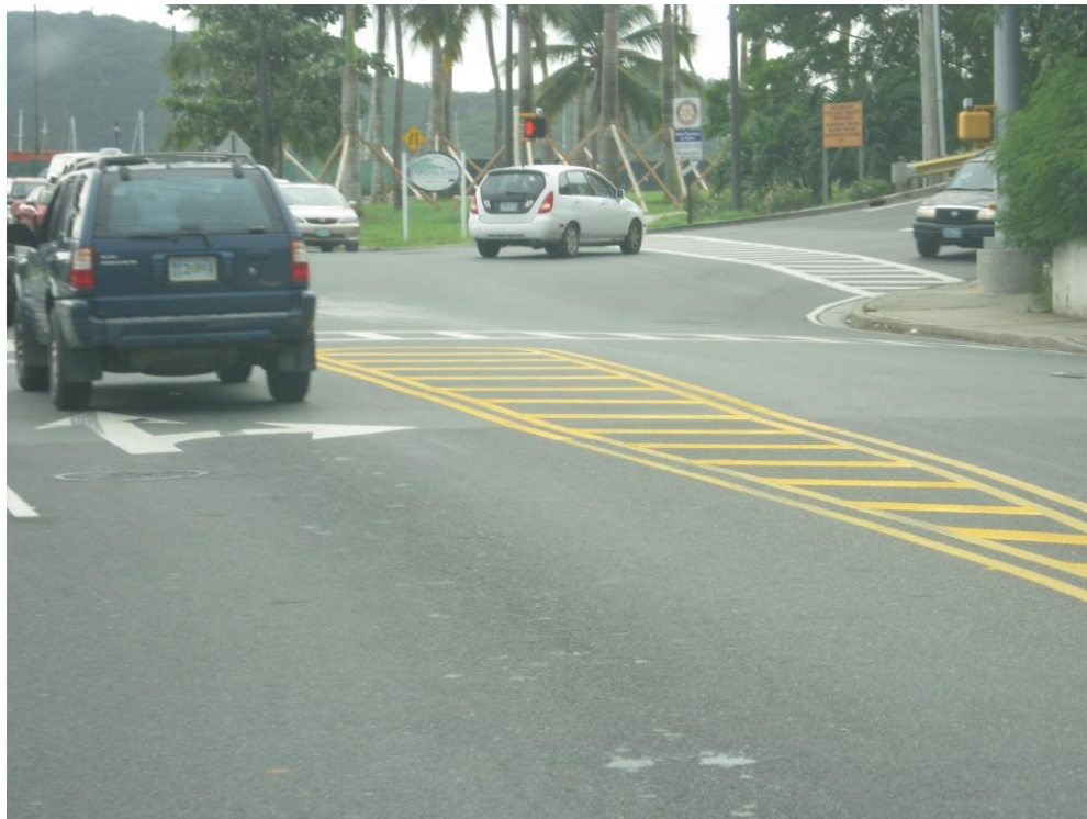
Picture 34. Completed project at the intersection of LBR-Lovers-Lane-Veterans Drive-De Beltjem Rd. View from Lover's Lane looking South to Veterans Drive.
