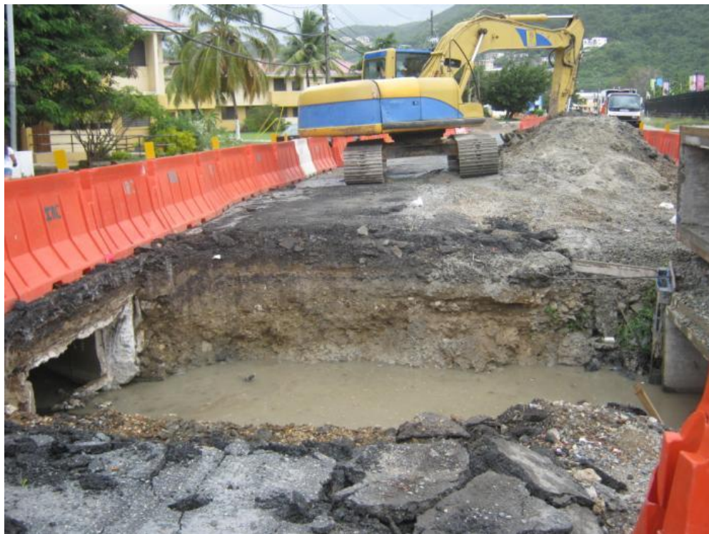
Picture 22. Contractor, IRC seeing removing existing reinforced concrete box culvert on the Left (North) side of LBR at about station 20+50L
