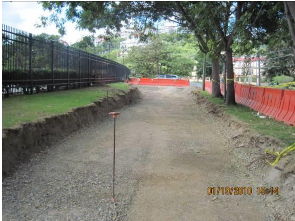
Picture 3. Contractor, IRC, begins project construction with roadway excavation on South side of LBR in front of YHG. View from station 20+50R looking West
