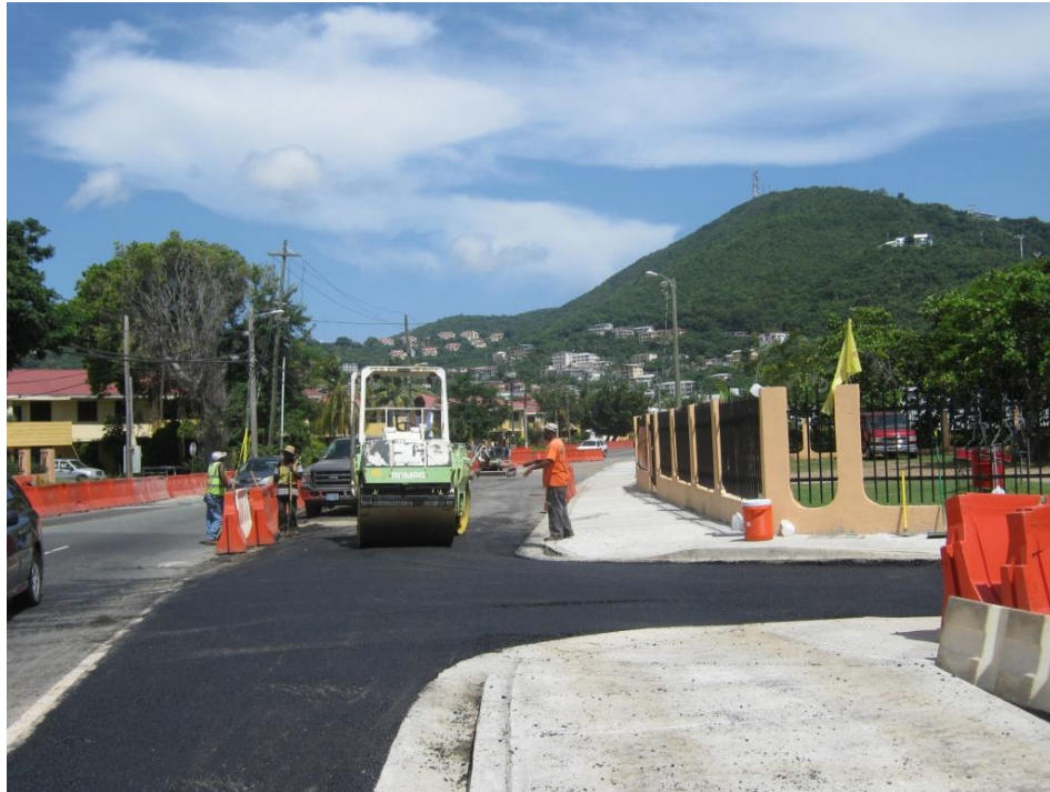
Picture 29. Contractor, IRC, after completion of sidewalk, curb and gutter and new concrete wall proceeded to pave VIPD impounding lot driveway on the Right (South) side of LBR between stations 18+00R and 19+50R
