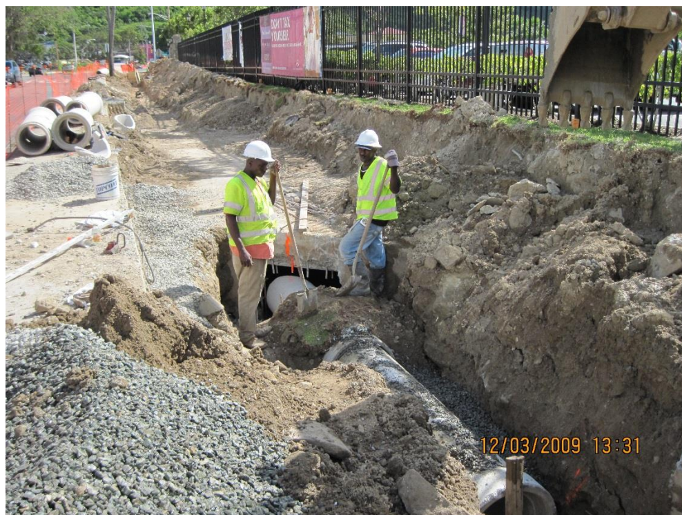
Picture 6. Subcontractor, Rinstalling reinforced concrete pipe culverts along the South side of LBR in front of YHG. View from about station 27+70R looking East
