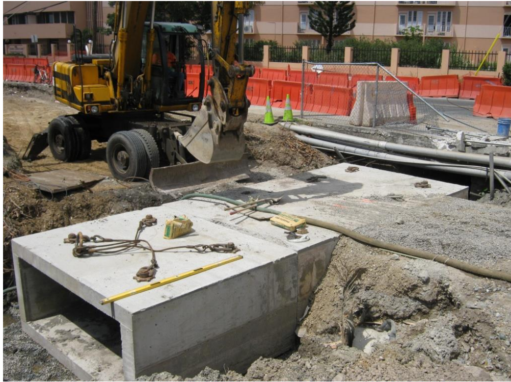
Picture 7. Station 20+50R (South side of LBR) Contractor, IRC, after removing existing concrete box culvert proceeded to install new precast 8'x3' reinforced concrete box culvert on the South side of LBR
