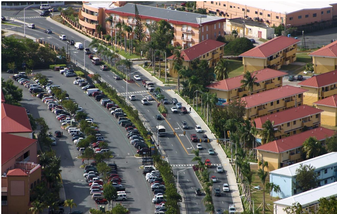
Picture 40. View of completed project West end (Lovers Lane Intersection of Veterans Dr, Lovers Lane, De Beltjem Rd and LBR) from up the hill above Frenchmans Bay Road looking West
