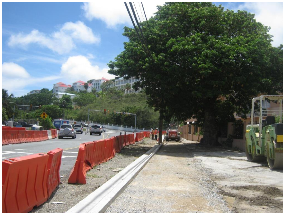
Picture 26. Contractor working on the Left (North) side of LBR on construction underground utilities, drainage, Street light and Traffic signal System, concrete curb and gutter, sidewalk, etc.
