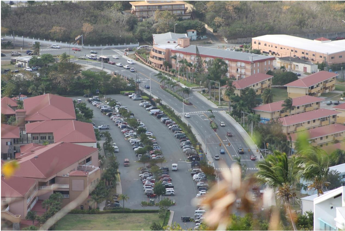
Picture 39. View of completed project West end (Lovers Lane Intersection of Veterans Dr, Lovers Lane, De Beltjem Rd and LBR) from up the hill above Frenchmans Bay Road looking West
