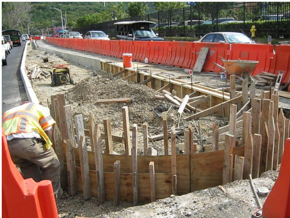
Picture 24. Subcontractor Ri-Tech seeing building concrete curb for middle island on LBR. View from station 26+35 looking East
