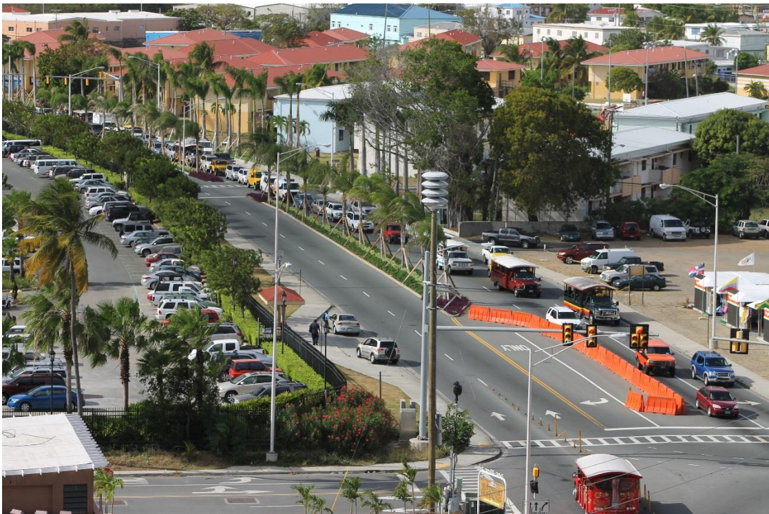
Picture 38. View of completed project East end (Mandela Circle Intersection of Centerline Rd. (CLR), CLR extension, Frenchman Bay Road and LBR) from up the hill above Frenchmans Bay Road looking West
