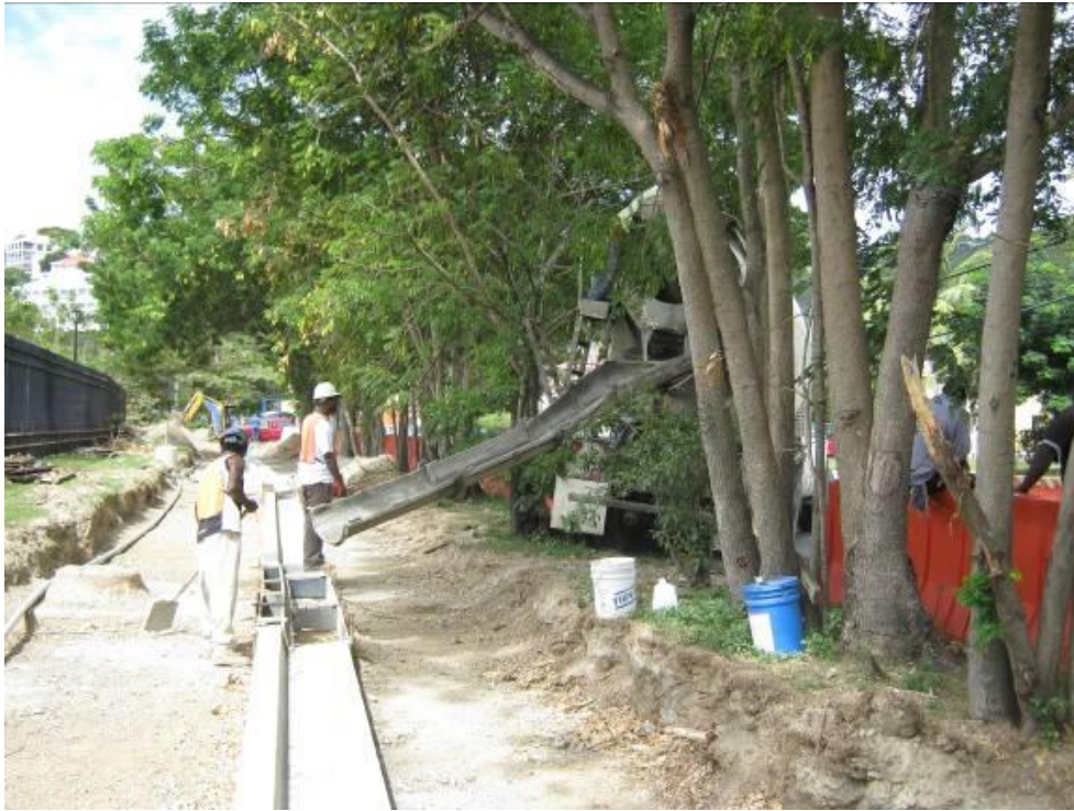
Picture 17. Subcontractor, Ri-Tech Seeing pouring new type 3 catch basin along the Right (South) side of LBR in front of YHG. View from about station 24+00 looking West
