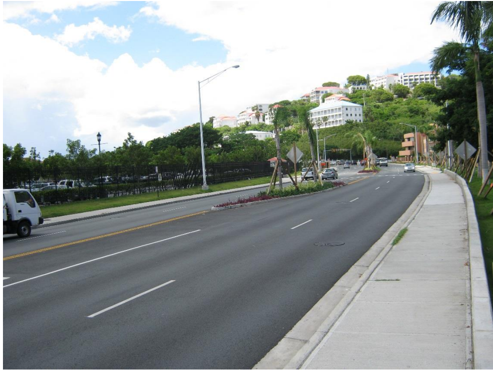
Picture 33. Completed project. View from the Left (North) side of LBR at station 25+00L looking West
