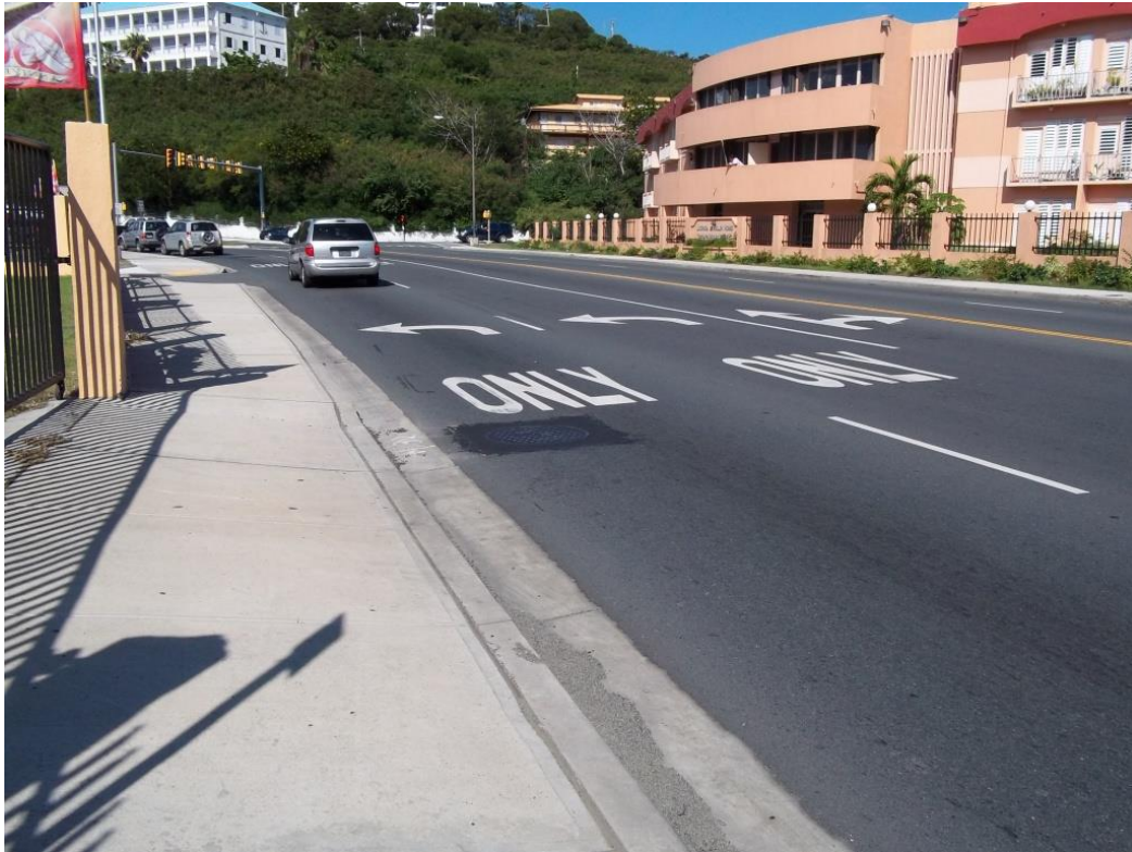
Picture 37. View of completed project at the Lovers Lane intersection of LBR, Veterans Drive, Lovers Lane and De Beltjem Rd. View from the Right (South) side of LBR station 20+20R looking West
