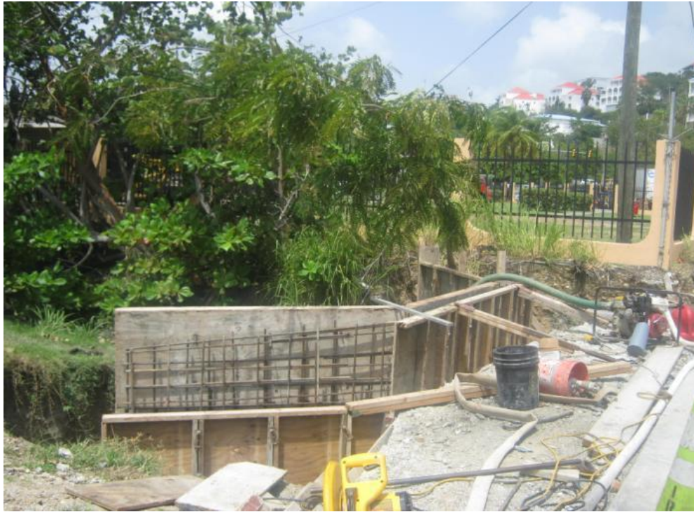
Picture 9. Station 20+50R (South side of LBR), Contractor, IRC, after removing existing concrete box culvert proceeded to install new precast 8'x3' reinforced concrete box culvert on the South side of LBR with new reinforced concrete wing walls on the outfall (South) side and will be attached to existing 8'x3' RC Box Culvert on the North side
