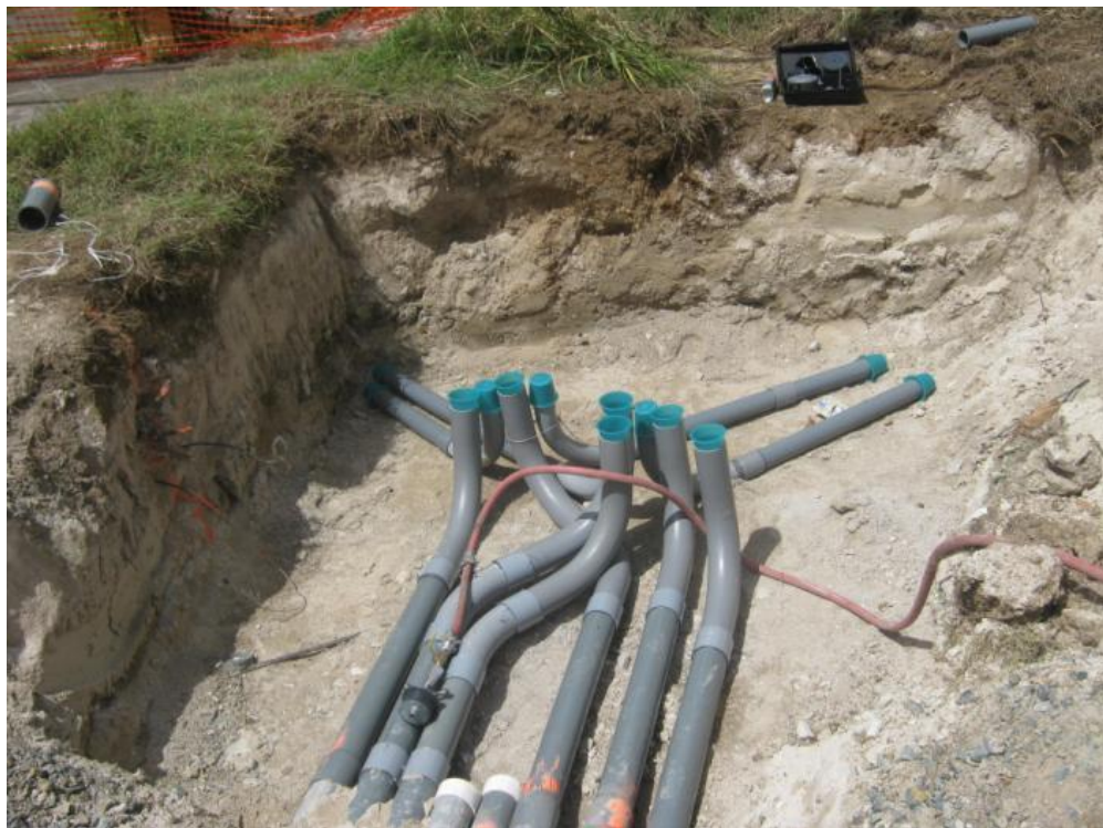
Picture 14. Contractor seeing installing underground conduits for installation of new traffic signal at the main entrance to YHG
