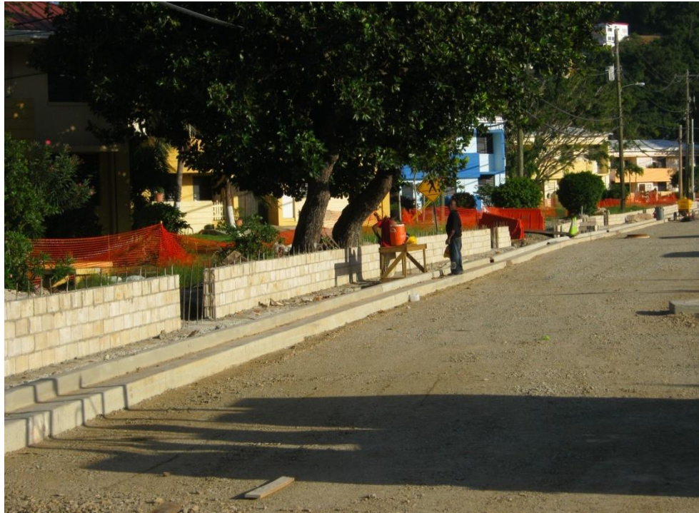
Picture 27. Subcontractor Ri-Tech seeing building reinforced concrete block wall along the Left (North) side of LBR in front of their front of Pearson Gardens Housing Authority Property
