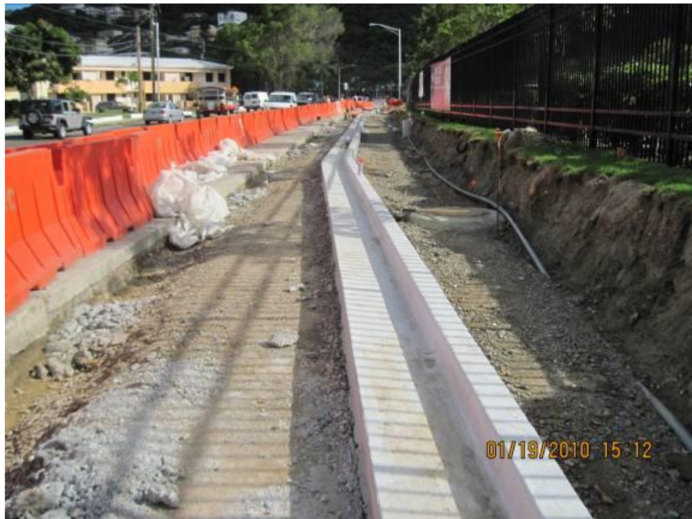
Picture 16. Subcontractor, Ri-Tech completed curb and gutter along the Right (South) side of LBR in front of YHG. View from about station 27+00 looking East
