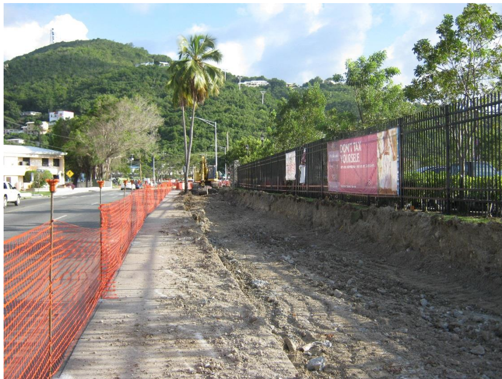
Picture 4. Contractor, IRC, begins project construction with roadway excavation on South side of LBR in front of YHG. View from station 27+70R looking East
