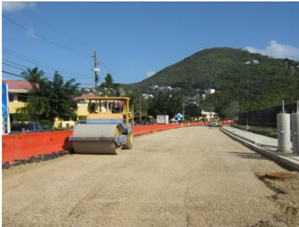
Picture 18. Sucontractor Ri-Tech completed concrete sidewalk, curb and gutter along the South side of LBR and A9 Trucking is seeing placing and compacting aggregate base.
