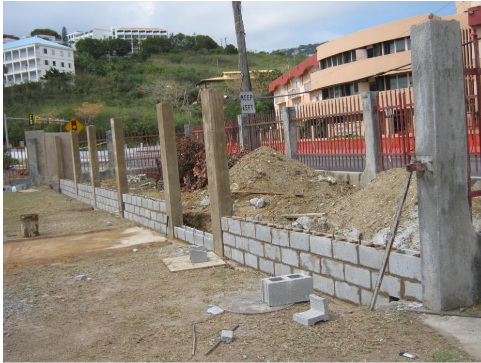
Picture 25. Subcontractor Ri-tech seeing relocating the concrete fence for the US VI Police Department Impounding Lot.
