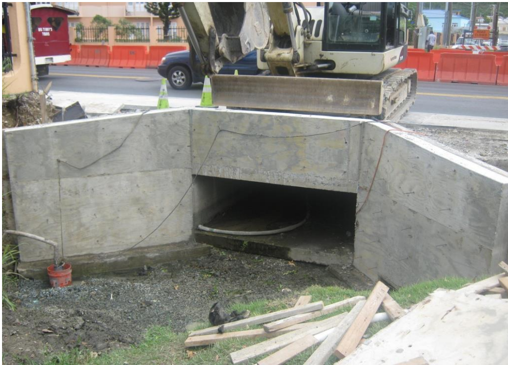
Picture 10. Station 20+50R (South side of LBR), Contractor, IRC, after removing existing concrete box culvert proceeded to install new precast 8'x3' reinforced concrete box culvert on the South side of LBR with new reinforced concrete wing walls on the outfall (South) side and will be attached to existing 8'x3' RC Box Culvert on the North side
