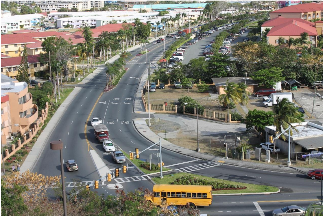
Picture 41. View of completed project West end (Lovers Lane Intersection of Veterans Dr, Lovers Lane, De Beltjem Rd and LBR) from up the hill above De Beltjem Rd looking East
