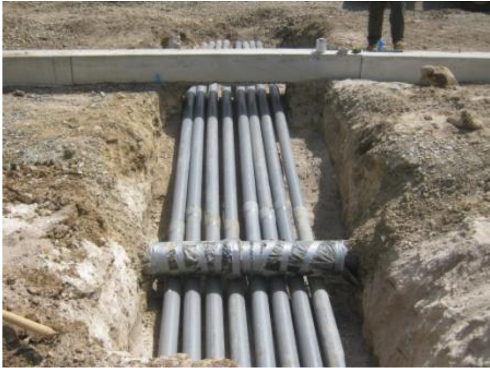
Picture 13. Contractor, IRC, seeing installing new underground communications ductbank below ductile iron waterline and electrical ductbank.
