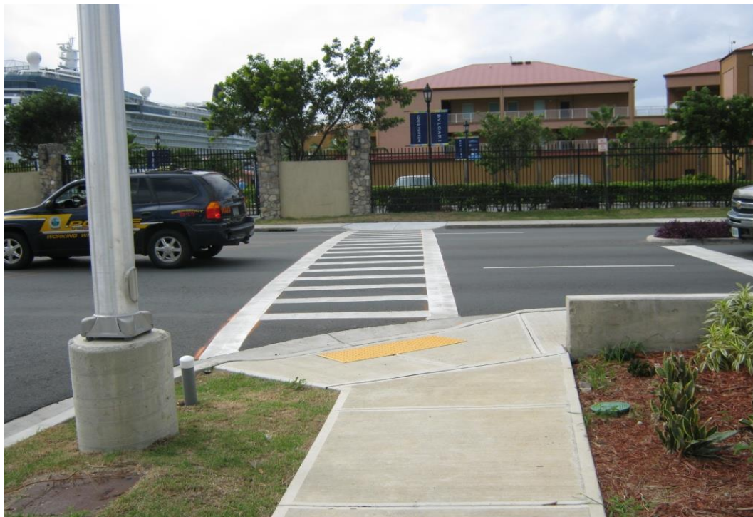
Picture 36. New Crosswalk requested by the VI Department of Public Works (DPW) at the exit of Pearson Gardens Housing Project station 29+50 and placed by subcontractor Precise Builders
