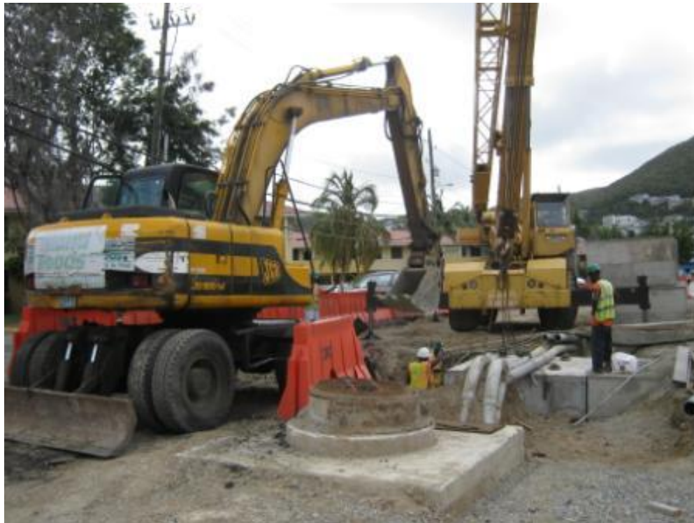
Picture 23. IRC works on underground drainage and Utility systems along the North side of LBR. View from station 20+20L looking East
