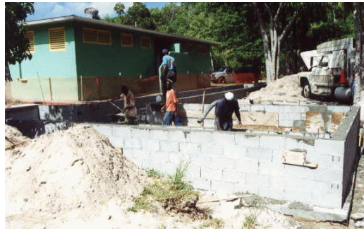
AOSDS trenches were built with cinder blocks. Sand was then backfilled around the structure.
