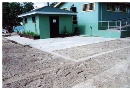
The subterranean trench style AOSDS at the Magens Bay bathhouse (before planting) is unobtrusive in the landscape.
