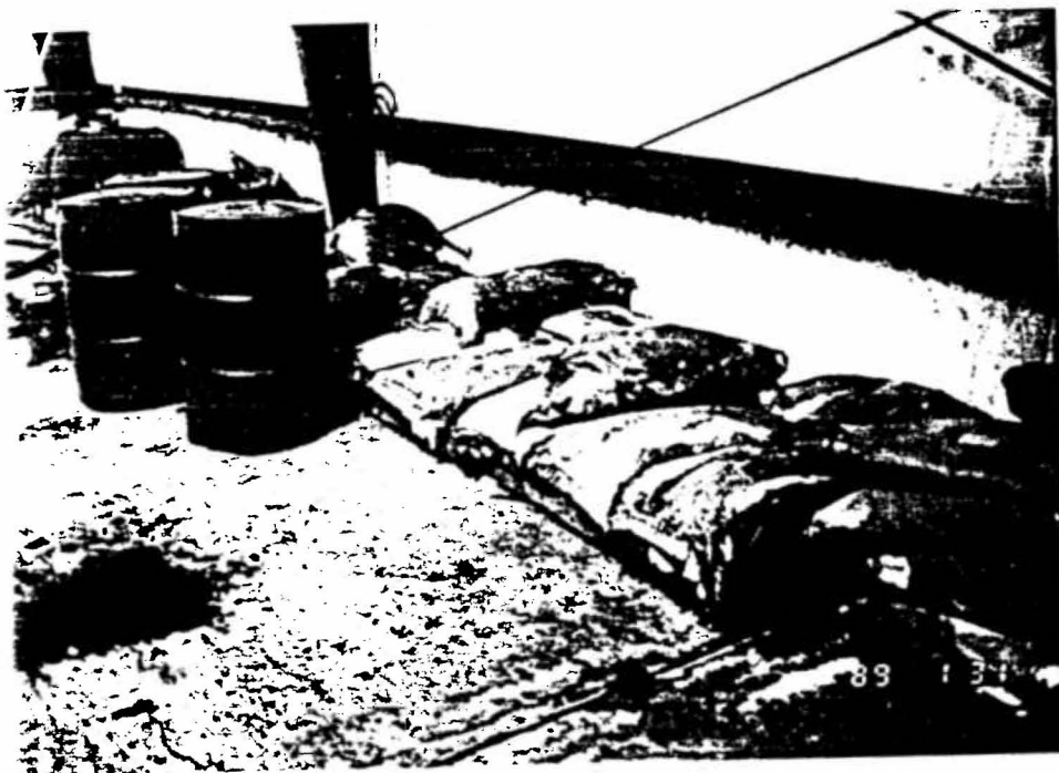
Photo #21. Deteriorating bags in area 6
