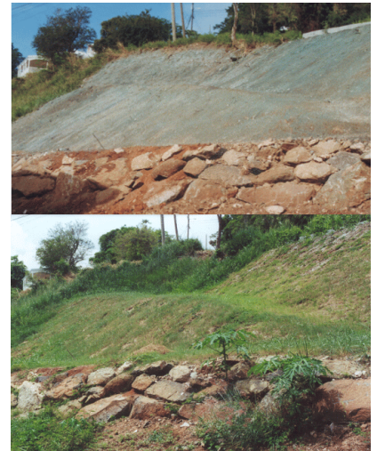
Home hydroseeding site when seeded (above) and after 2 months growth (below).
