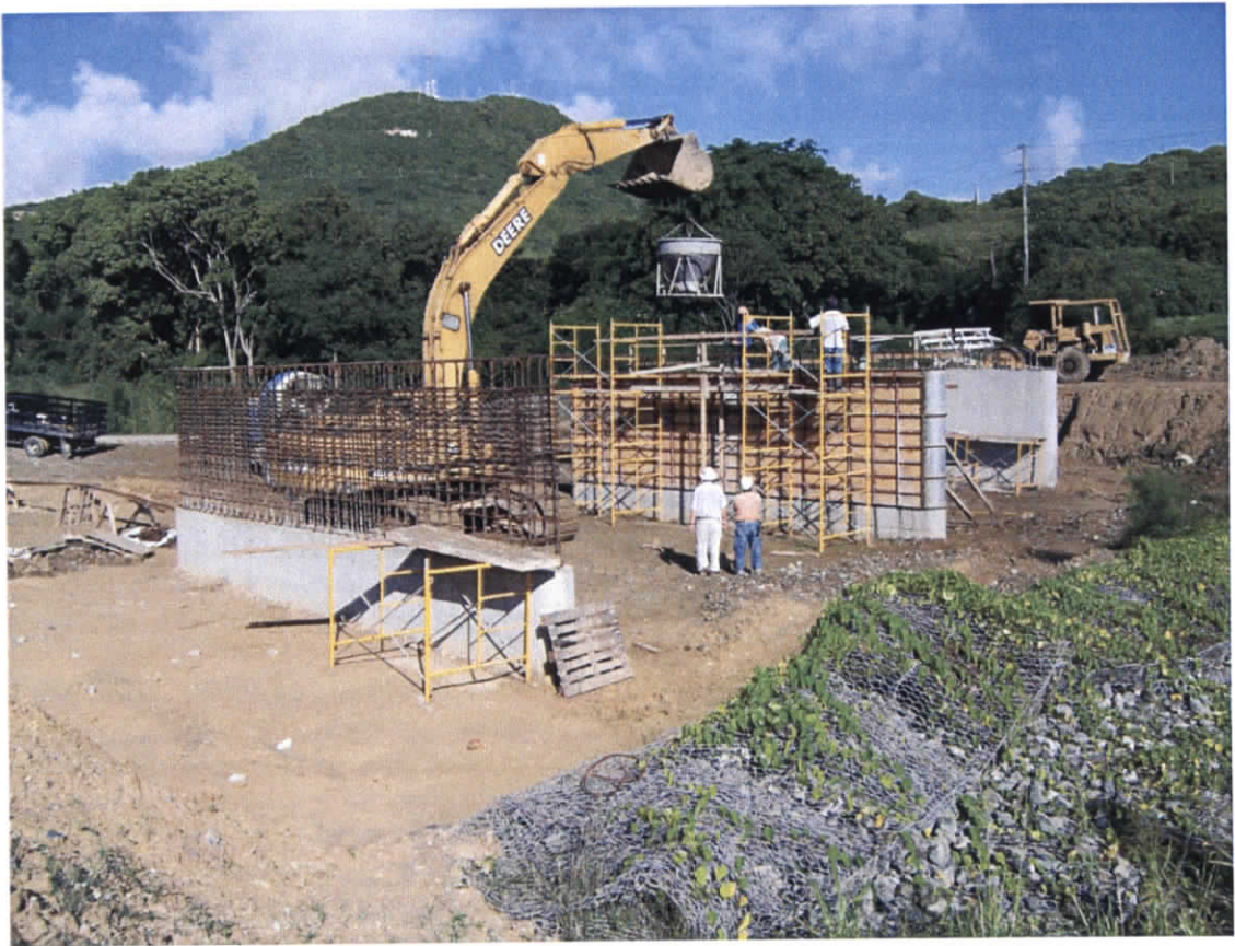
Hwy. 73 Bridge Pier Construction
