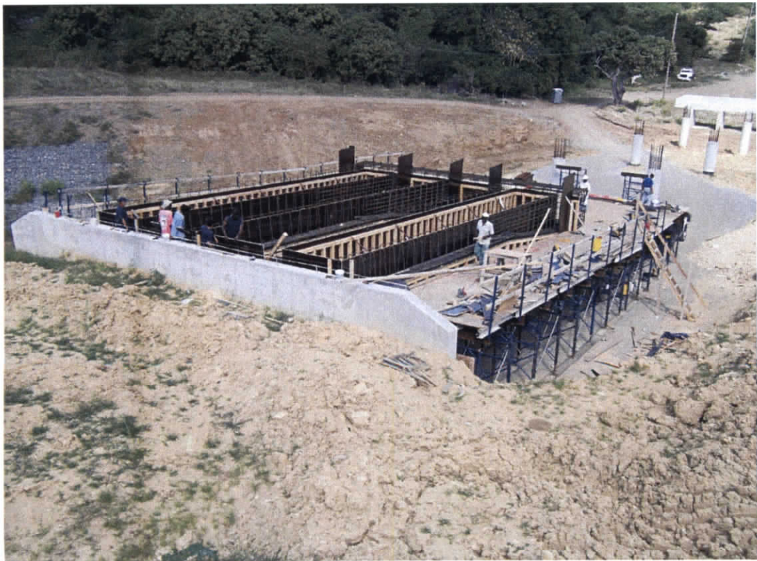
Glynn Road Bridge Beam Construction
