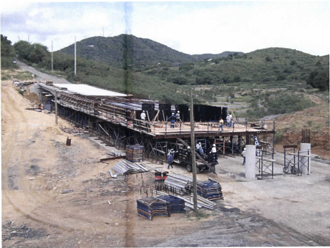
Glynn Rd. Bridge Deck Construction
