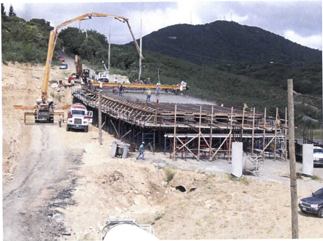
Glynn Rd. Bridge Deck Construction
