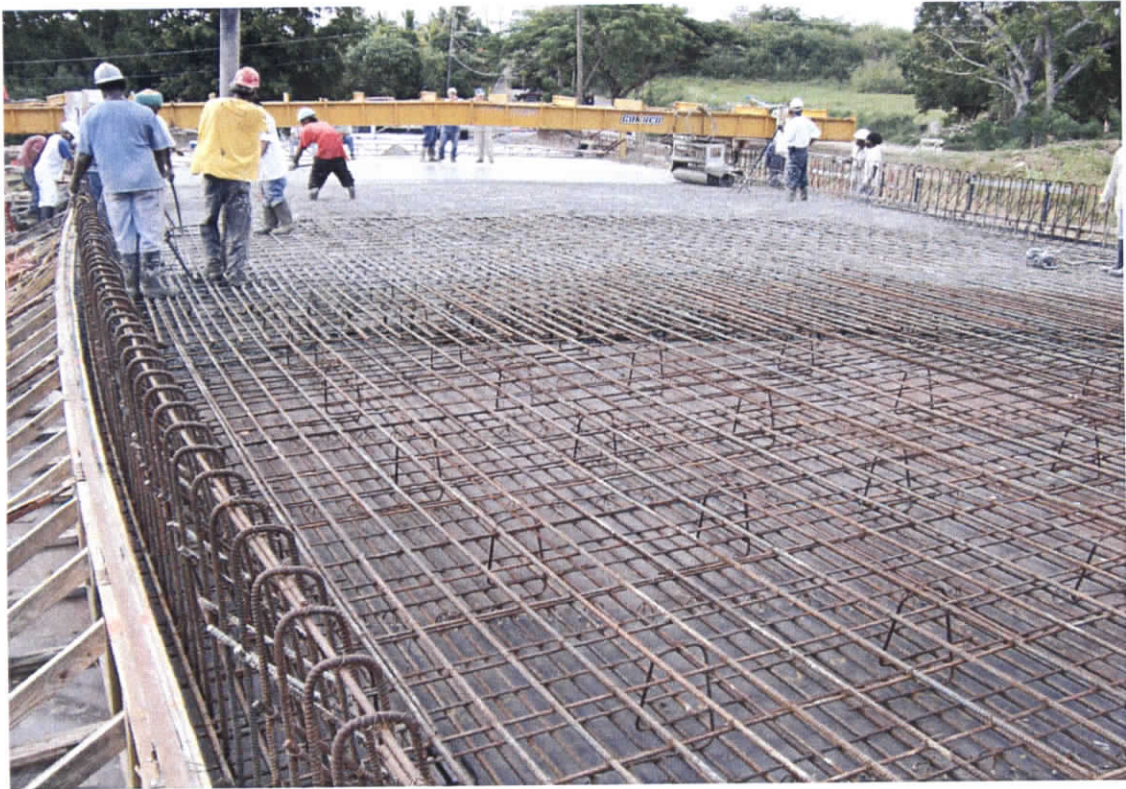
Hwy. 73 Bridge Deck Construction
