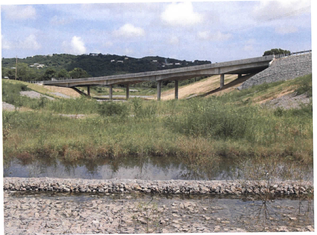
Glynn Rd. Bridge Final Product
