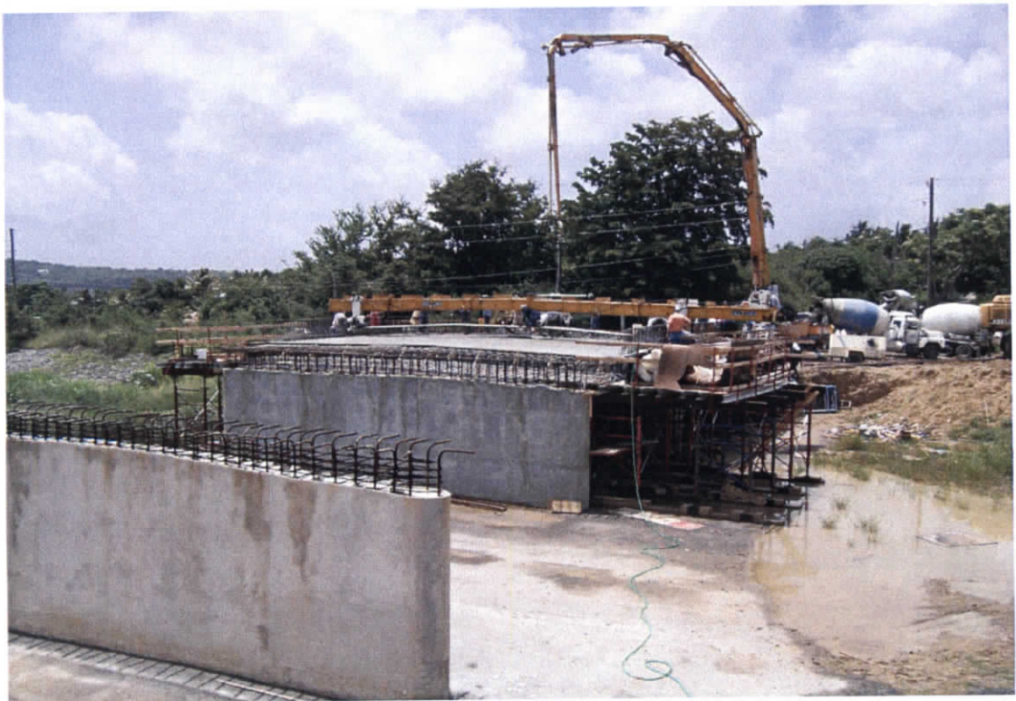
Hwy. 73 Bridge Deck Construction
