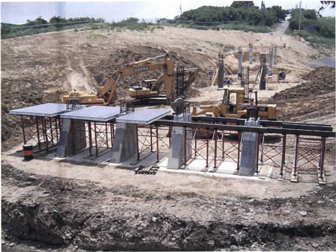
Glynn Rd. Bridge Abutment Construction
