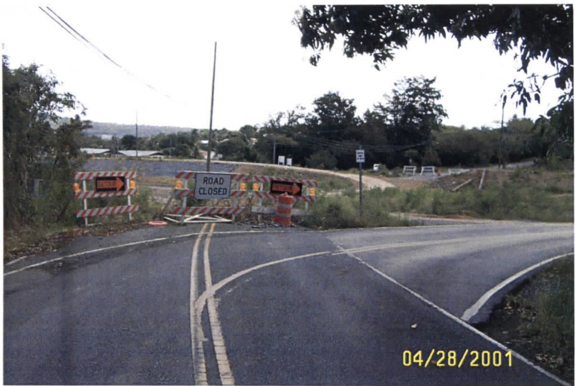
Hwy 73 Bridge before construction
