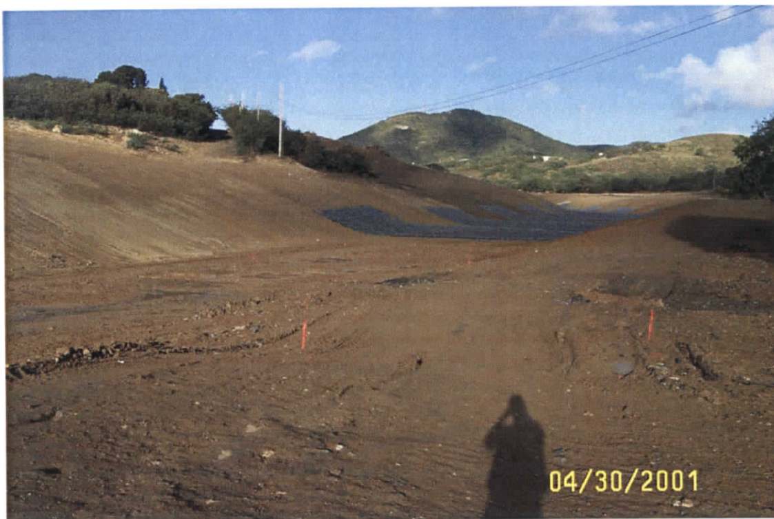
Glynn Rd. Bridge Location Before Construction
