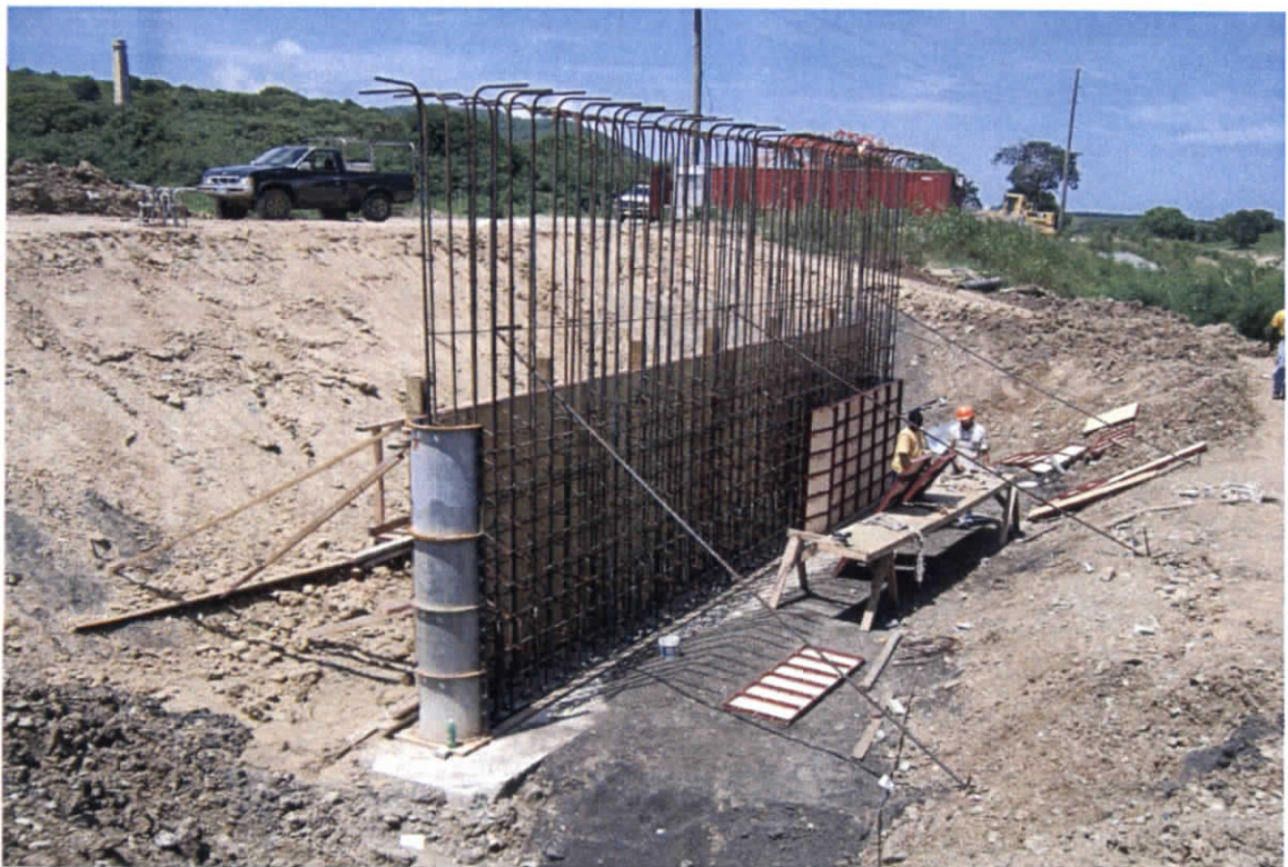
Hwy 73 bridge pier construction
