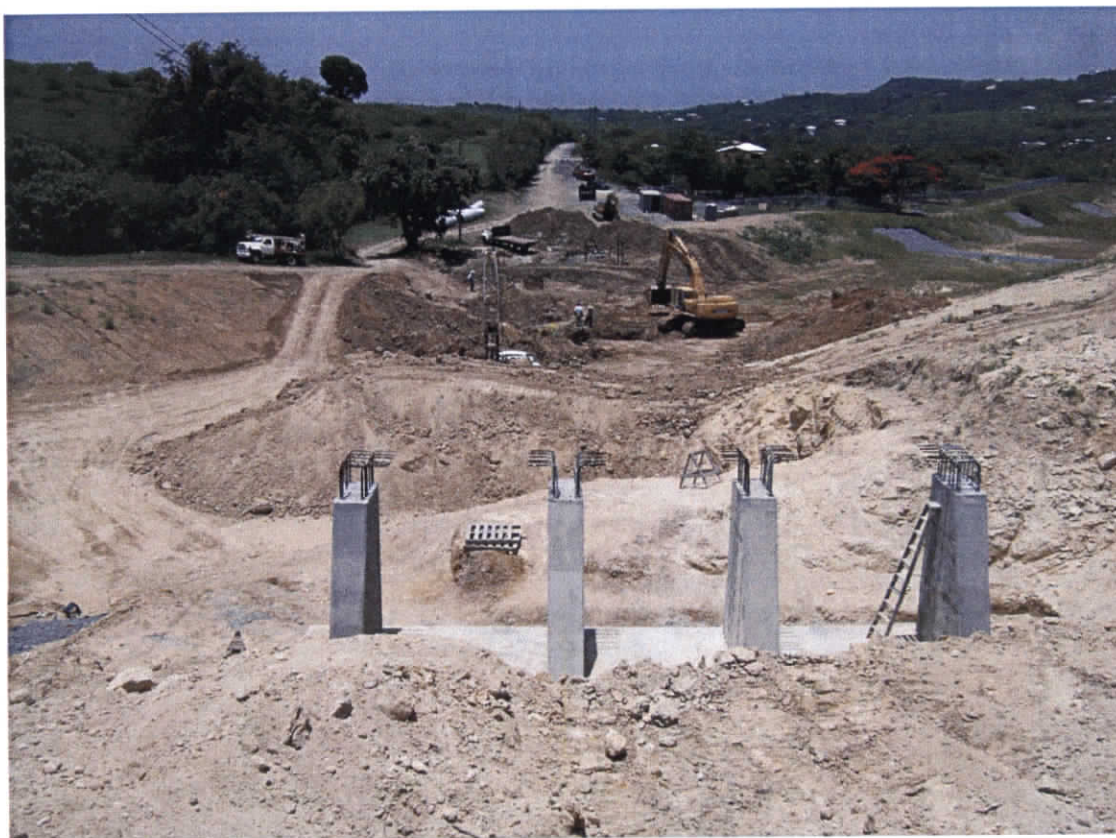
Glynn Rd. Bridge Constructing Abutment
