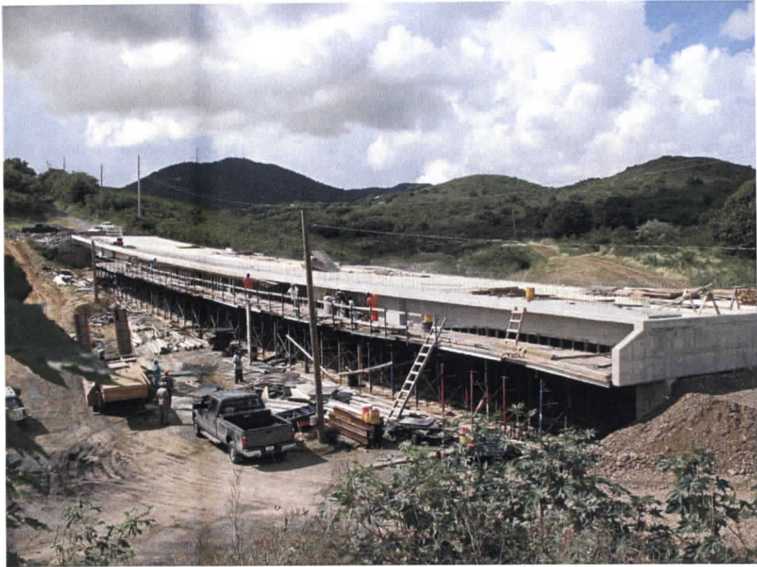
Glynn Rd. Bridge Deck Construction
