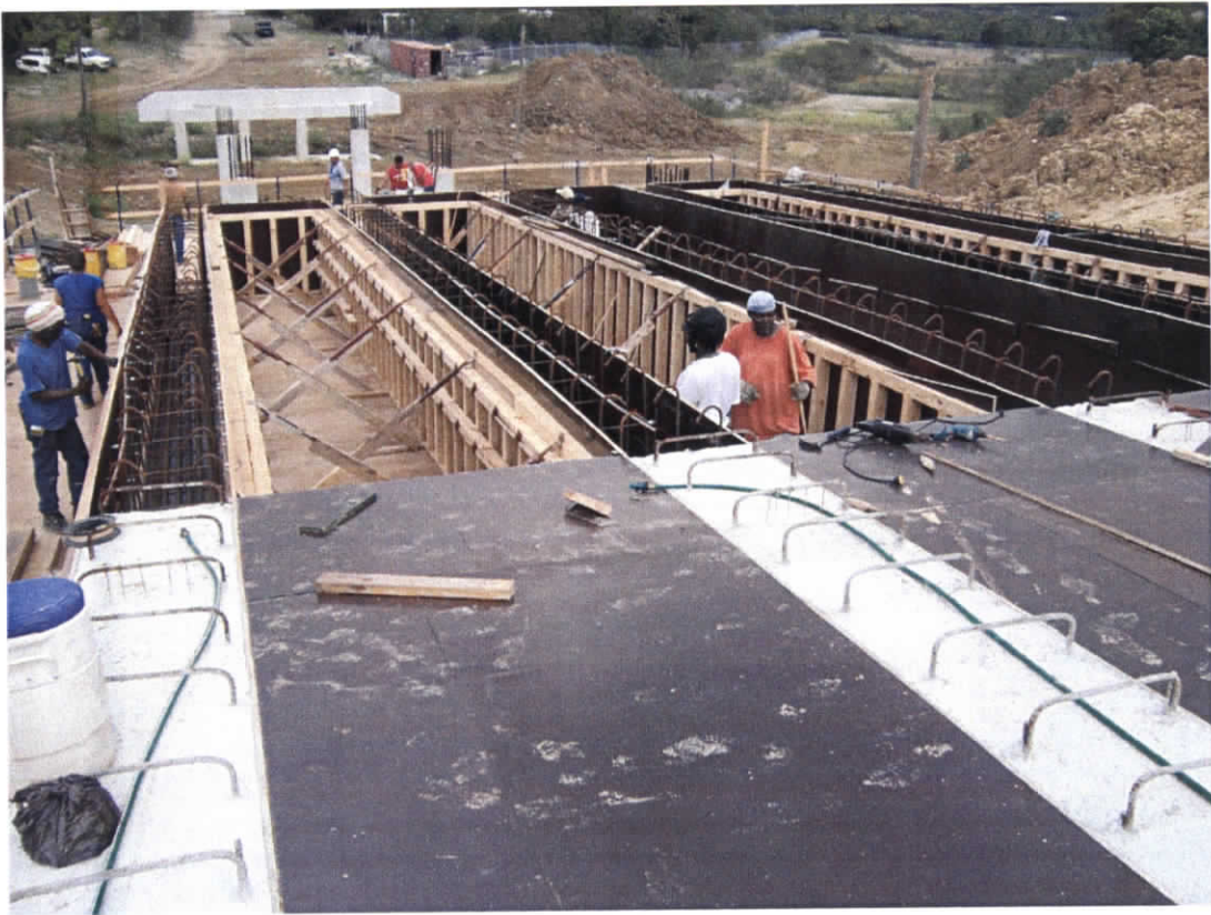
Glynn Rd. Bridge Deck Construction
