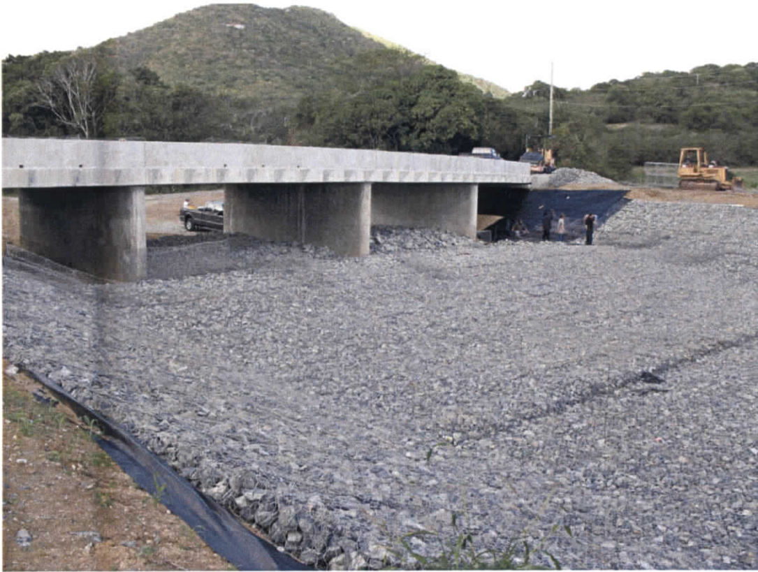
Hwy. 73 Bridge Placing Gabion Baskets
