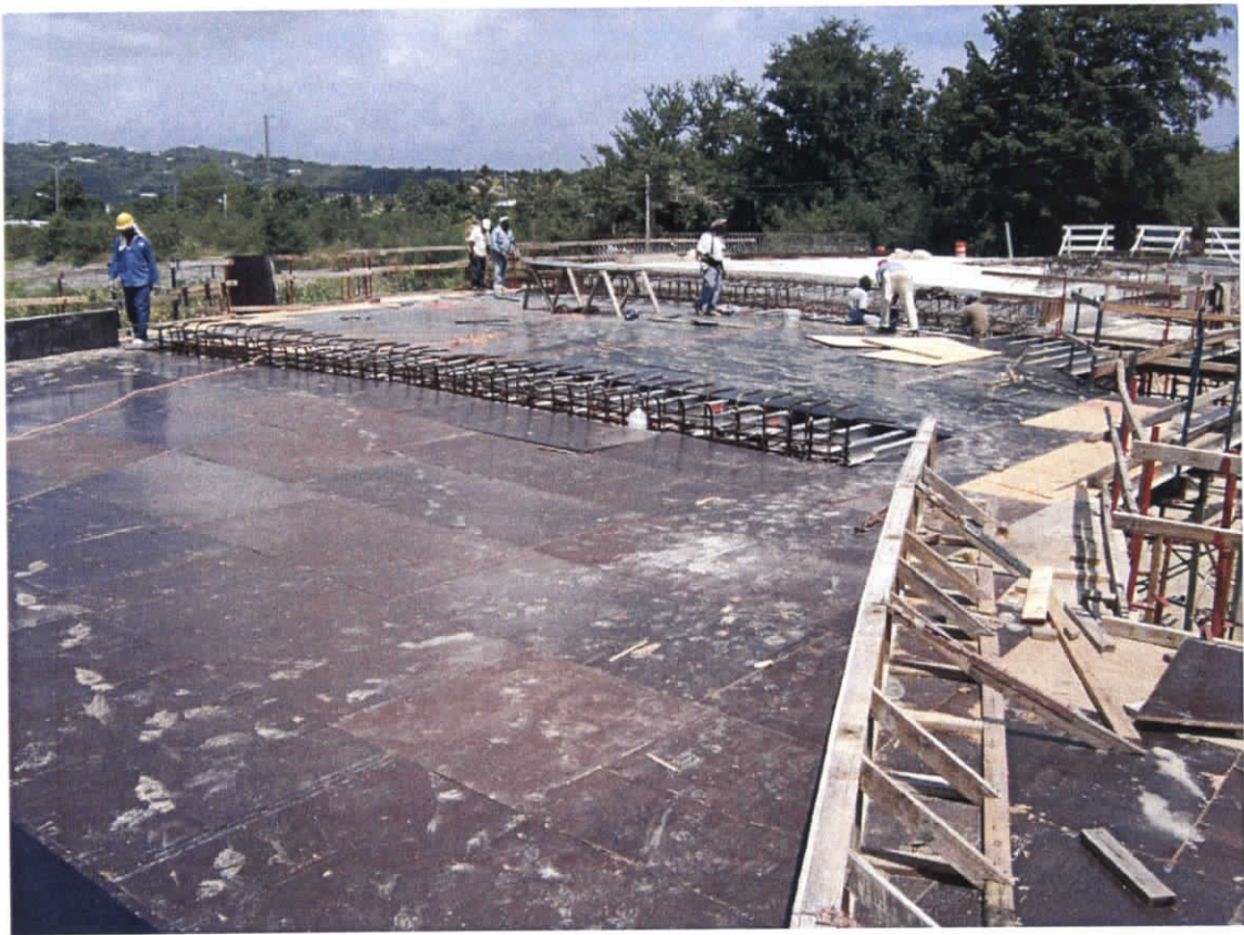
Hwy. 73 Bridge Deck Construction
