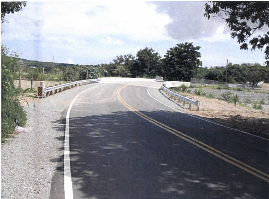
Hwy. 73 Bridge Completed Project
