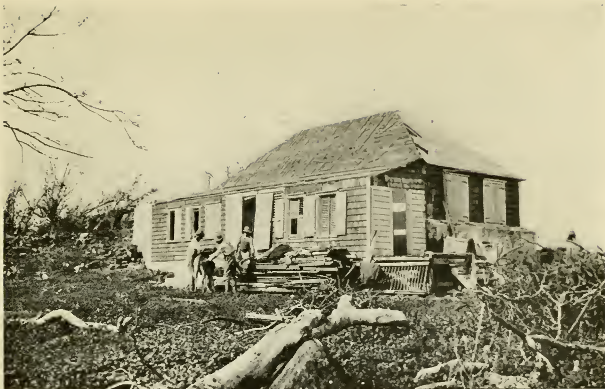
CANAAN ESTATE HOUSE, AFTER HURRICANE
