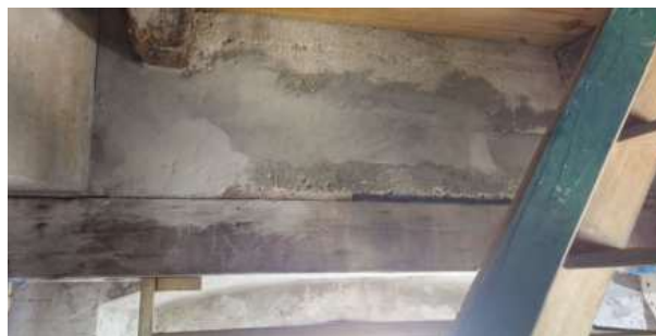
FIGURE 3-130. Concrete patch or repair on southwest wall of third tier.
