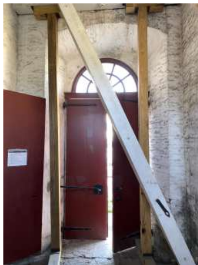
FIGURE 2-66. Photographs of temporary support beams installed at the western entrance door and north window in the steeple tower taken February 2022. Photograph by the author.
