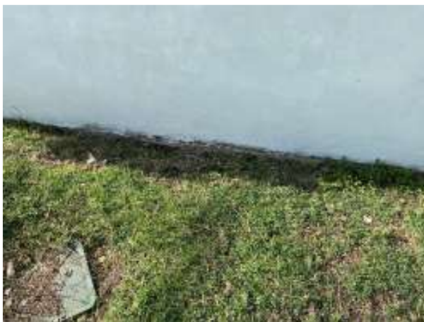
FIGURE 3-146. Close-up of the top of the foundation beneath the exterior masonry wall.
