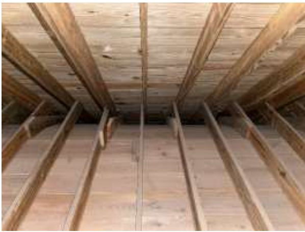
FIGURE 3-156. Roof framing over a one-story portion of Steeple Building.
