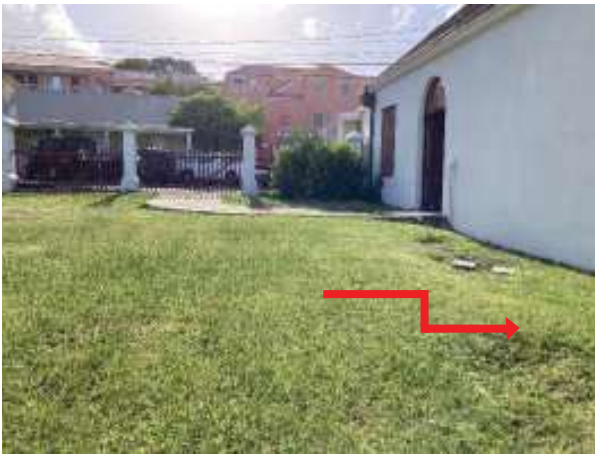
FIGURE 3-153. Site drainage toward the south wall.
