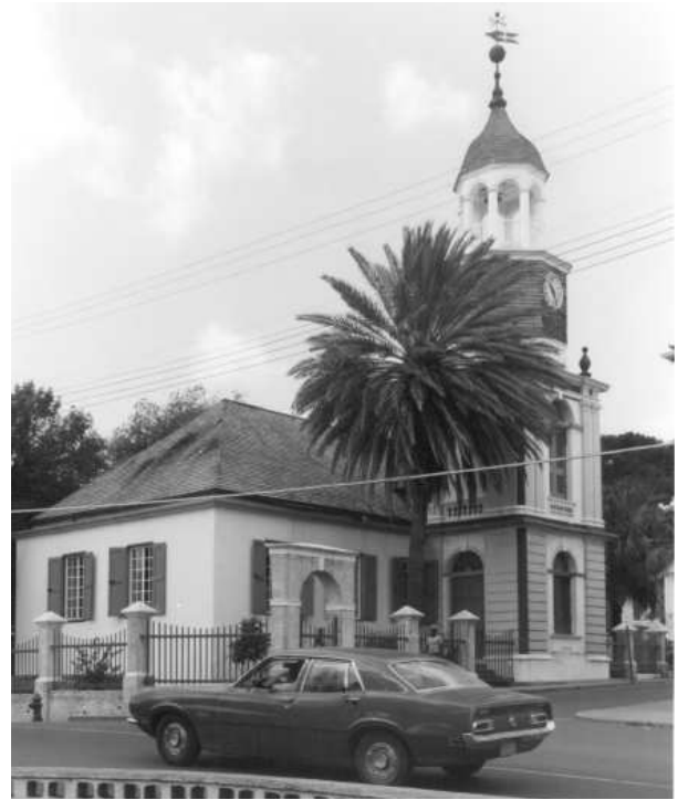
FIGURE 2–31. The northeast corner of the Steeple Building in 1976, as documented for the National Register Nomination Form. Photo: National Register of Historic Places Nomination Form for Christiansted National Historic Site, 1976.
