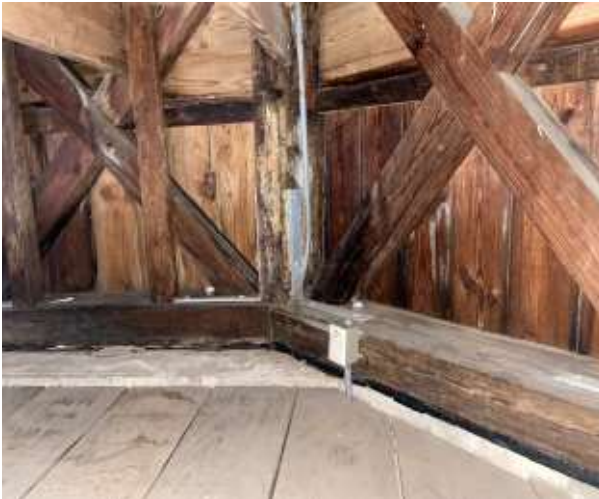
FIGURE 3-166. Retrofit wood cupola framing.
