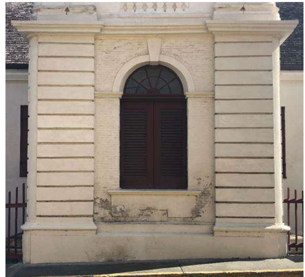
FIGURE 3-33. Northwest elevation, first tier.
