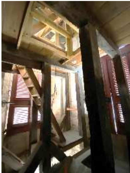
FIGURE 3-161. Internal wood framed ladder and landing.
