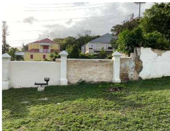
FIGURE 2–67. Photograph of the rear yard wall with repairs completed, as evident by the new bricks and stucco finish on portions of the wall at left and more weathered portions of the wall at right, taken February 2022. Photograph by the author.
