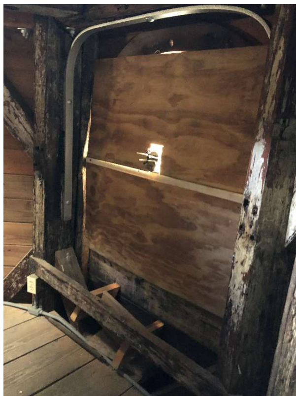
FIGURE 3-137. East wall of fourth tier.
