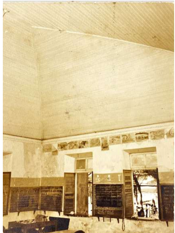
FIGURE 2-18. Interior of the Steeple Building in 1953 when used as a classroom, looking toward the east end windows. Photo: Frederik C. Gjessing, Condition Reports of Historic Buildings, 1953, photo 4.
