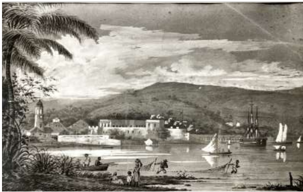
FIGURE 2–12. Christiansted, St. Croix, ca. 1845–1851 with Steeple Building visible at left. Note the east window in the second tier of the steeple is open in this painting; it was bricked up in 1851. Source: Lithograph by A. Nay from a painting by W. Melbye. From a copy in the Trade and Shipping Museum at Kronborg Castle, Elsinore, Denmark. From Herbert Olsen, Historic Structures Report , 1959, fig. 16.
