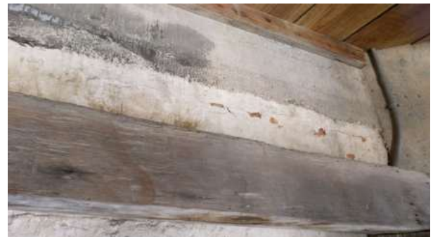
FIGURE 3-127. New concrete slab pour on southeast wall of third tier.
