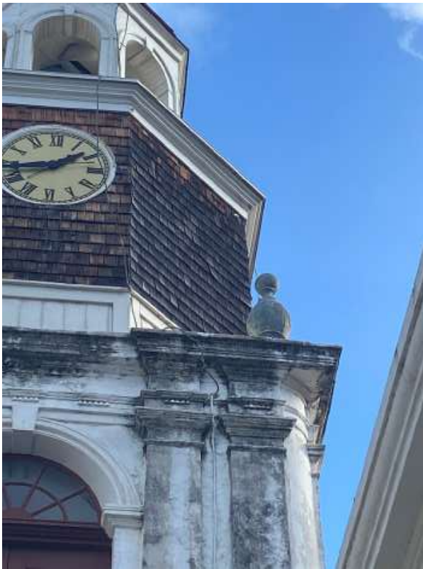
FIGURE 5-13. Finials at the top of the masonry pier
