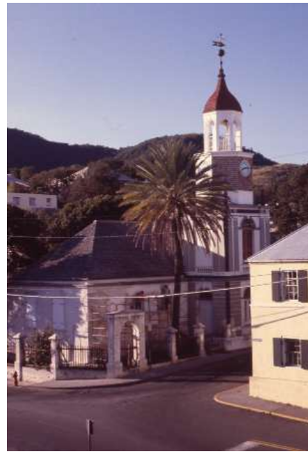
FIGURE 2–44. February 1986 photograph of Steeple Building prior to paint color change for steeple. Photo: Christiansted National Historic Site Archives.
