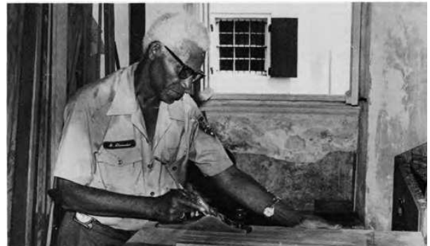
FIGURE 2-43. Master carpenter Joseph Alexander hand planing shutter frame for Steeple Building. Source: Barta, “Christiansted National Historic Site.”
