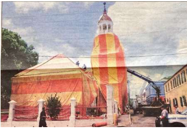
FIGURE 2-61. Newspaper photograph of the Steeple Building under a fumigation tent during treatment for termites in 2010. Photo: Cristian Simescu, "Under the big top," The Virgin Islands Daily News , No. 21828, August 3, 2010.
