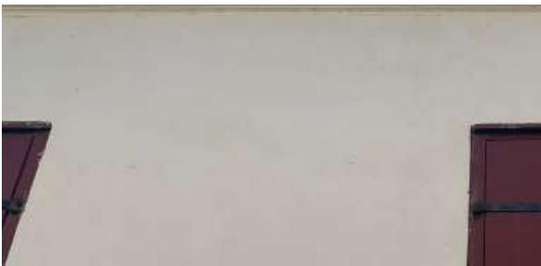
FIGURE 3-14. Cracking between Windows 5 and 6.
