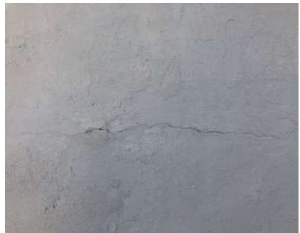
FIGURE 5-1. Exterior crack.
