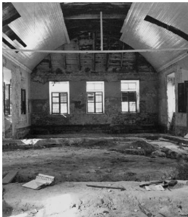
FIGURE 3-148. A transverse foundation wall documented below the existing floor in the HABS documentation.
