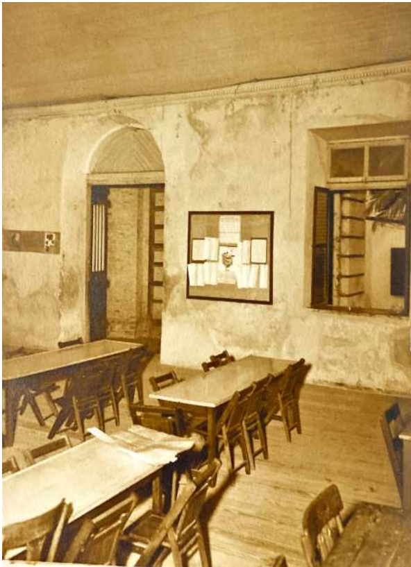
FIGURE 2-17. Interior of the Steeple Building in 1953 when used as a classroom, looking towards the door between the tower and the main building. Photo: Frederik C. Gjessing, Condition Reports of Historic Buildings, 1953, photo 3.
