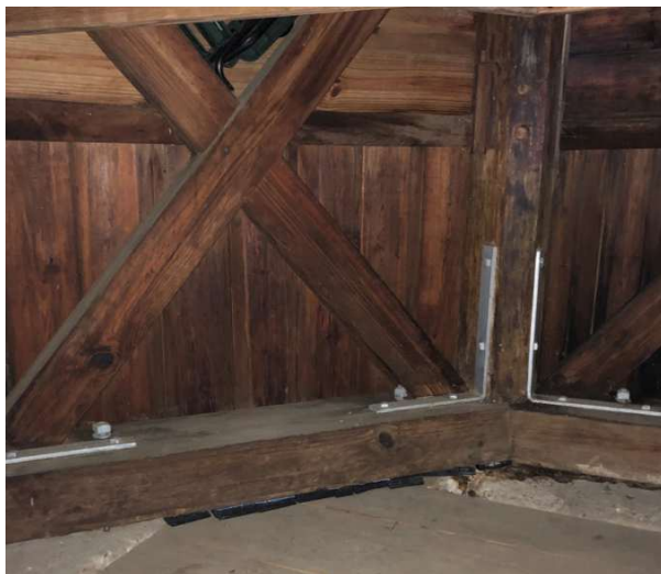
FIGURE 3-136. East wall of fourth tier.
