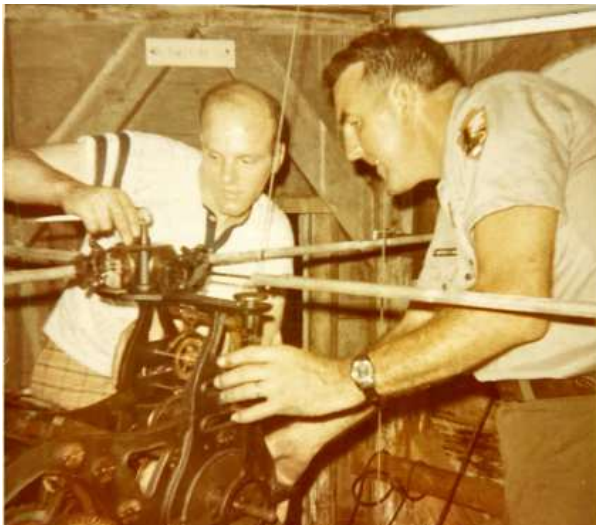
FIGURE 2–33. 1970 inspection of Steeple Building clock by National Park Service staff. Photo: Christiansted National Historic Site Archives.
