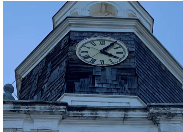
FIGURE 3-38. Northeast elevation, third tier.
