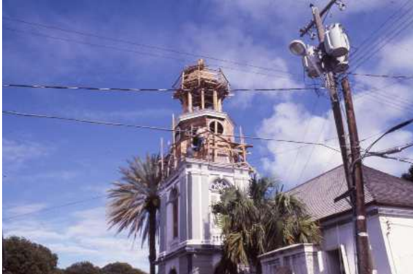
FIGURE 2-41. 1985 photo showing cupola reconstruction project in progress. Photo: Christiansted National Historic Site Archives.
