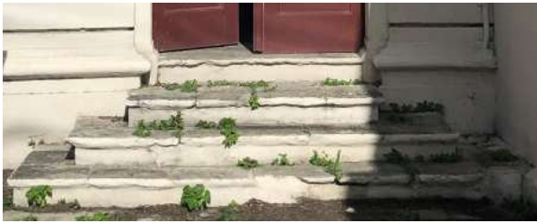
FIGURE 3–40. Steps to Door B on southwest elevation.
