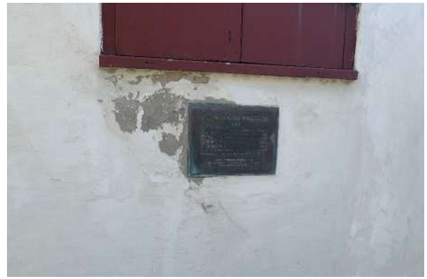
FIGURE 3-5. Plaster damage.
