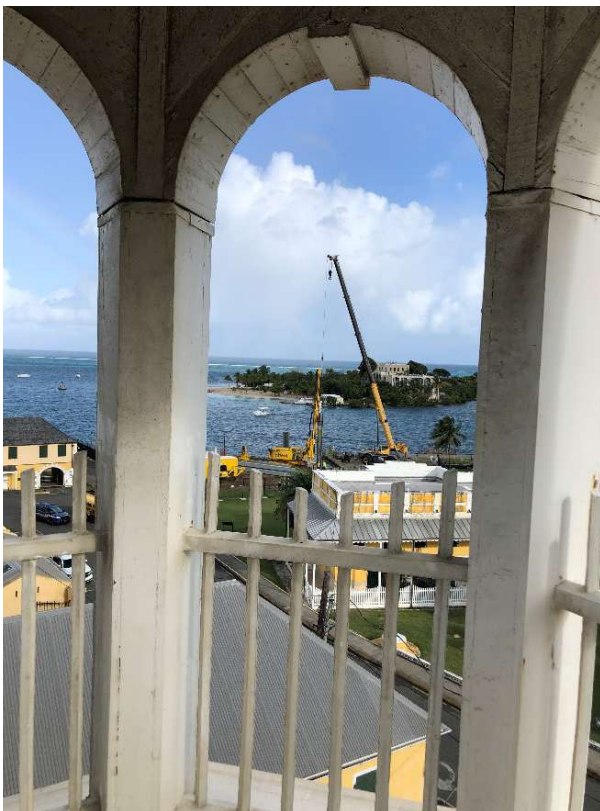
FIGURE 3-142. Columns, railing, and arch of cupola facing north.
