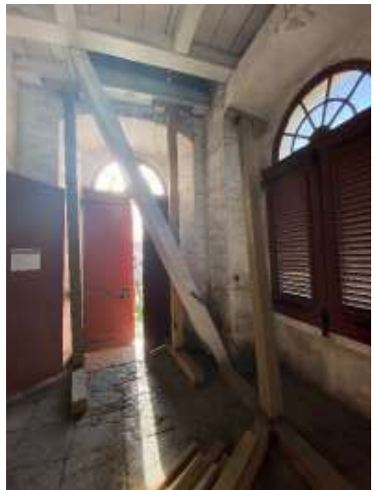
FIGURE 3-160. Temporary shoring placed at ground floor.
