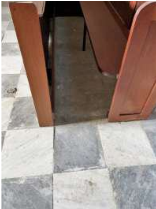
FIGURE 3-149. Close-up of tile and brick paver transition at the pew locations.
