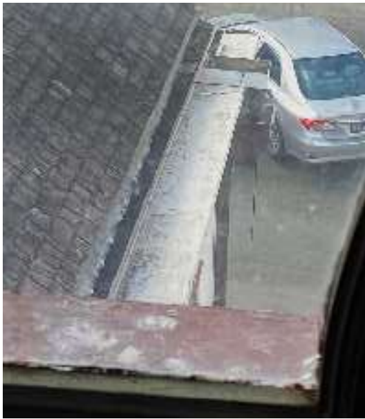
FIGURE 3-170. Gutter at existing Steeple Building.
