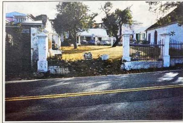
Steeple Building Fence showing Hurricane Hugo damage
