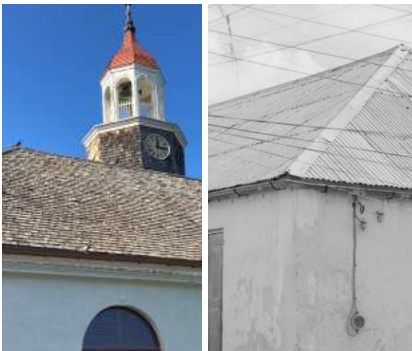
FIGURE 3-157. Wood shingles (today) vs. corrugated metal roof (1950s).
