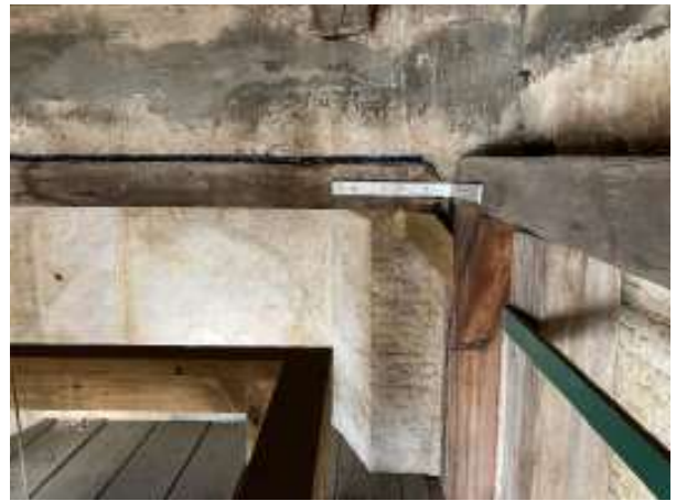
FIGURE 3-159. Concrete bond beam between second and third tier in the steeple.
