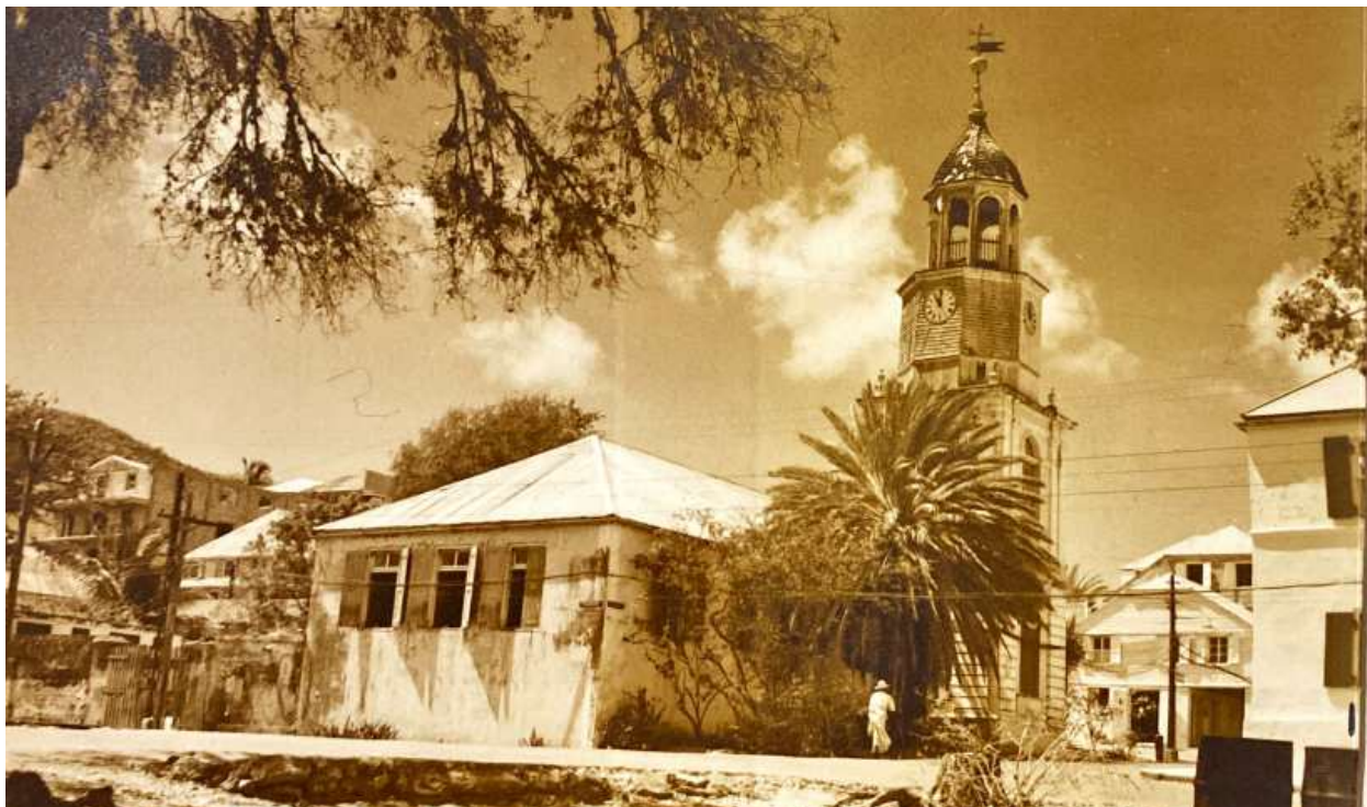
FIGURE 2-19. North corner of the Steeple Building and wall around rear yard in 1953. Photo: Frederik C. Gjessing, Condition Reports of Historic Buildings, 1953, photo 2.
