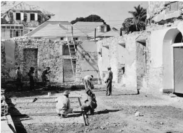
FIGURE 3-168. Historic photo showing when two walls were removed and rebuilt.
