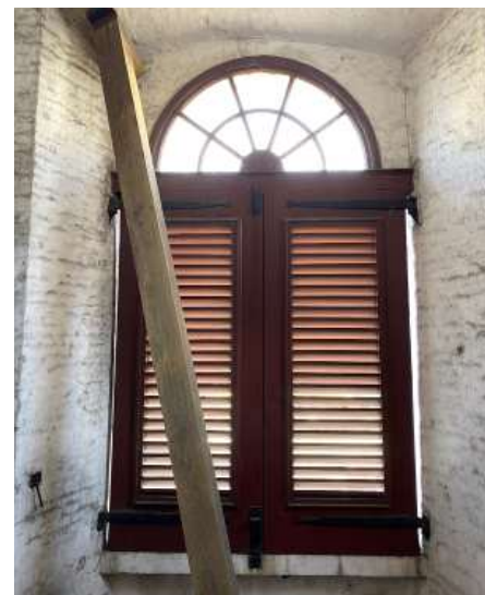
FIGURE 2-66. Photographs of temporary support beams installed at the western entrance door and north window in the steeple tower taken February 2022. Photograph by the author.
