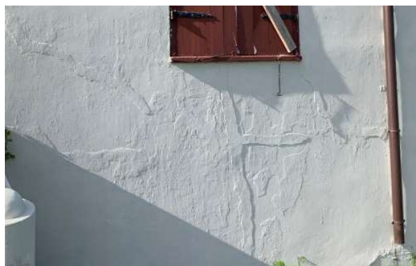
FIGURE 3-29. Series of patches under Window 9.
