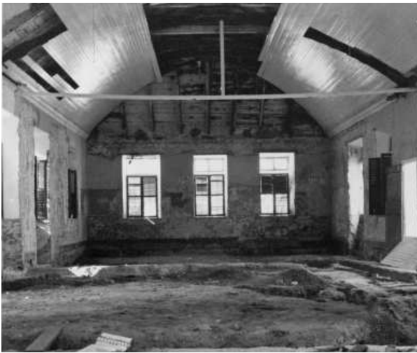
FIGURE 2–25. 1957 photo of the Steeple Building interior at the beginning of the demolition phase of the rehabilitation. Source: Historic American Buildings Survey No. VI-1.
