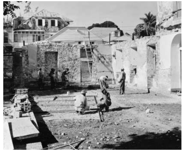
FIGURE 2–26. 1961 photo of the Steeple Building during the demolition phase of the rehabilitation. The roof, east end wall, and south wall had been removed. Note the bricked up window openings on the west end wall at center and a portion of the steeple tower visible at right. Source: Historic American Buildings Survey No. VI-1.
