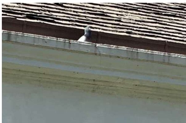
FIGURE 3-26. Crack in cornice near Door D.
