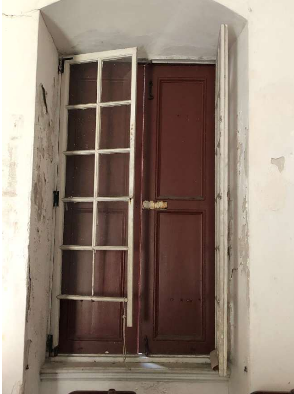
FIGURE 3-57. Plaster around Window 6.
