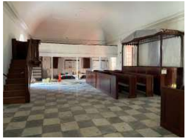
FIGURE 3-155. Wood-framed mezzanine at the west end of the interior.
