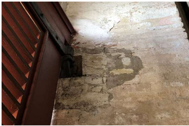
FIGURE 3-109. Repaired bracket on right side of window 14.
