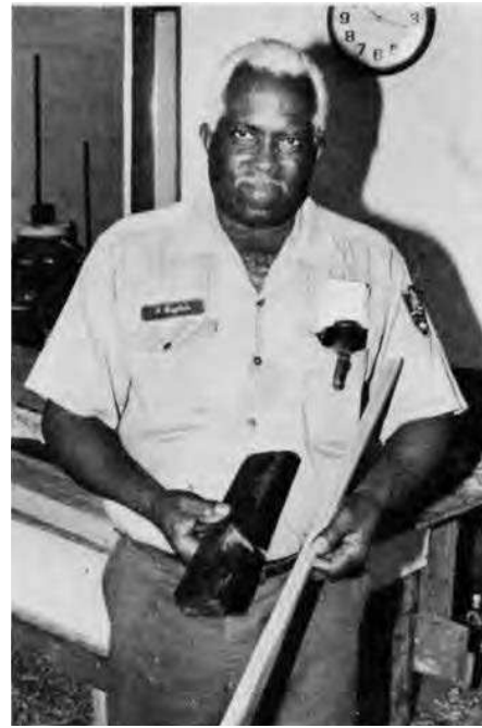
FIGURE 2-42. Maintenance supervisor Philbert Baptiste holding custom plane created to replicate original molding Steeple Building. Source: Barta, “Christiansted National Historic Site.”
