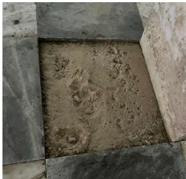
FIGURE 5-6. Floor tile setting bed.
