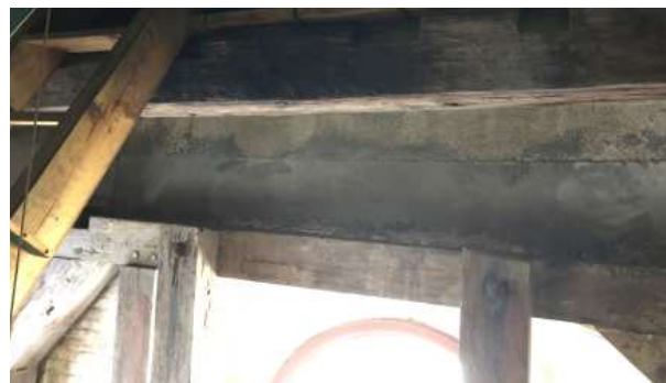
FIGURE 3-122. Concrete patch or repair on northwest wall of third tier.
