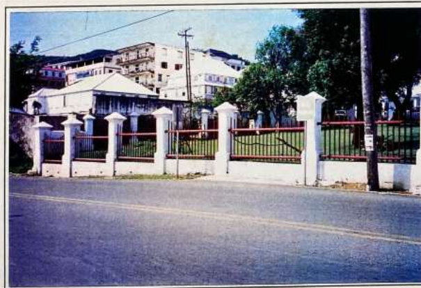
Steeple Building Fence following repairs by Field Services Unit
