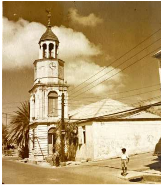
FIGURE 2–15. Figure 13. Tower and west corner of the Steeple Building in 1953 with hairline cracks visible in end wall. Photo: Frederik C. Gjessing, Condition Reports of Historic Buildings , 1953, photo 1.
