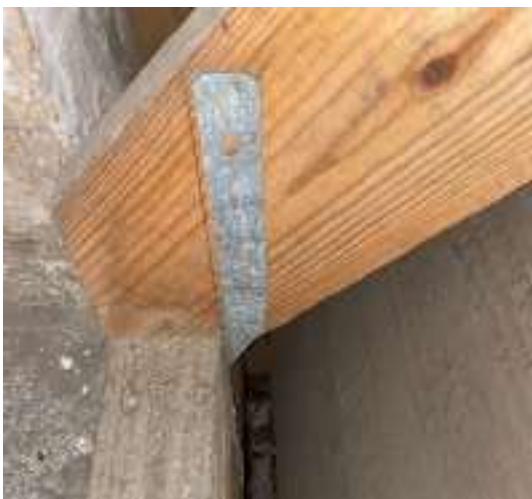
FIGURE 3-169. Metal strap at the roof rafter attachment to the masonry wall.
