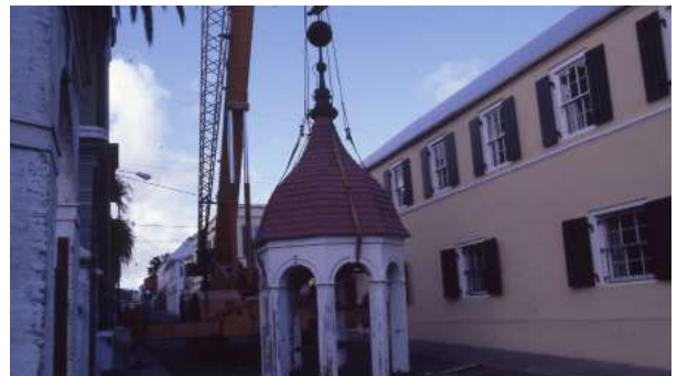
FIGURE 2-38. 1982 photograph of deteriorated cupola sitting on Company Street, having been removed from Steeple. Photo: Christiansted National Historic Site Archives.
