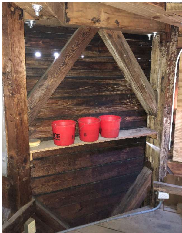
FIGURE 3-135. East wall of fourth tier.
