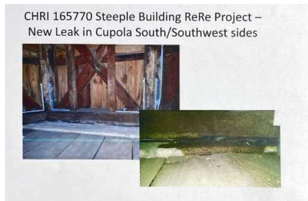
FIGURE 2-63. Photographs taken in 2017 by the National Park Service staff showing the location of a newly identified leak in the cupola. Source: National Park Service, Christiansted National Archives.
