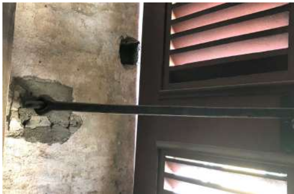
FIGURE 3-110. Repaired bracket on left side of window 14.
