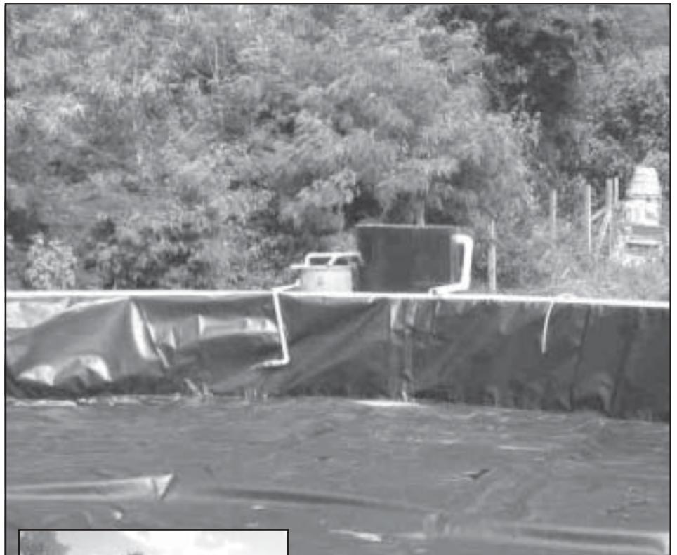
Top: The HDPE liner holds the water in the tank
