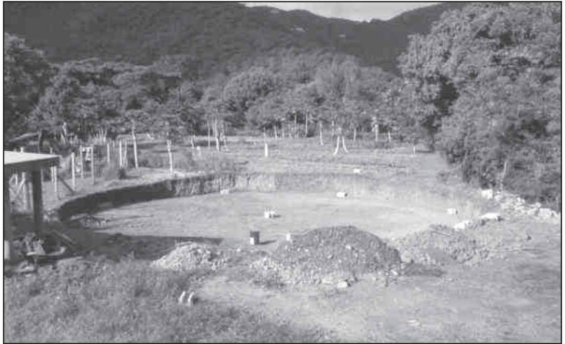
Above: The greenwater tanks site is adjacent to the existing vegetable gardens. The land was cleared and leveled before the block walls were constructed
