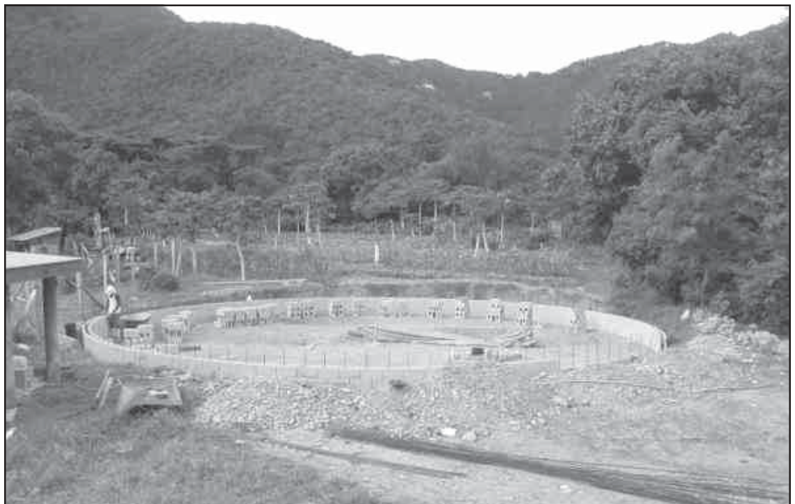
Below: The tiers of block were stacked to form the circular tank walls
