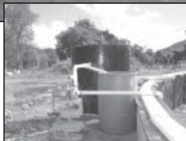
Top: The HDPE liner holds the water in the tank
