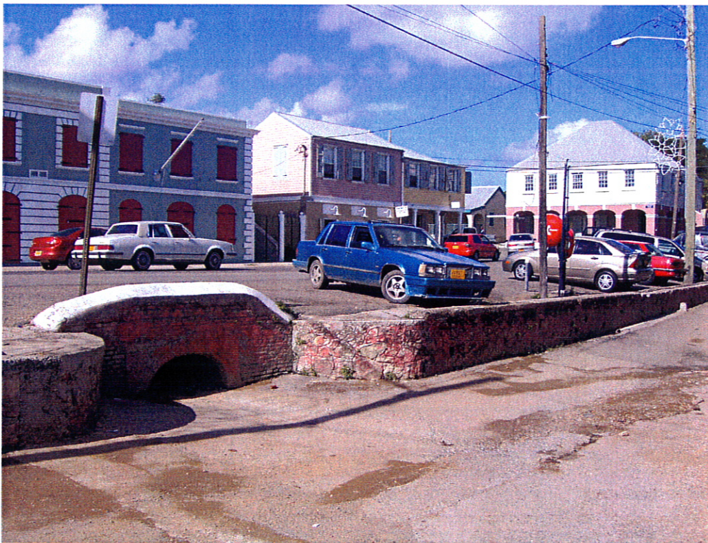
PICTURE 5: Before Construction – Market St., culvert outlet headwall (eastern)
