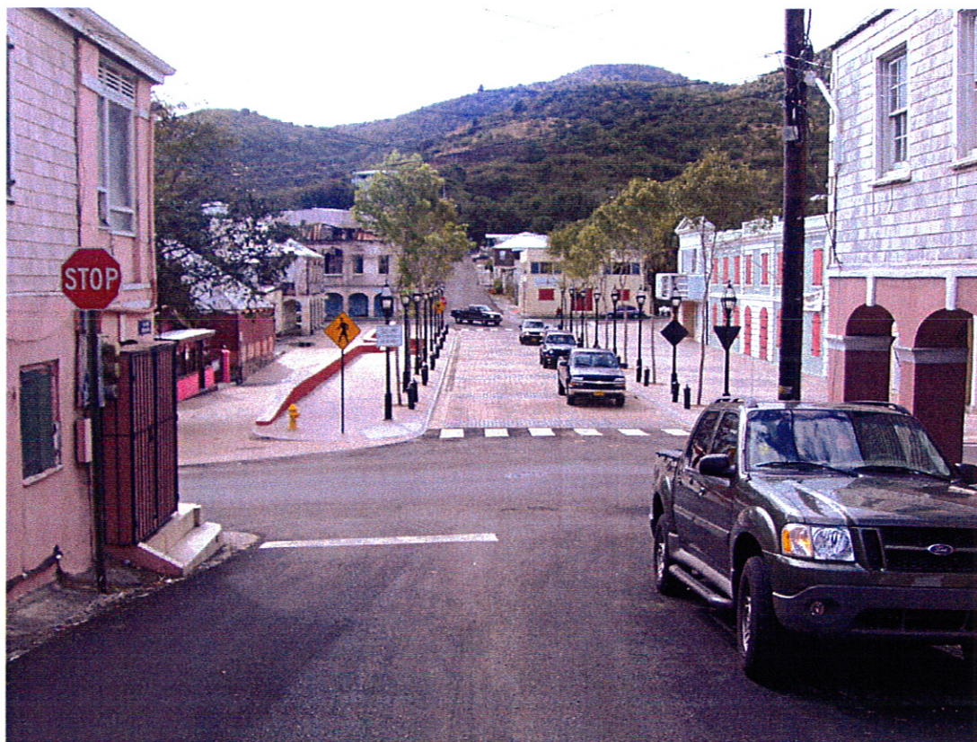
PICTURE 2: After Construction – No. Market Street looking south
