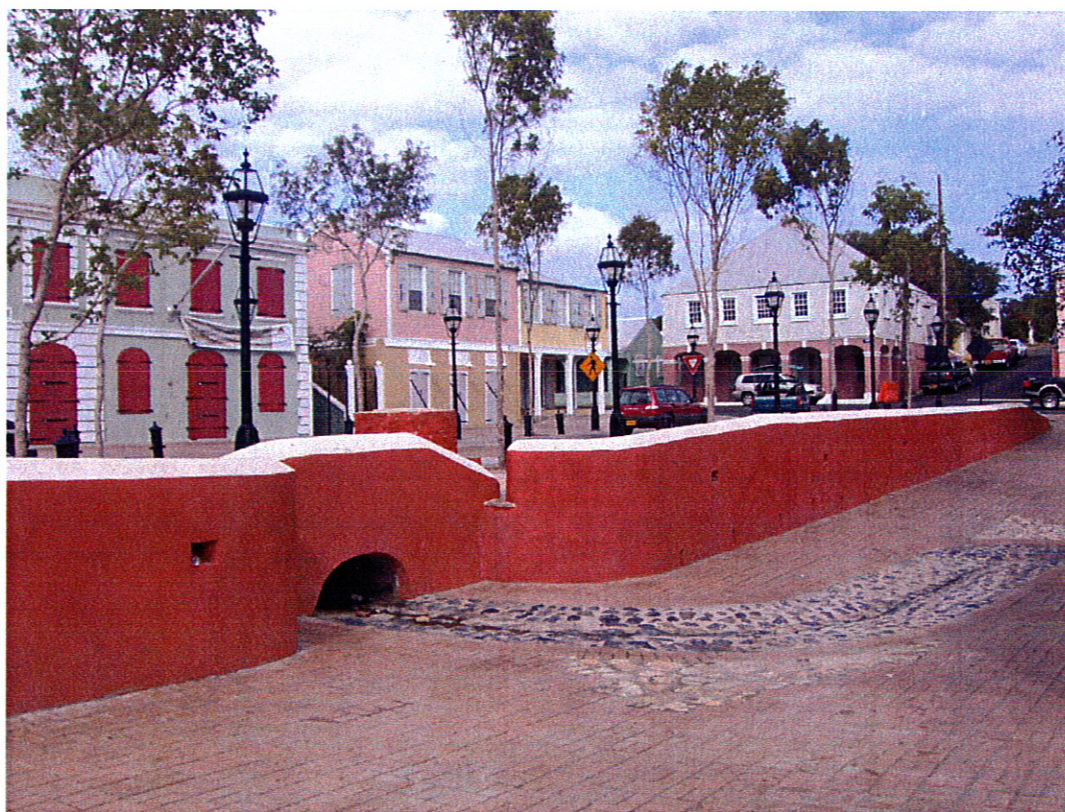
PICTURE 6: After Construction – Market St., culvert outlet headwall (eastern)
