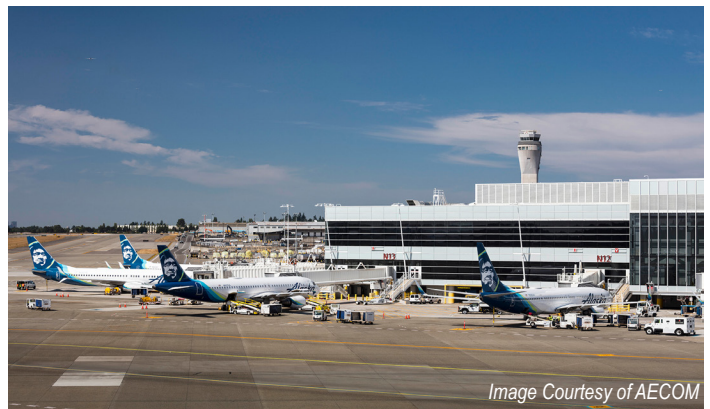
Seattle-Tacoma International Airport North Satellite
