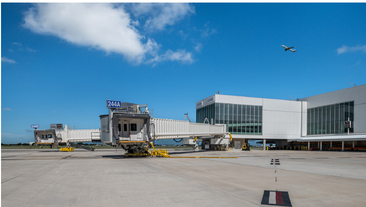
Orlando International Airport South Terminal C
