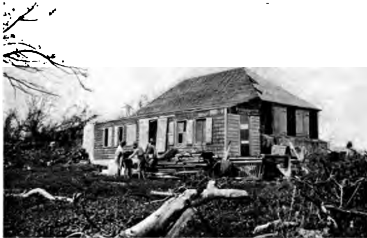
CANAAN ESTATE HOUSE, AFTER HURRICANE
