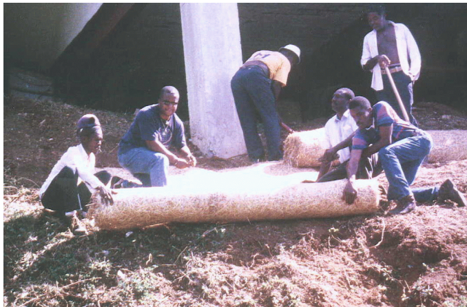
Installation of erosion & sediment control matting at Donoe Housing Community on St. Thomas.
