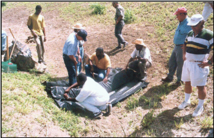
Figure 23. Erosion & Sediment Control Workshop trainees install a Triangular Silt Dike™ check dam in Estate St. George's Hill, St. Croix, June 1998.
