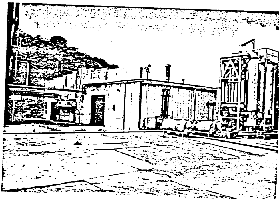
Photo #3. Maintenance building
