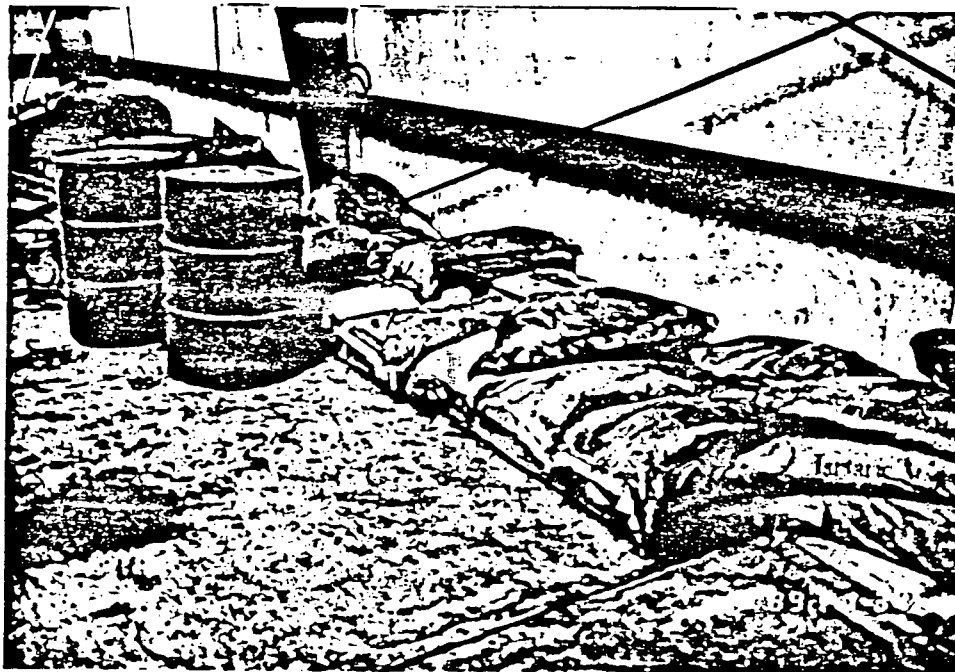
Photo #21. Deteriorating bags in area 6
