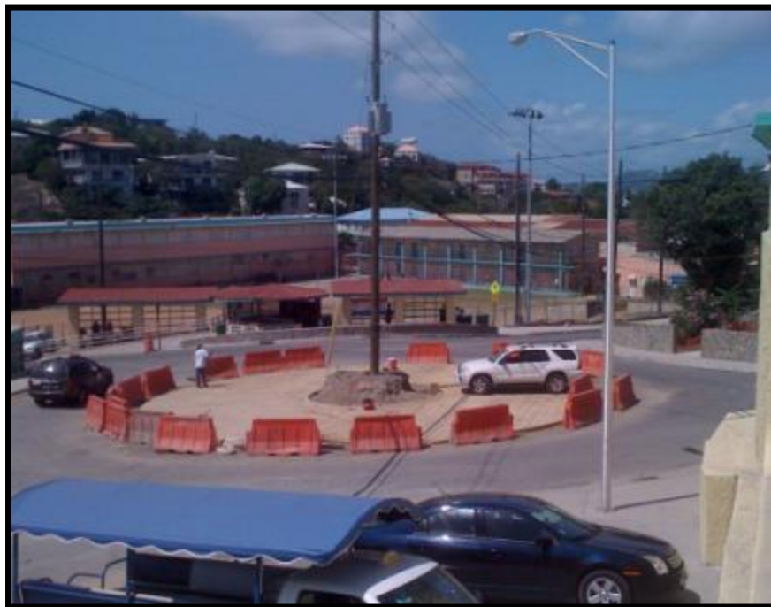
Constructed roundabout with stamped concrete
