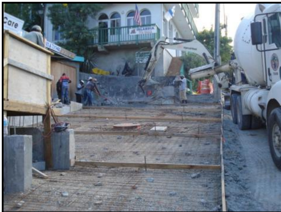
Route 10 East/Centerline Road – Boulon Parking construction
