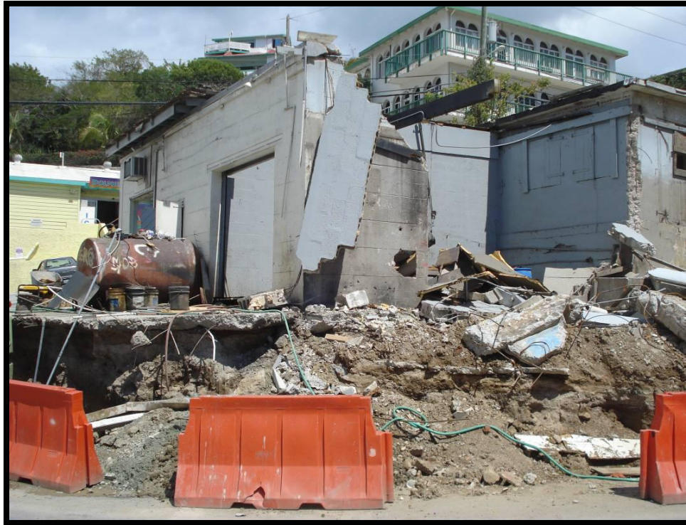
Gas Station building demolition works; view from Road 104/Southside road
