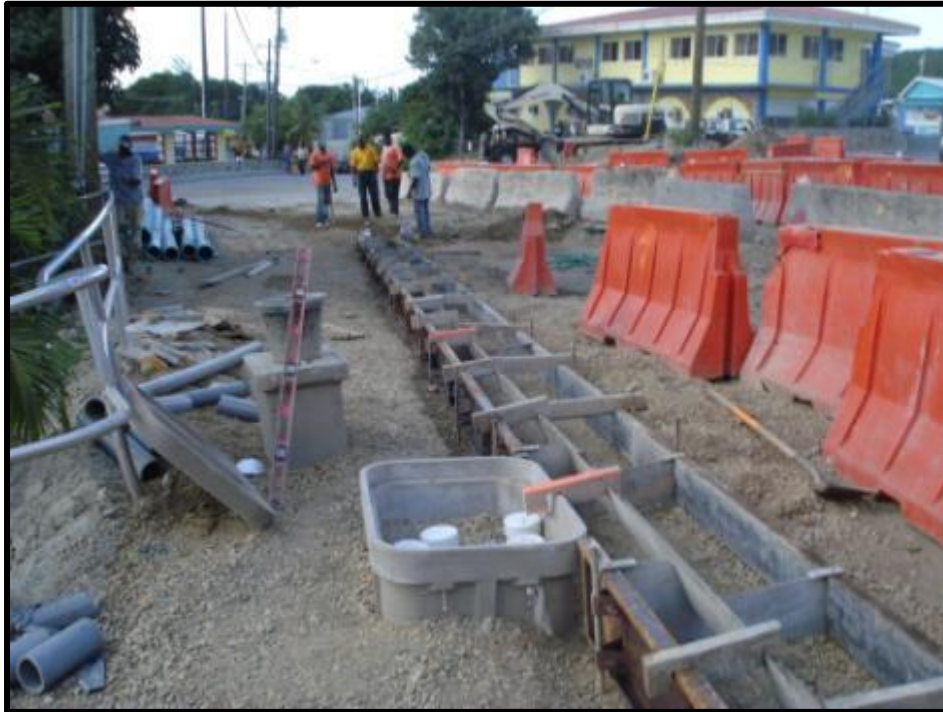
Route 104/ Southside Road curbs and gutter construction
