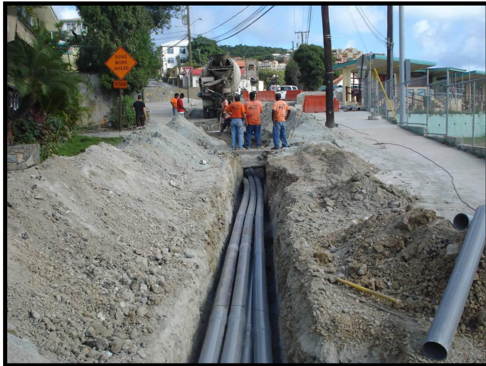
Electric conduit installation at Centerline Road/Route 10 West
