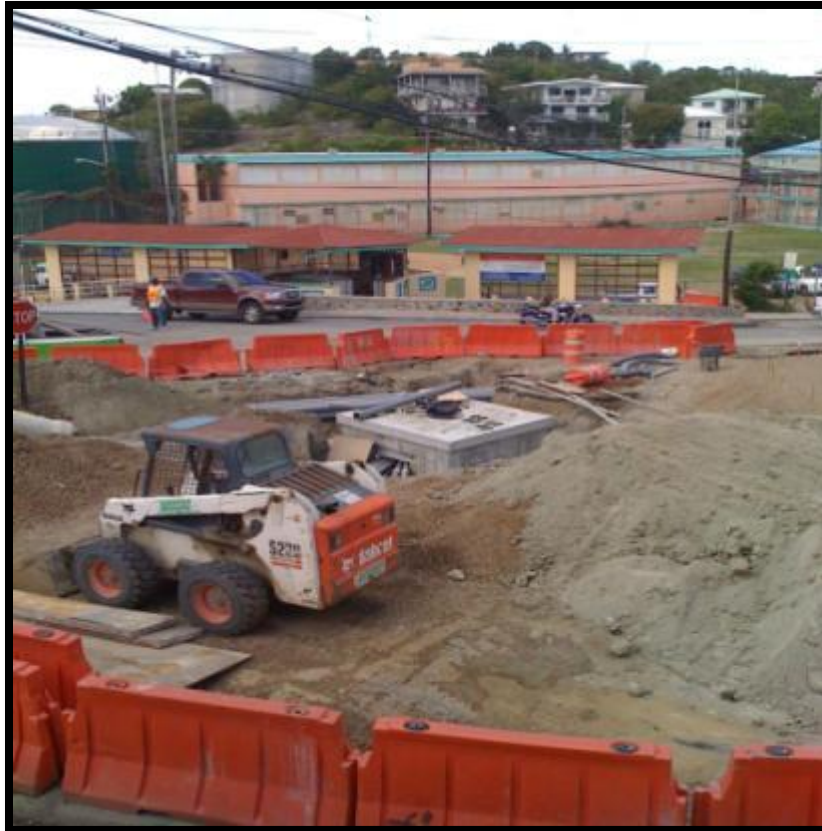
Roundabout area – electrical manhole and conduit installation
