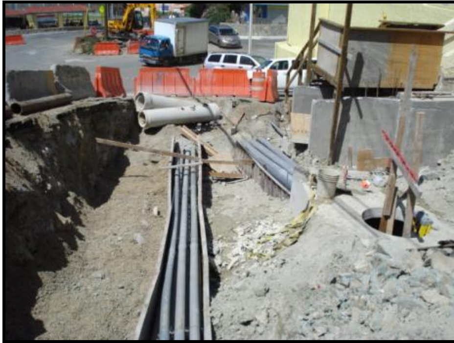
Route 10 East/Centerline Road – utilities infrastructure construction
