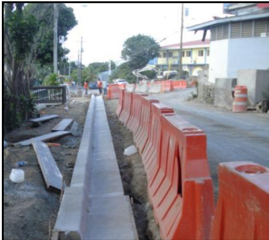
Route 104/Southside Road curbs and gutter construction
