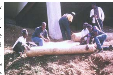
CES & VIHA staff install erosion control mats at Donoe Housing Community.
