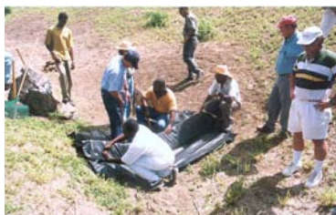
Installation of triangular dike check dam, Estate St. George's Hill, St. Croix.
