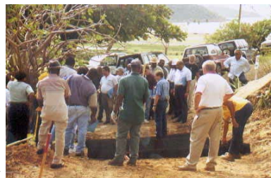
Workshop attendees learn how to install GeoWeb®.
