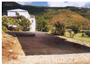
GeoBlock® with gravel entrance, prior to being filled with soil.
