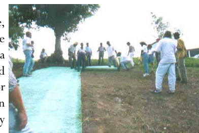
Workshop participants install excelsior erosion control mat on St. Croix.
