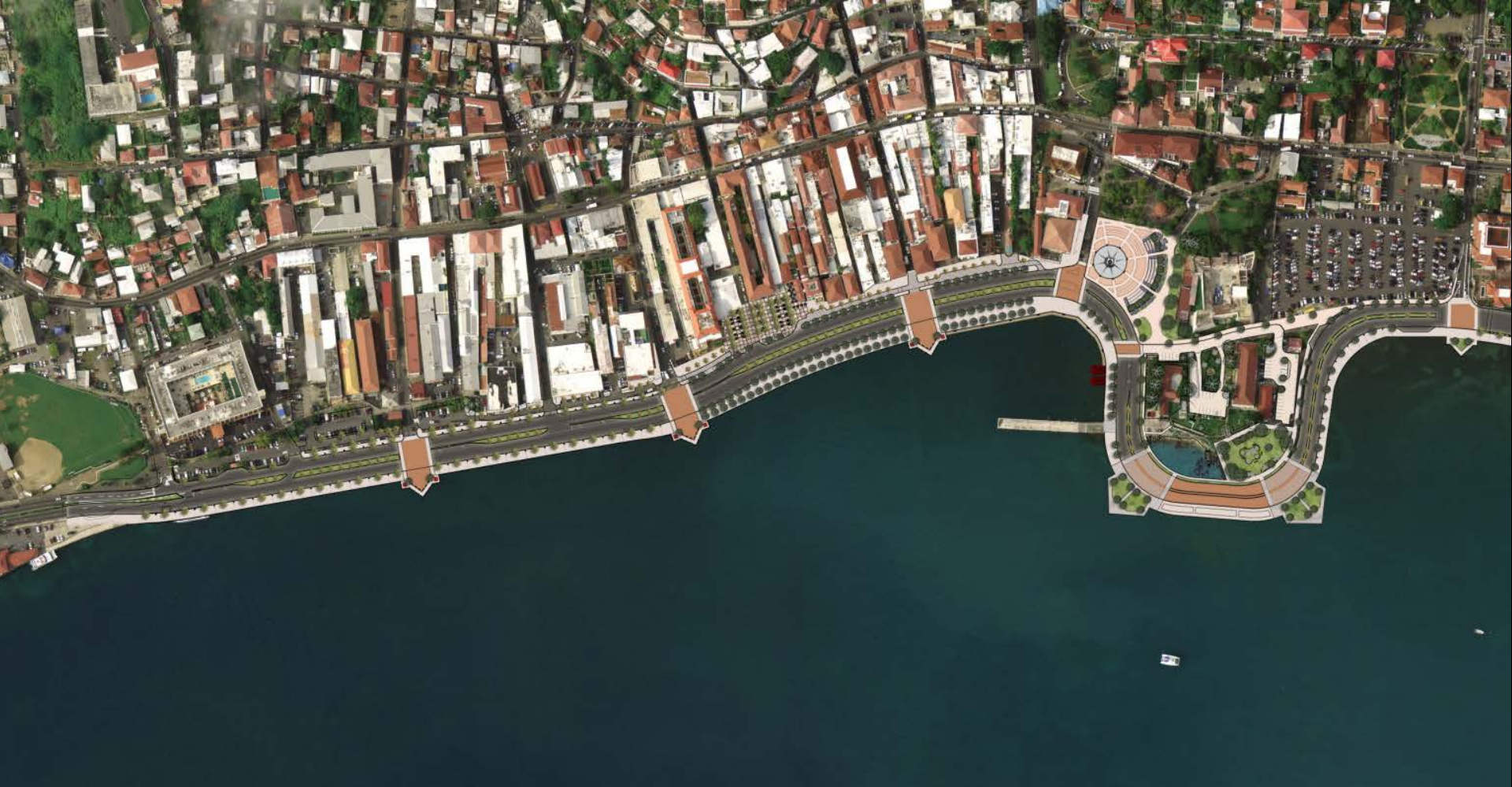
Veterans Drive – Phase 2 (Hospital Gade to Windward Passage Hotel)
