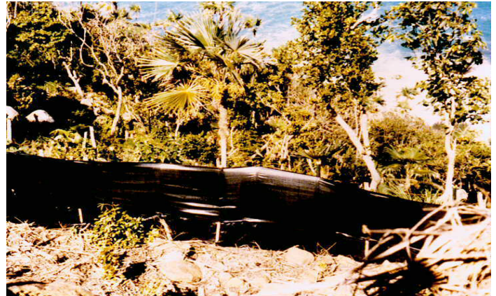
Wire mesh reinforced silt fence with steel posts installed prior to clearing along the downhill side of Caret Bay Villas site.
