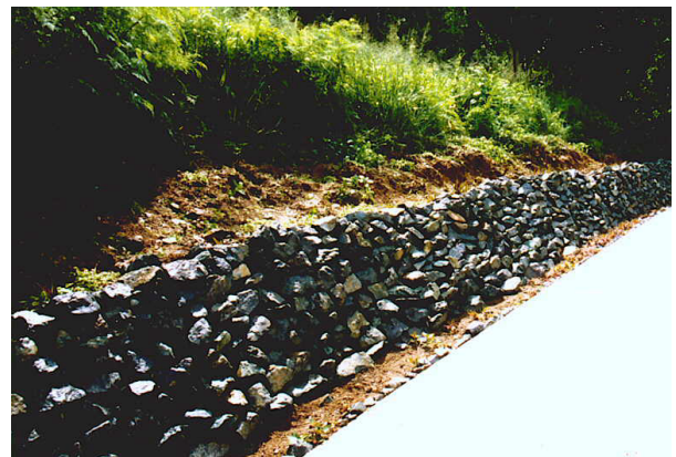
Stone terrace built to retain soil on driveway cut in Fortuna, St. Thomas.
