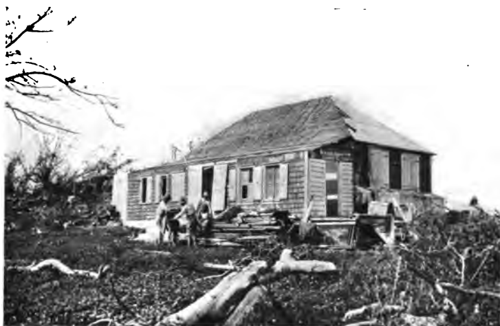
CANAAN ESTATE HOUSE, AFTER HURRICANE
