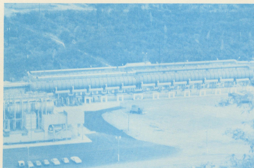
FIGURE 5b. Seawater flash vaporization desalination plant at Krum Bay (Sub Base).
