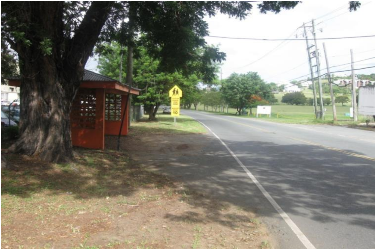
BUS SHELTER PRIOR TO REMOVAL
