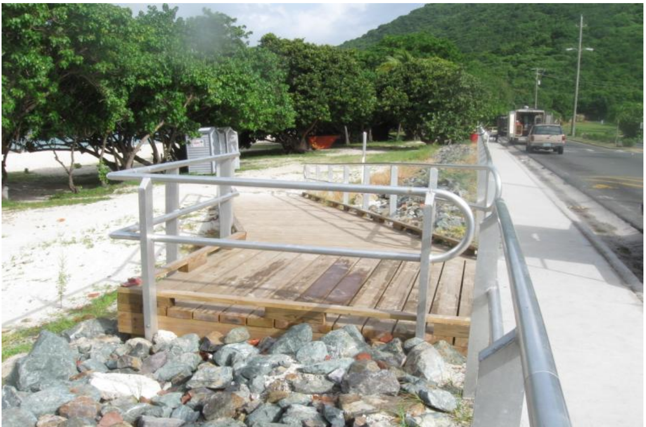
ACCESS TO BREWER'S BEACH AFTER INSTALLATION OF ACCESSIBILITY RAMP
