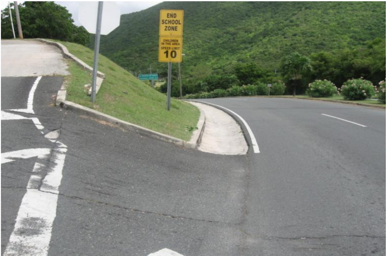
STATION 689+91 PRIOR TO SIDEWALK AND ROCKERY WALL INSTALLATION
