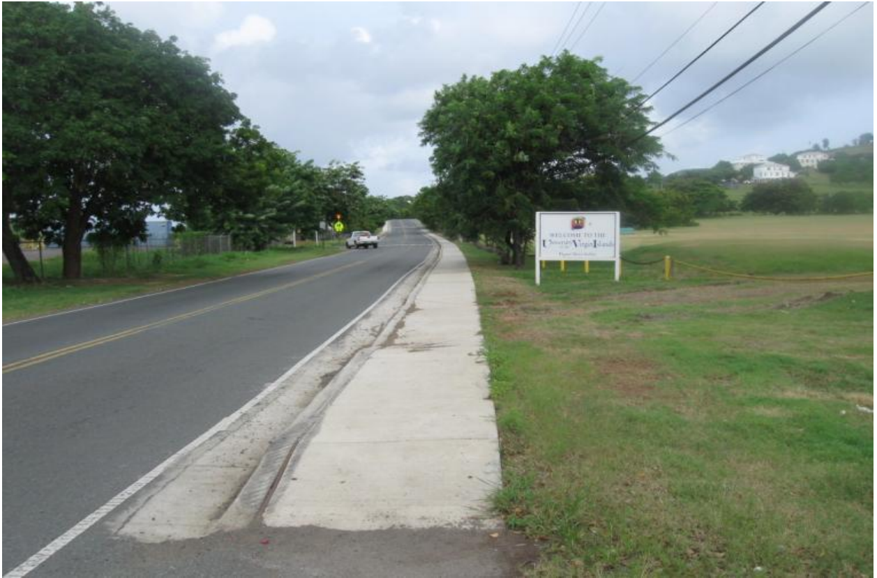
JULIAN JACKSON DRIVE AFTER SIDEWALK INSTALLATION
