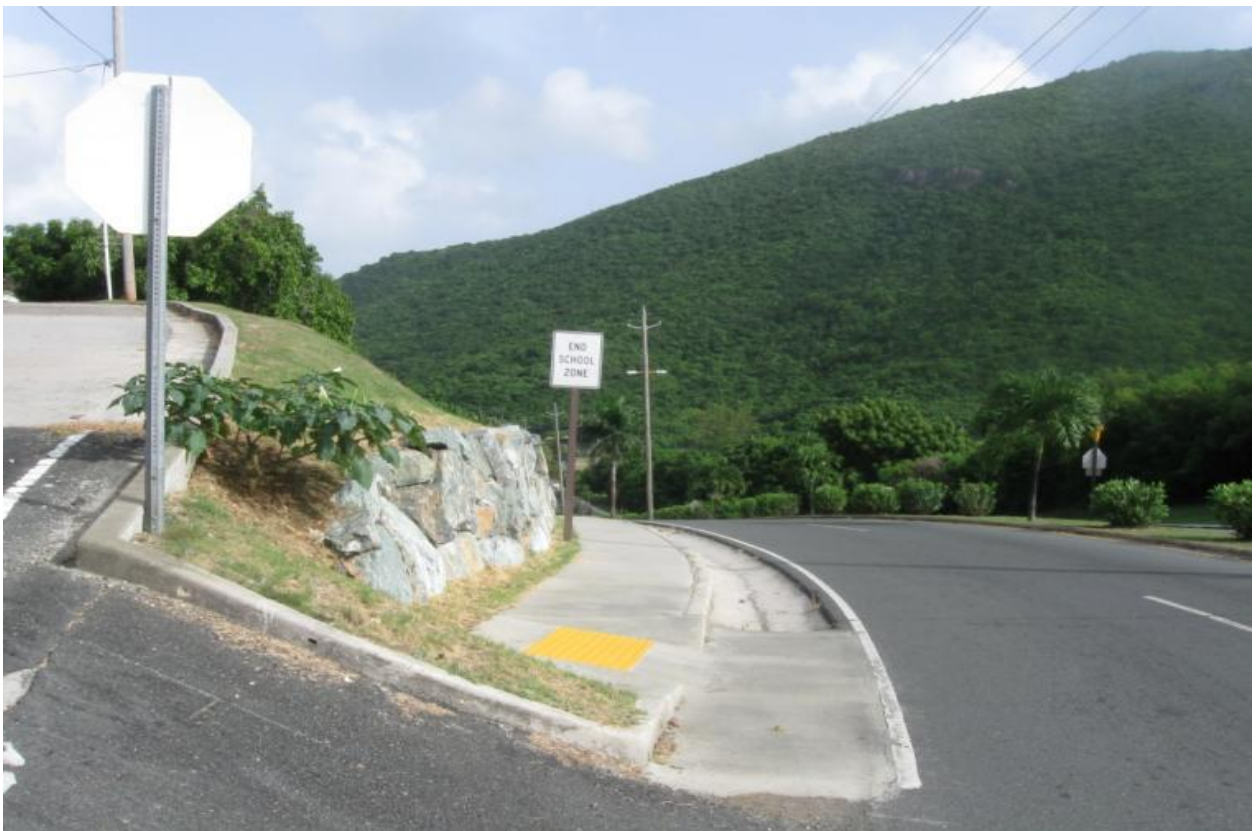
STATION 689+91 AFTER SIDEWALK AND ROCKERY WALL INSTALLATION
