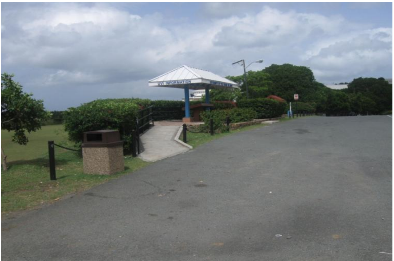
BUS PULL-OFF PRIOR TO SIDEWALK AND BOLLARD INSTALLATION
