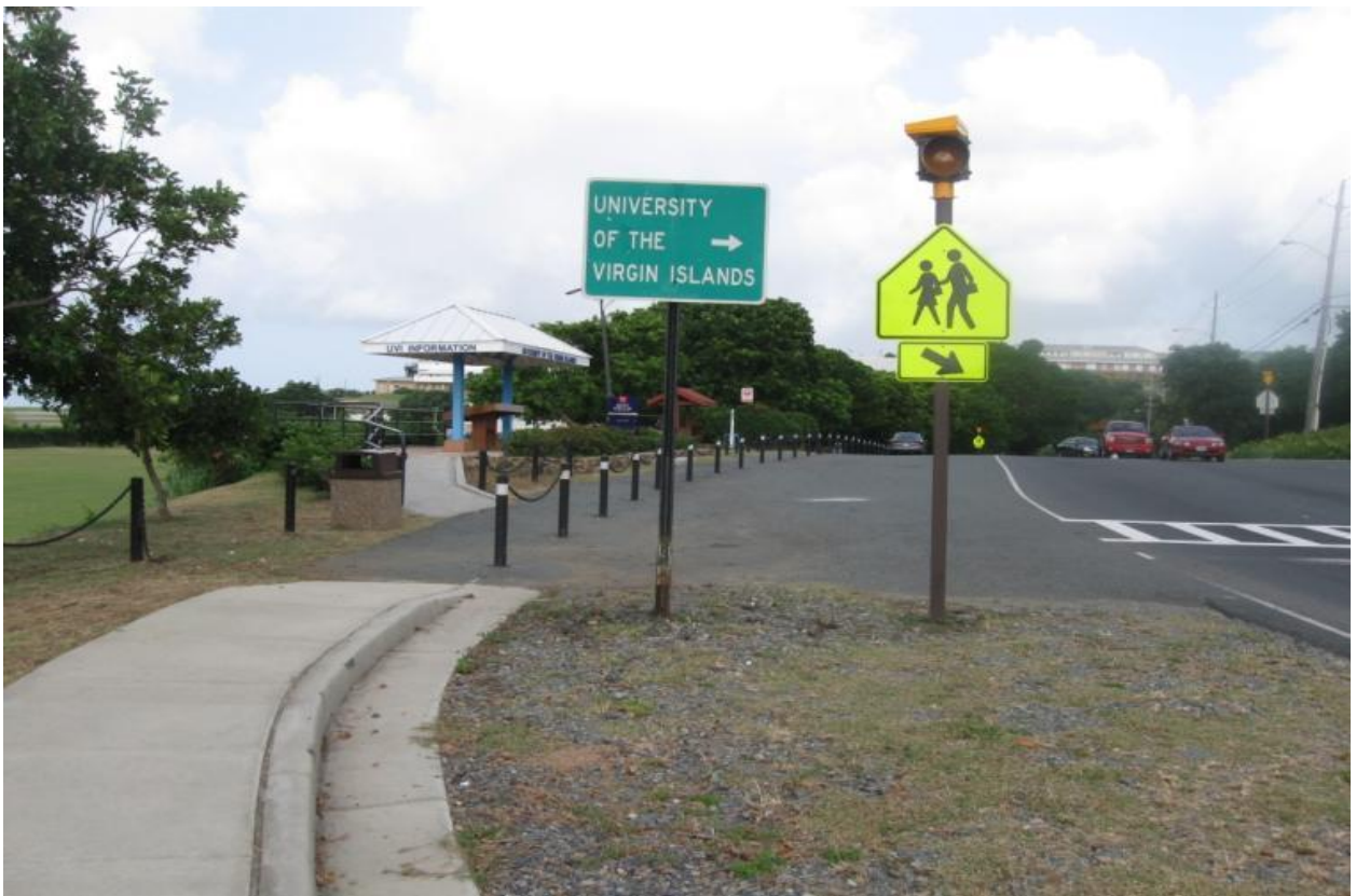
BUS PULL-OFF AFTER SIDEWALK AND BOLLARD INSTALLATION
