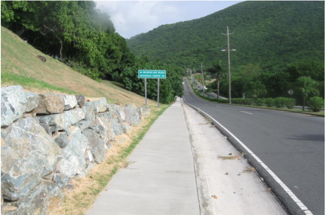
STATION 689+91 AFTER SIDEWALK AND ROCKERY WALL INSTALLATION
