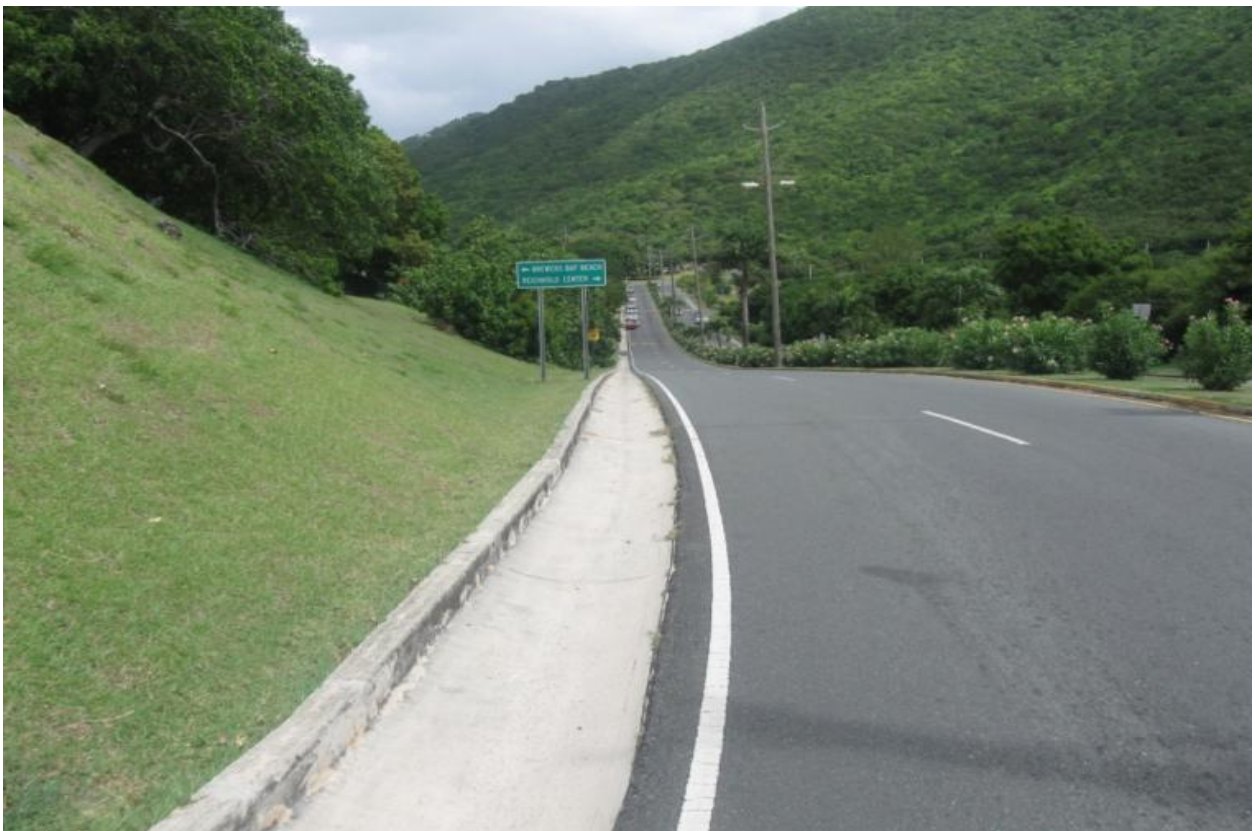
STATION 690+50 PRIOR TO SIDEWALK AND ROCKERY WALL INSTALLATION
