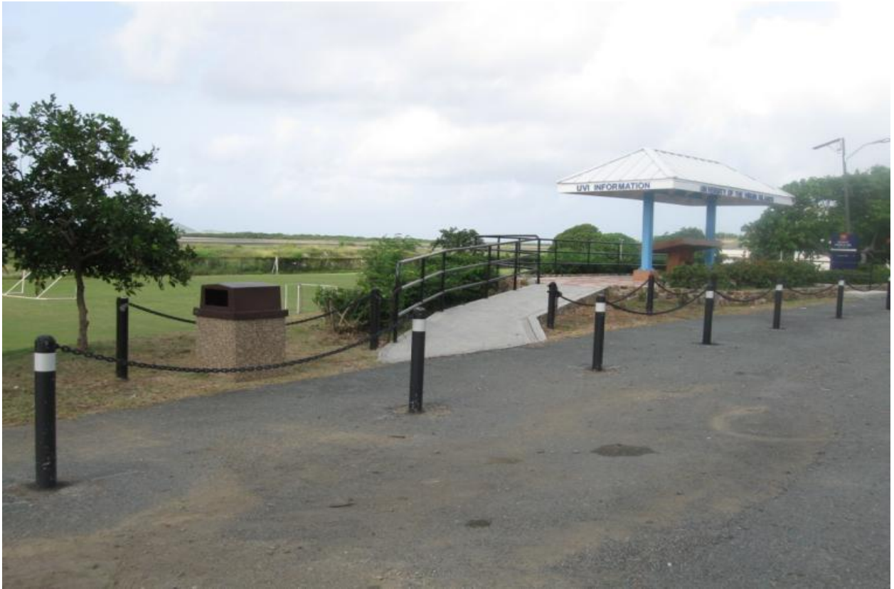
BUS PULL-OFF AFTER SIDEWALK AND BOLLARD INSTALLATION
