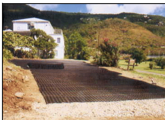
Figure C.12. Geoblock pavement installed at UVI-CES St. Thomas office, prior to filling with soil and seeding (photo by Dale Morton, 1999).
