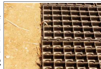
Figure C.13. Geoblock installation close-up, note j-bars used to anchor blocks in place (photo by Dale Morton, 1999).
