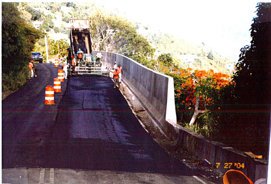
Placing hot asphalt. Rt. 35/40
