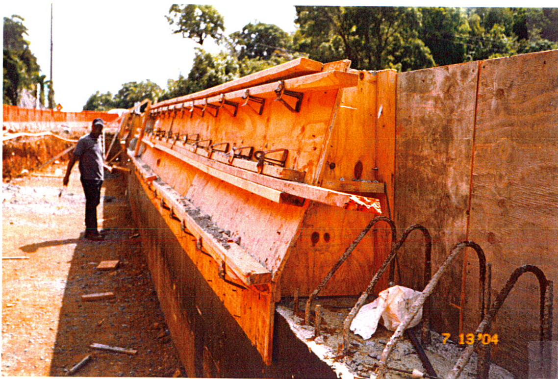
Formwork for parapet. Rt. 35/40
