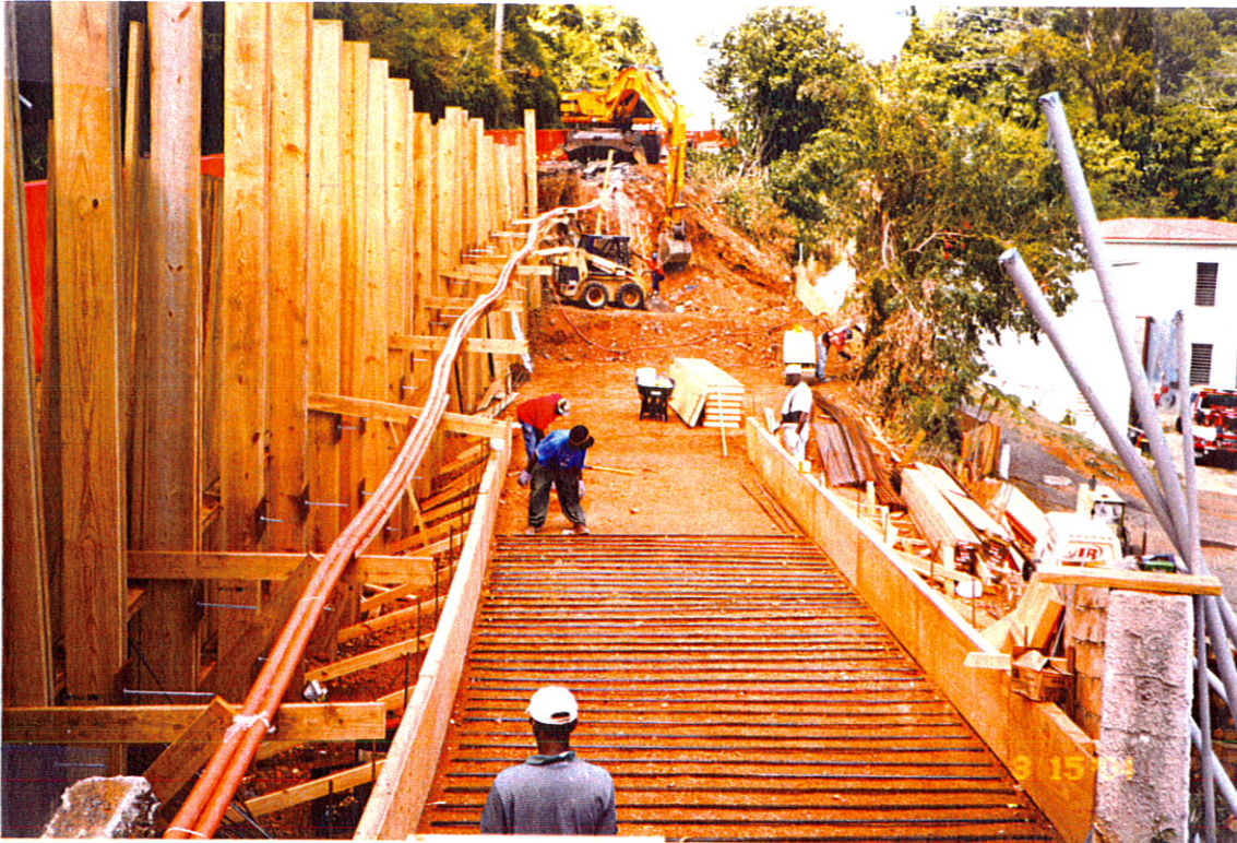
Setting forms and tying rebar for footing. Rt. 35/40
