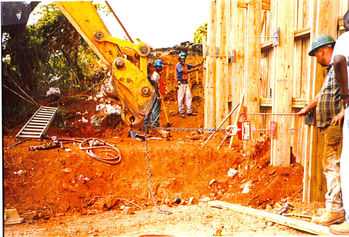
Tensioning soil anchors for shoring system Rt 33
