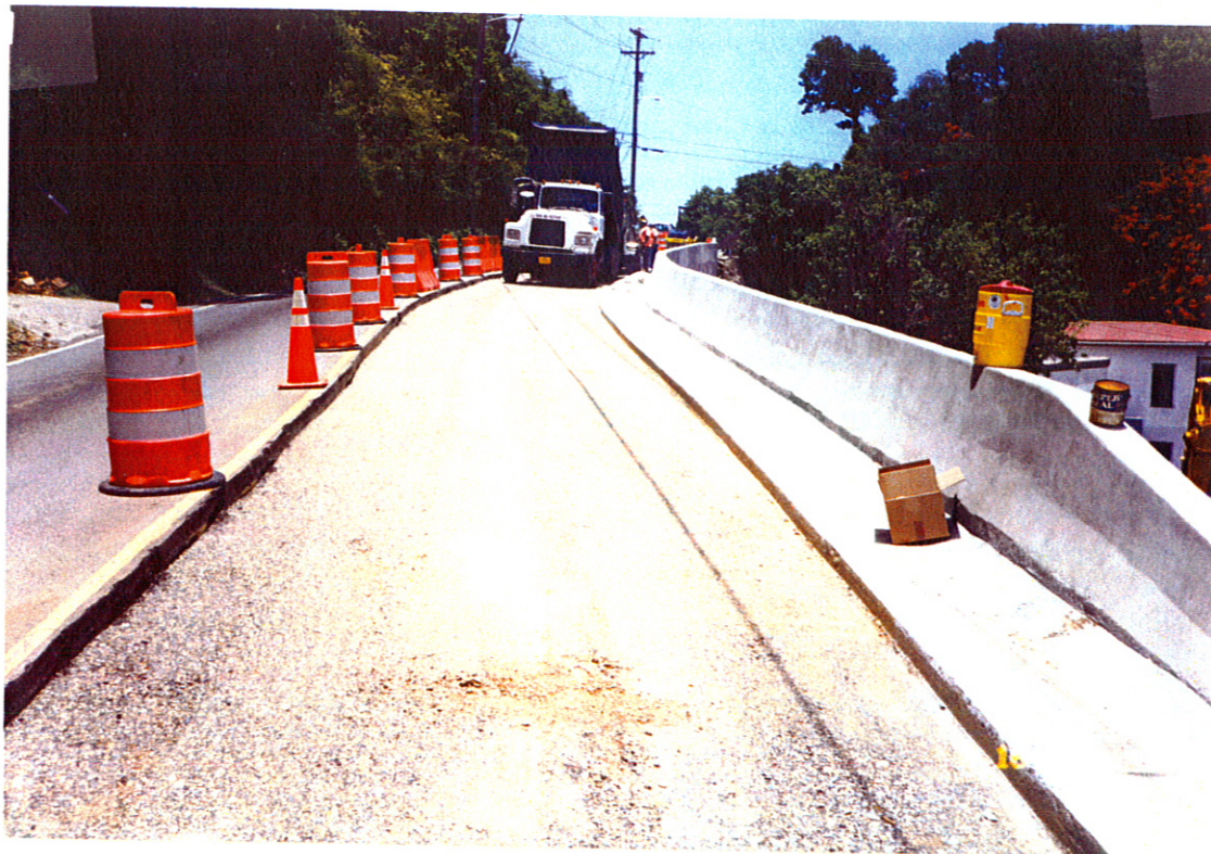
Placing hot asphalt. Rt. 35/40
