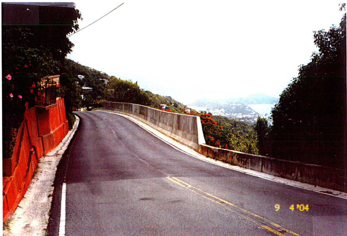
Rt. 33 site after construction.
