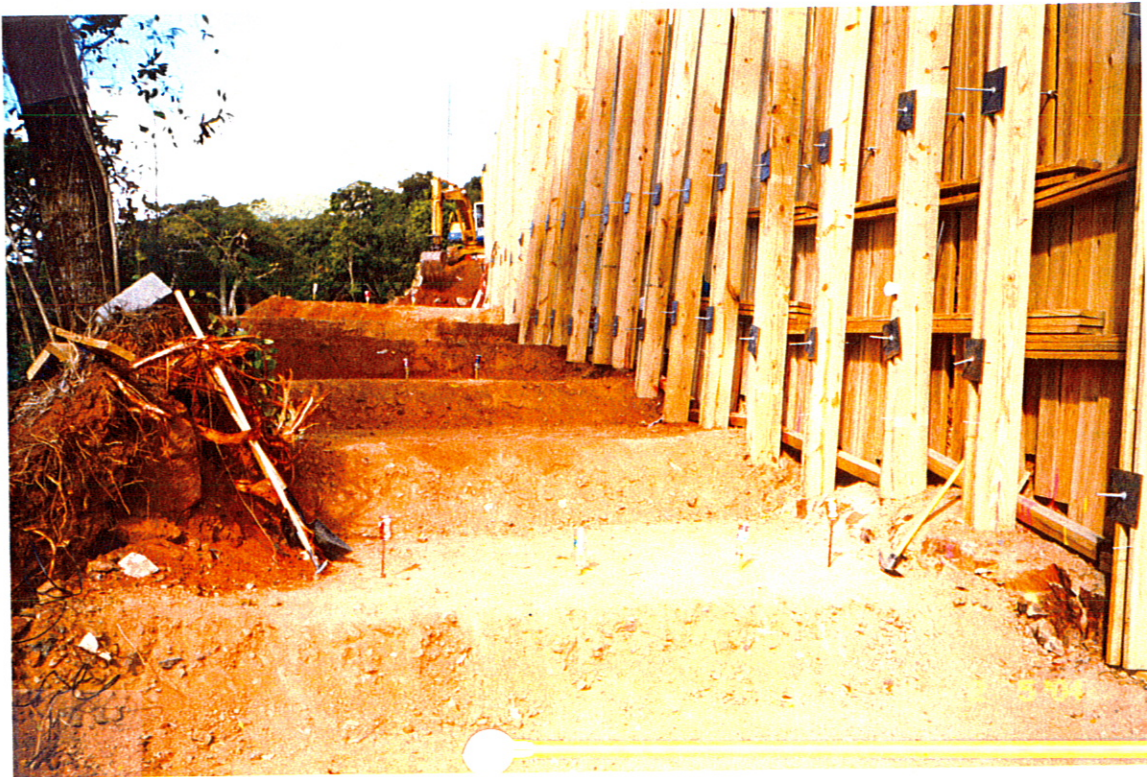
Shoring in place/excavation on grade/ready to set footing forms. Rt 33
