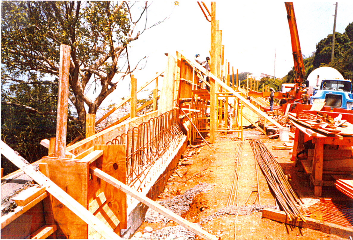
Placing concrete for parapet. Rt. 33
