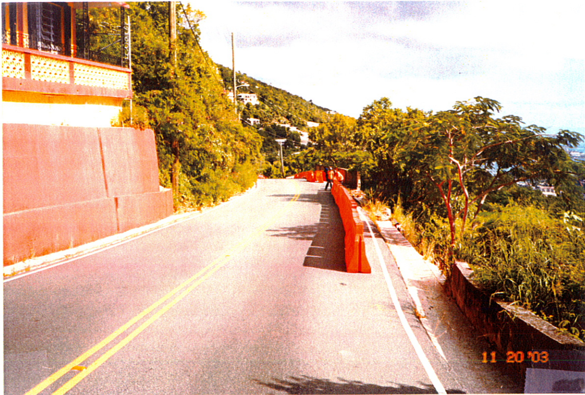
Rt. 33 site before construction.
