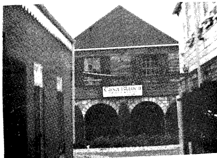
flush sign of inappropriate material and lighting
