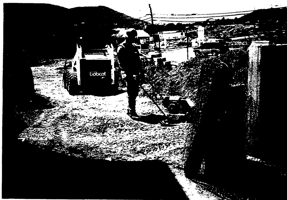
Photo No. 4 - Compacting Clean Backfill Soils in the Excavation Area
