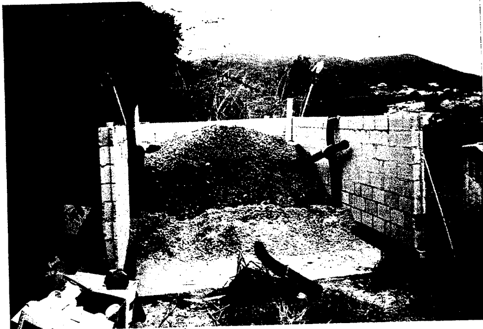
Photo No. 7 - Excavated Soils Were Interlayered With Washed Coarse Gravel
