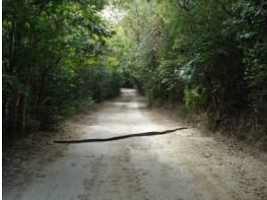
Deflectors along John Head Road.
