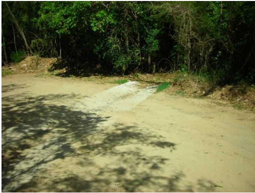
New cemented swale along Cocoloba Trail at Point 2 in map.
