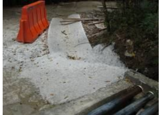
Cemented swale along JH Rd (construction phase).
