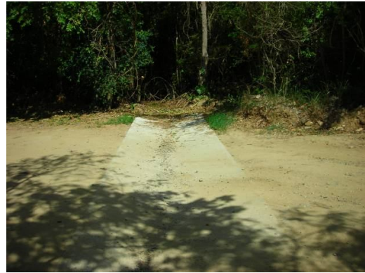
New cemented swale on Cocoloba Trail at Point 1 in map. Swale diverts upslope runoff from flowing over the lowermost sections of Cocoloba Trail.
