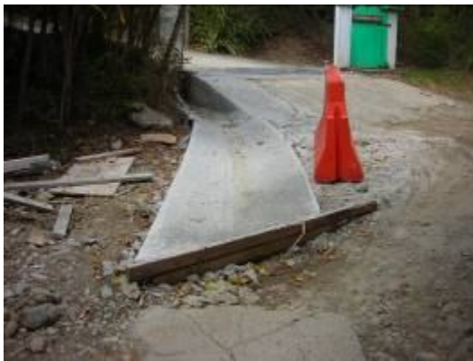
Cemented swale & pre-existing cattle-guard drain along John Head Road (construction phase).
