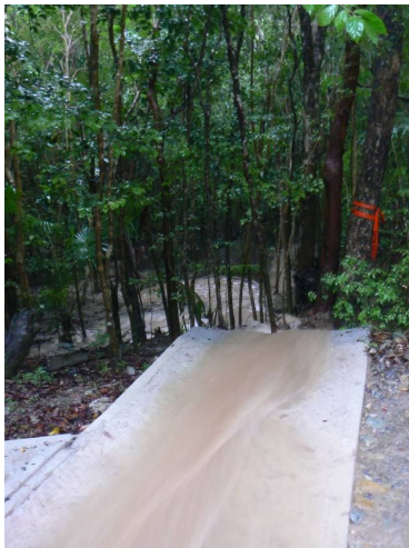
Cemented swales at Points 1 (left) and 3-4 (right) in map during an extreme rainfall event in October 2008. Notice on the picture to the right that some runoff is overtopping the swale and inducing runoff concentration and erosion on the lower portions of the road.
