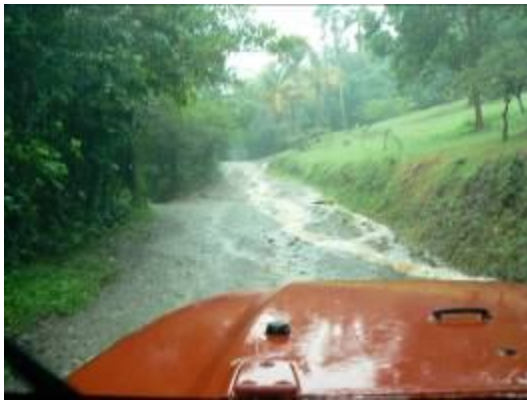
Deflectors during an intense rain event in October 2008. Pictures show that the deflectors were unable to maintain runoff on the inside portions of the road due to runoff overflow and the lack of a new deep ditch.
