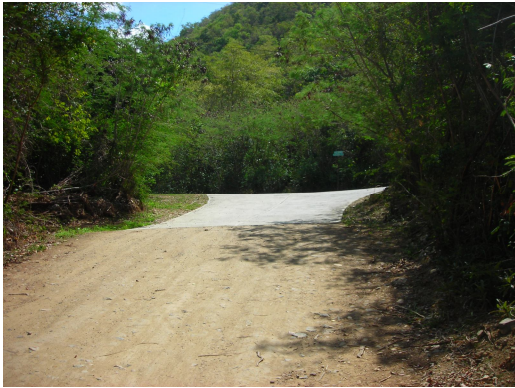
New cemented swale on Cocoloba Trail at Point 1 in map. Swale diverts upslope runoff from flowing over the lowermost sections of Cocoloba Trail.
