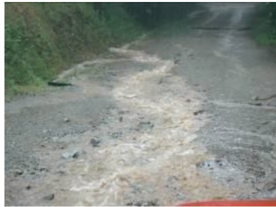
Deflectors during an intense rain event in October 2008. Pictures show that the deflectors were unable to maintain runoff on the inside portions of the road due to runoff overflow and the lack of a new deep ditch.
