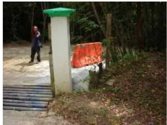
Cemented swale & pre-existing cattle-guard drain along John Head Road (construction phase).
