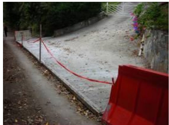
Cemented swale & pre-existing cattle-guard drain along John Head Road (construction phase).
