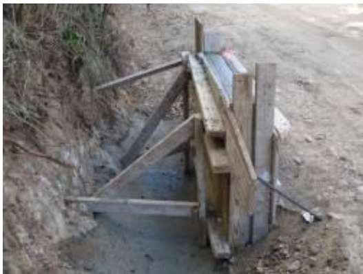
New headwall & culvert installed at Caribe Road (Point 2 in map).
