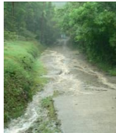
Deflectors during intense rainfall event in October 2008. Picture to the left is a close-up of runoff overtopping the deflector. Picture to the right shows runoff continuing to flow on the road surface instead of the intended purpose to maintain in on the inside ditch.
