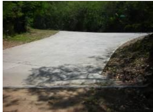
New cemented swale on Cocoloba Trail at Point 1 in map. Swale diverts upslope runoff from flowing over the lowermost sections of Cocoloba Trail.
