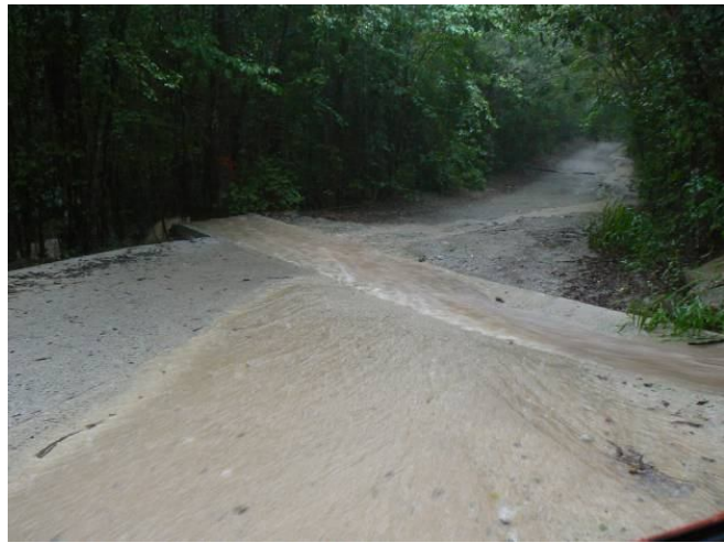
Cemented swales at Points 1 (left) and 3-4 (right) in map during an extreme rainfall event in October 2008. Notice on the picture to the right that some runoff is overtopping the swale and inducing runoff concentration and erosion on the lower portions of the road.
