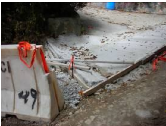
Cement slab and cemented swale along John Head Road (construction phase).
