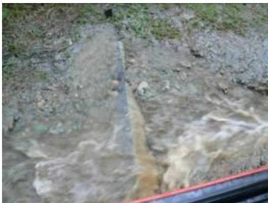
Deflectors during intense rainfall event in October 2008. Picture to the left is a close-up of runoff overtopping the deflector. Picture to the right shows runoff continuing to flow on the road surface instead of the intended purpose to maintain in on the inside ditch.
