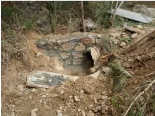
New headwall on pre-existing culvert at Caribe Road (Point 1 in map).
