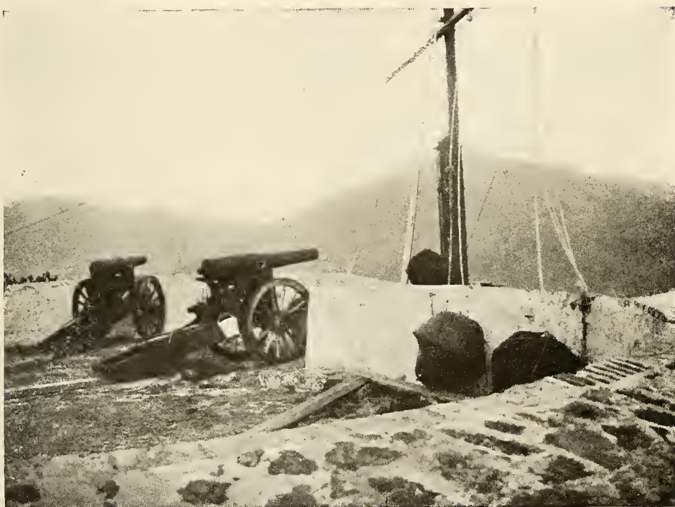
SIGNAL STATION, TOP OF COWELL'S BATTERY
