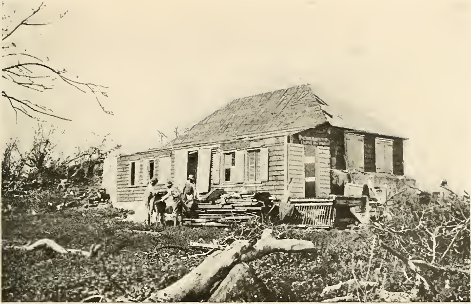
CANAAN ESTATE HOUSE, AFTER HURRICANE
