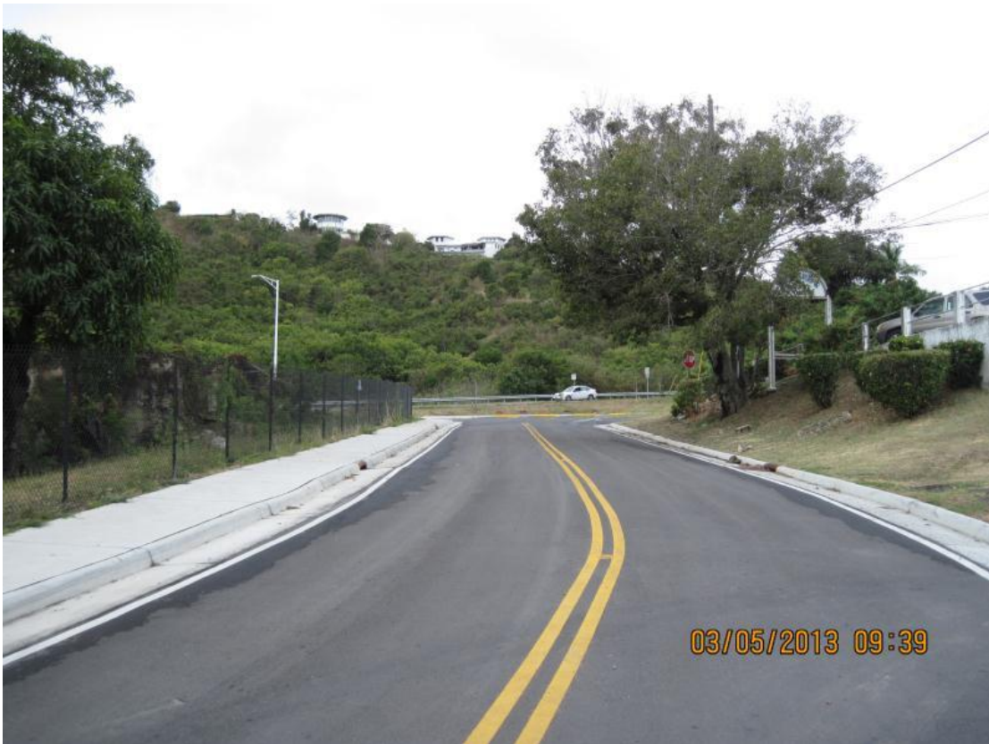
Completed construction - Road Line 7
