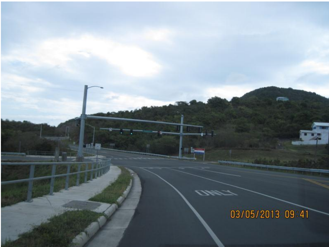
Completed construction - Contentment Road Intersection, Station 41+50
