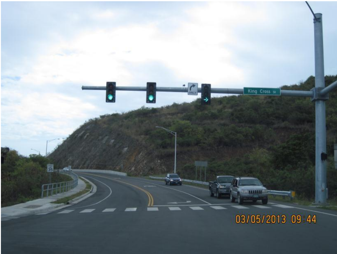
Completed construction - King Cross Street Intersection, Station 76+00
