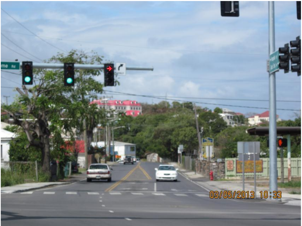
Completed construction - view of Hospital Street from East End Intersection
