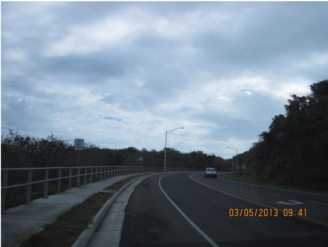
Completed construction - Station 43+00
