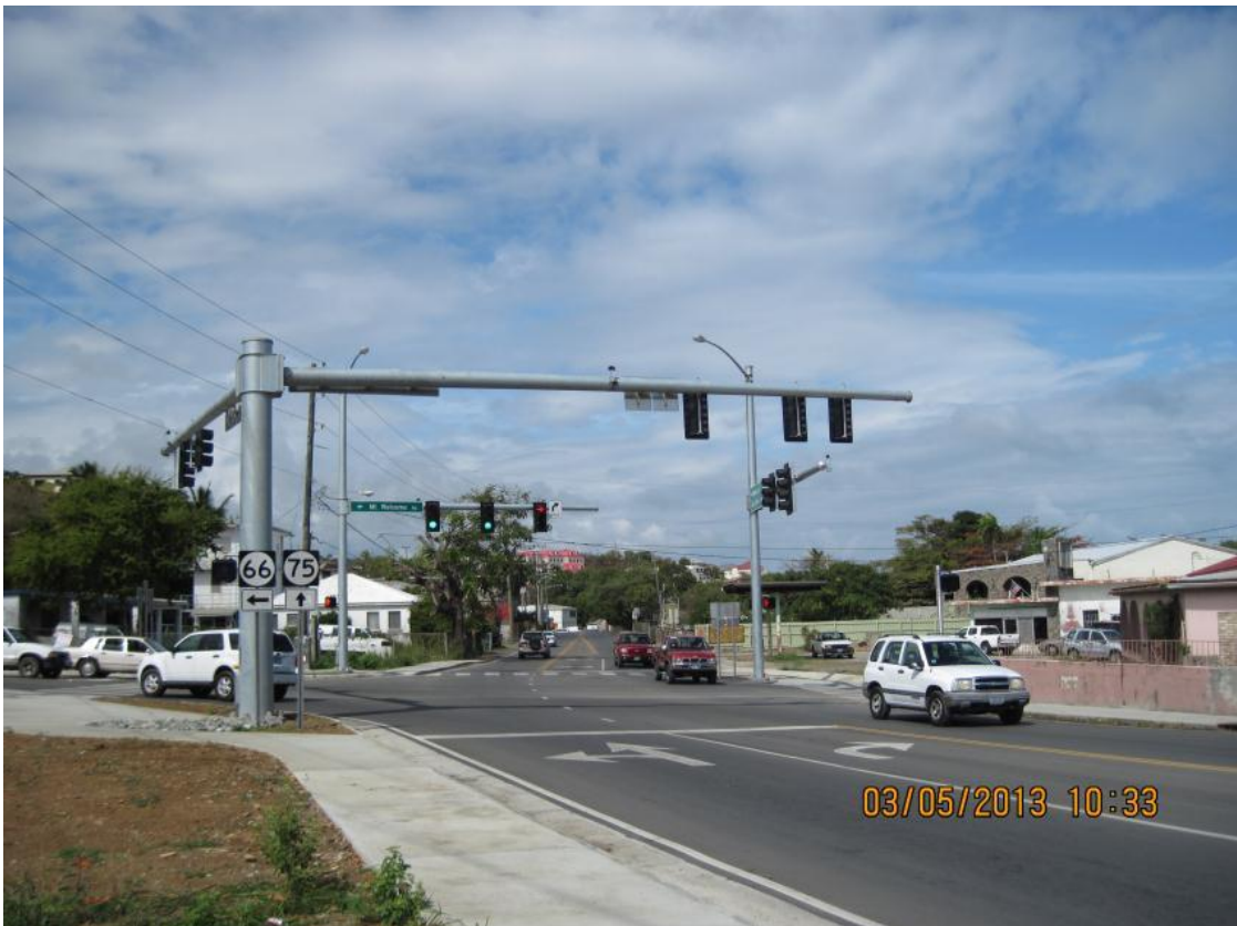
Completed construction - East End Intersection, Station 99+80
