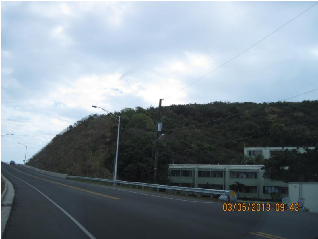
Completed construction - Station 59+00
