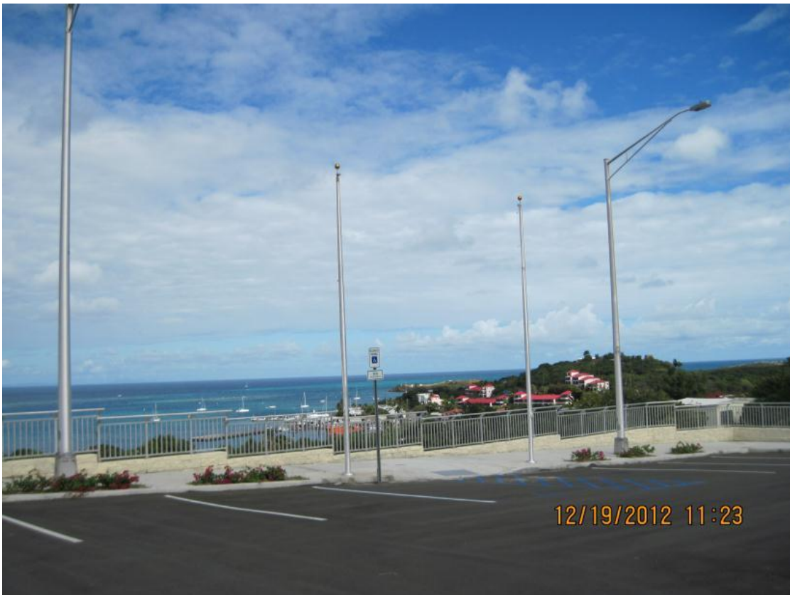
Completed construction - new Outlook Parking Area, Station 86+00
