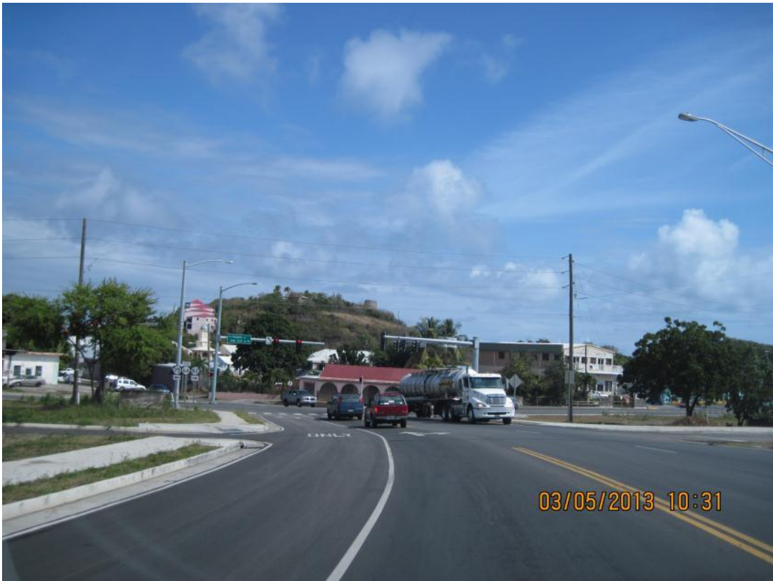
Completed construction, Station 97+50
