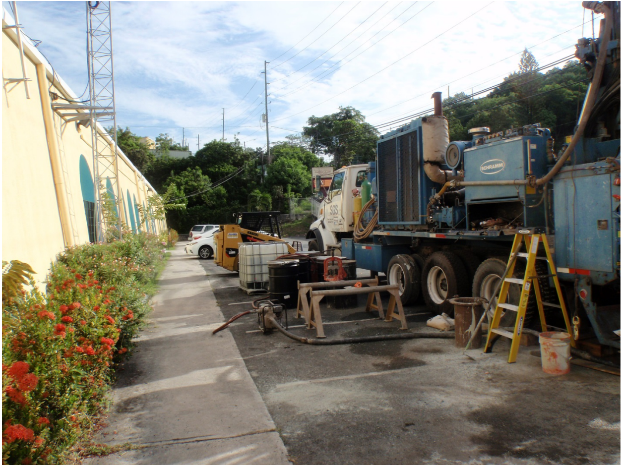
Photograph 1: View east of Tutu Wells South Project area showing geotechnical drilling equipment.
