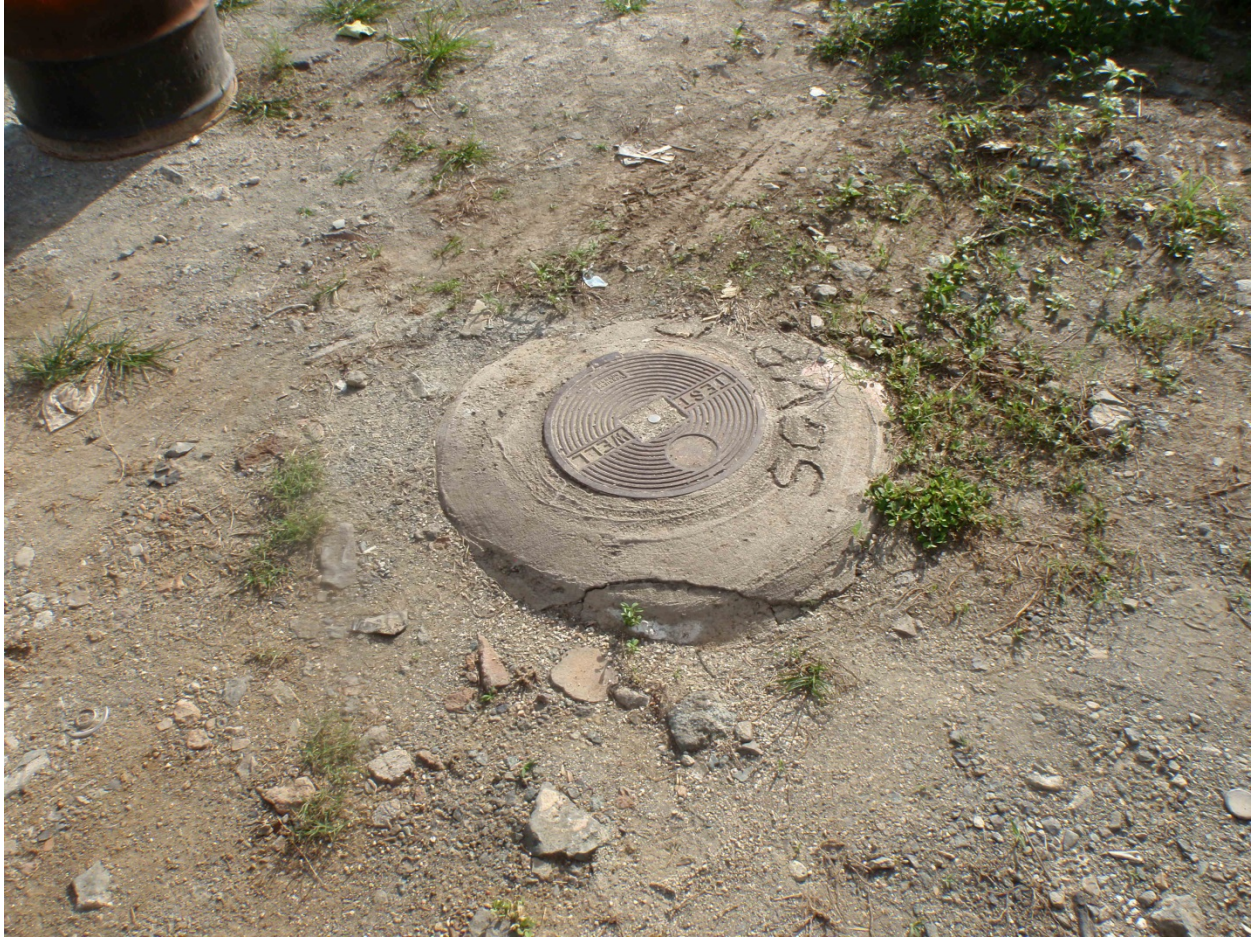
Photograph 11: Closeup of preexisting well location and graded rocky surface.
