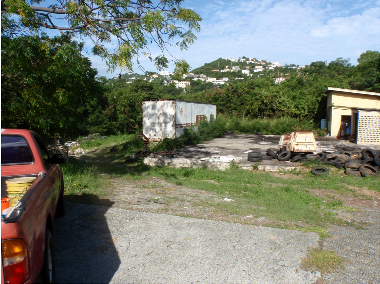
Photograph 18: View north of rear sector of Housing Authority.
