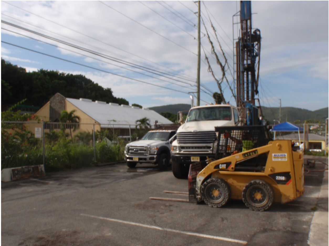
Photograph 3: View southwest of Curriculum Center parking area.
