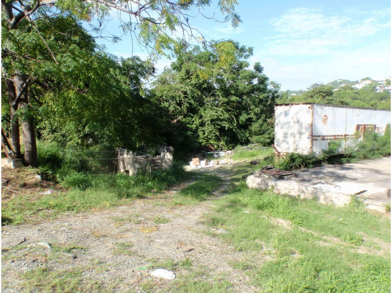
Photograph 19: View northwest of rear of Housing Authority showing graded and disturbed surface.
