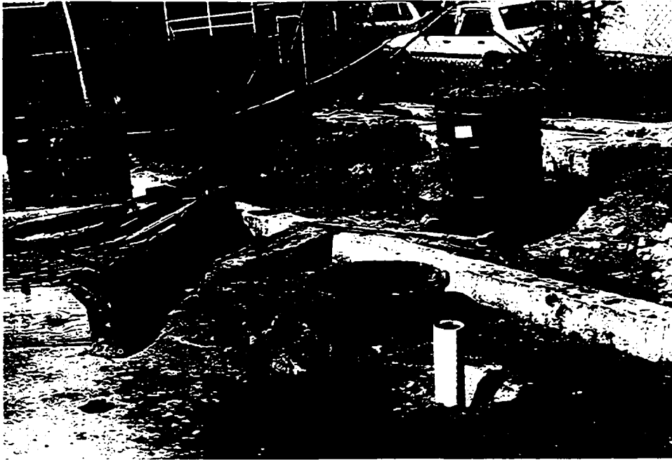
(9) Blank casing (arrow) was set over well screens in each monitor well. The casing was cut off below-grade after grouting.
