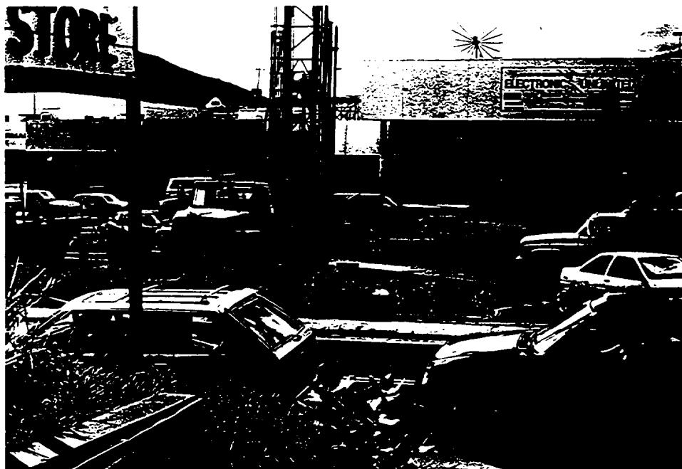
(7) View, looking west, of drill rig set up over TT-6, in Four Winds Shopping Center parking lot.
