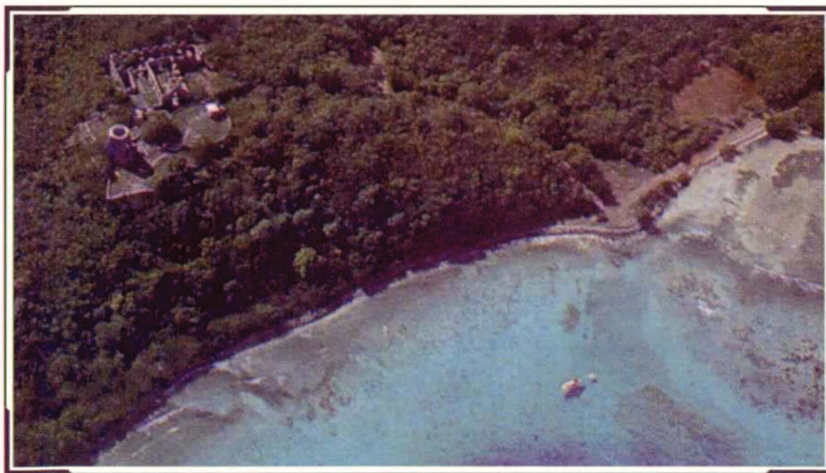
Above: Annaberg Factory Complex, ruins of the windmill , November 2000 (Photograph by D. Knight, 2000)
