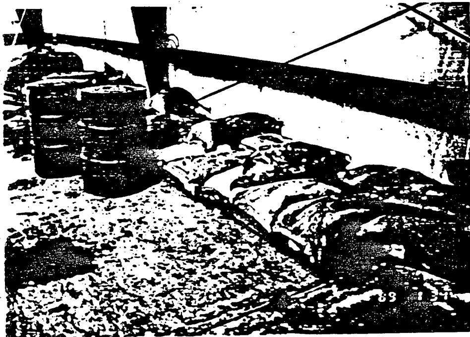
Photo #21. Deteriorating bags in area 6
