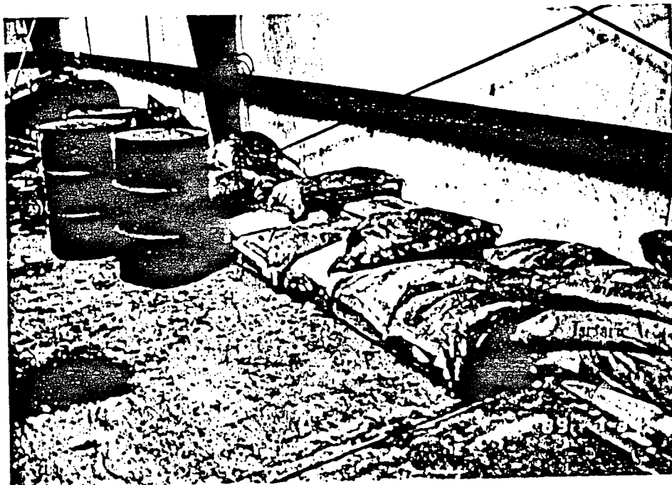
Photo #21. Deteriorating bags in area 6
