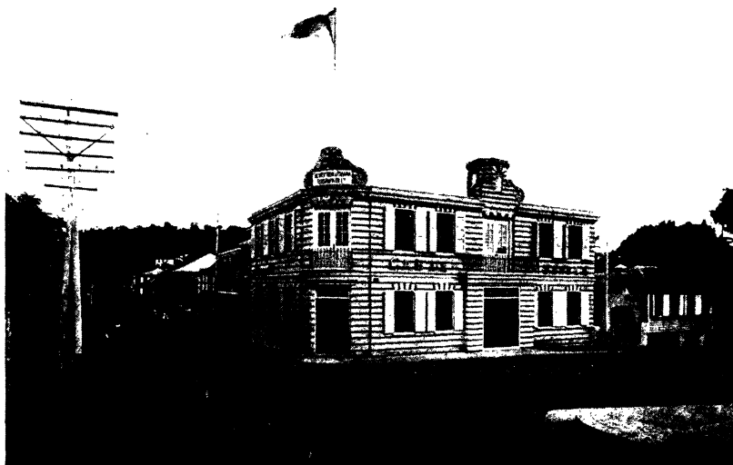
Cable Office, St. Thomas
