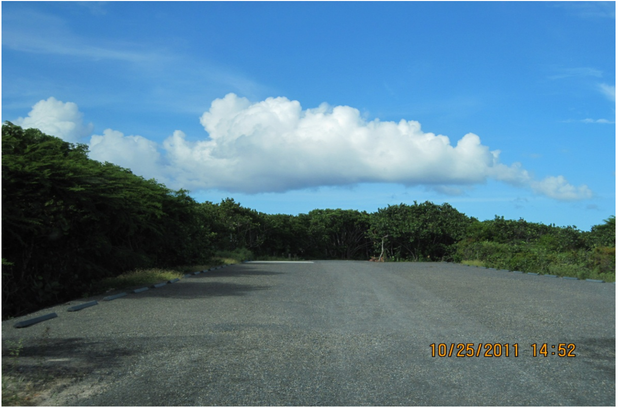
NEW PARKING AREA ON ROUTE 904, STATION 111+00
