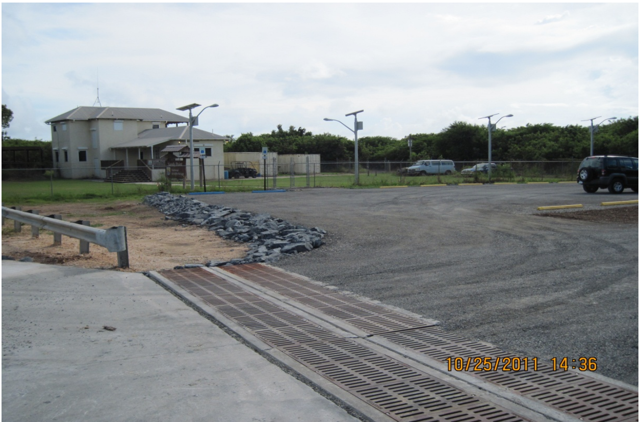
REFUGE ENTRANCE AND MAIN PARKING LOT AFTER REHABILITATION
