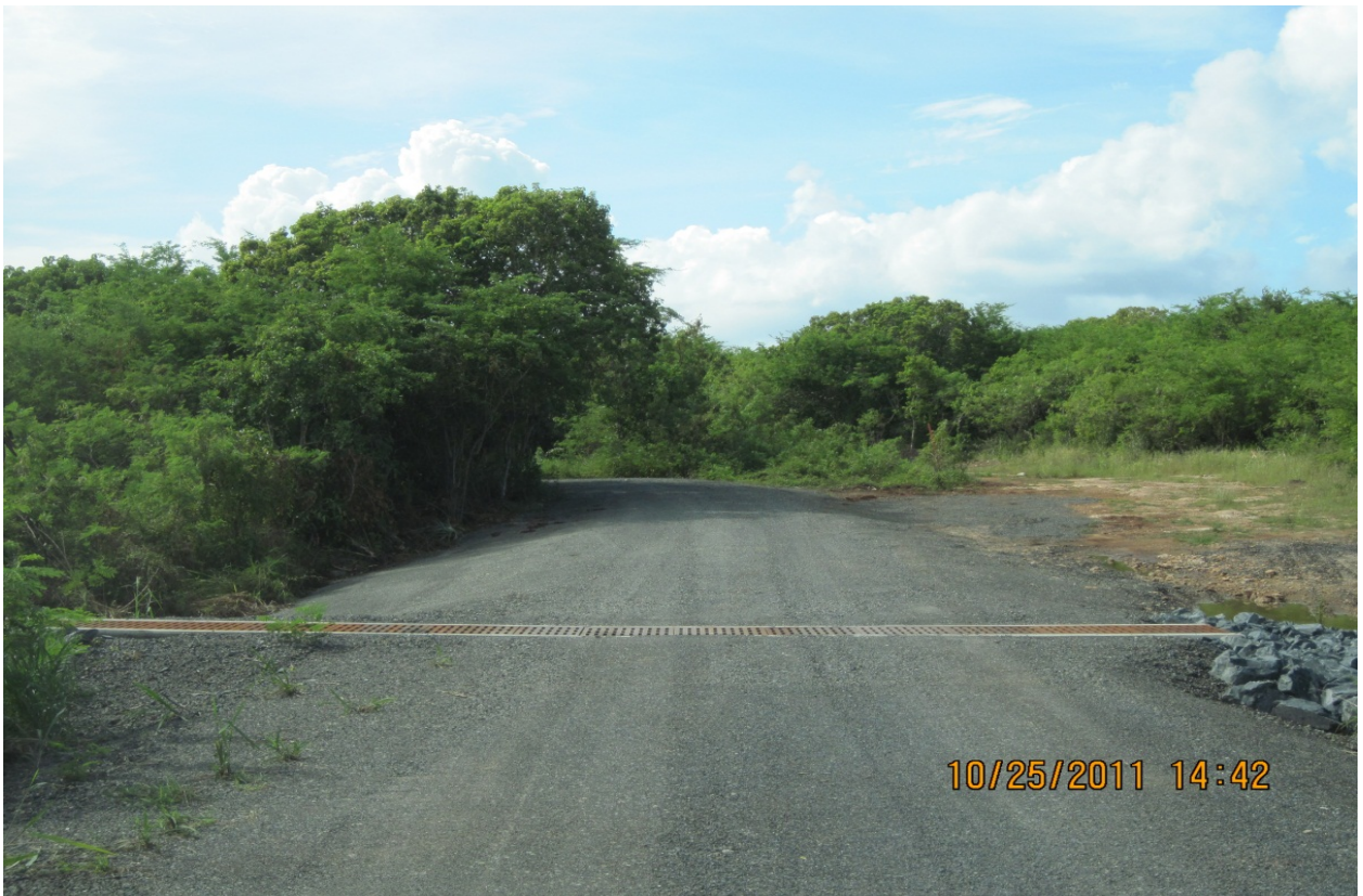
STATION 20+00 OF TRANBERG ROAD AFTER REHABILITATION
