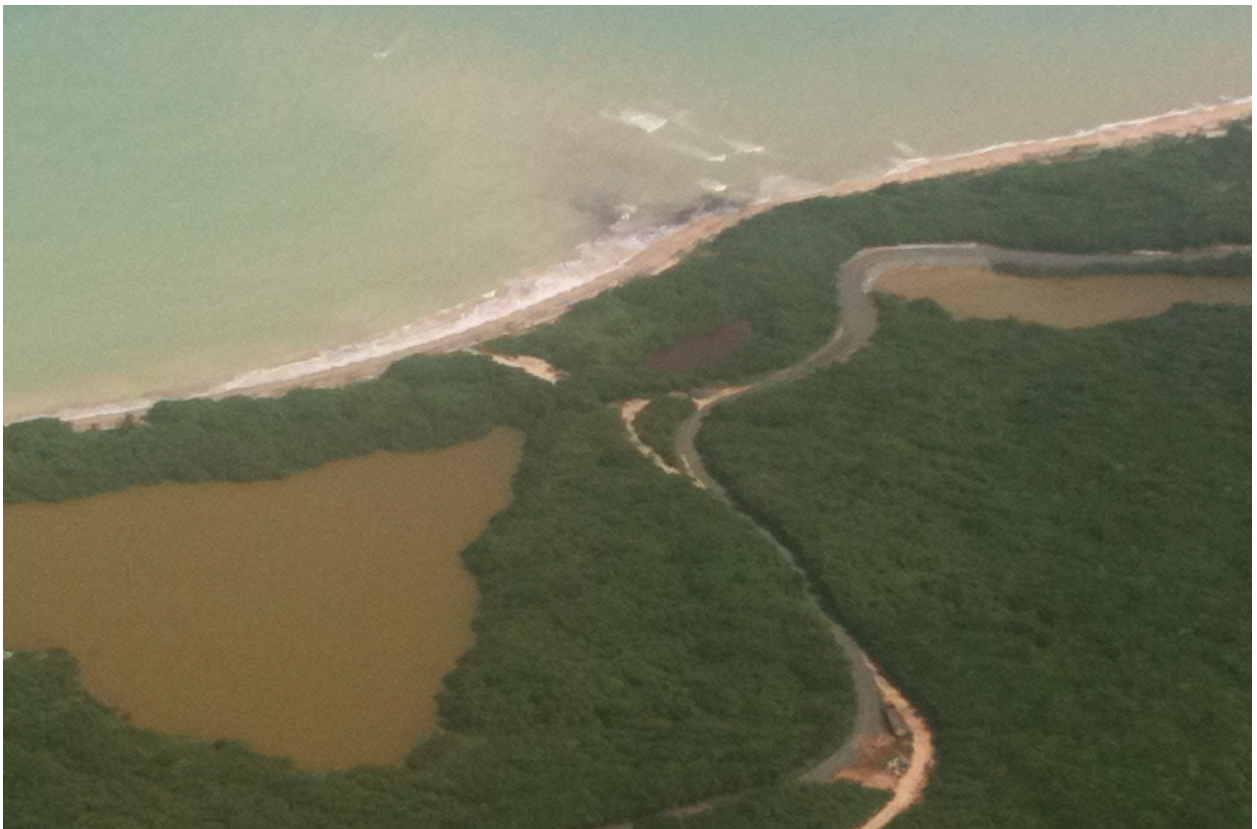
AERIAL VIEW OF THE TRANBERG ROAD AFTER REHABILITATION
