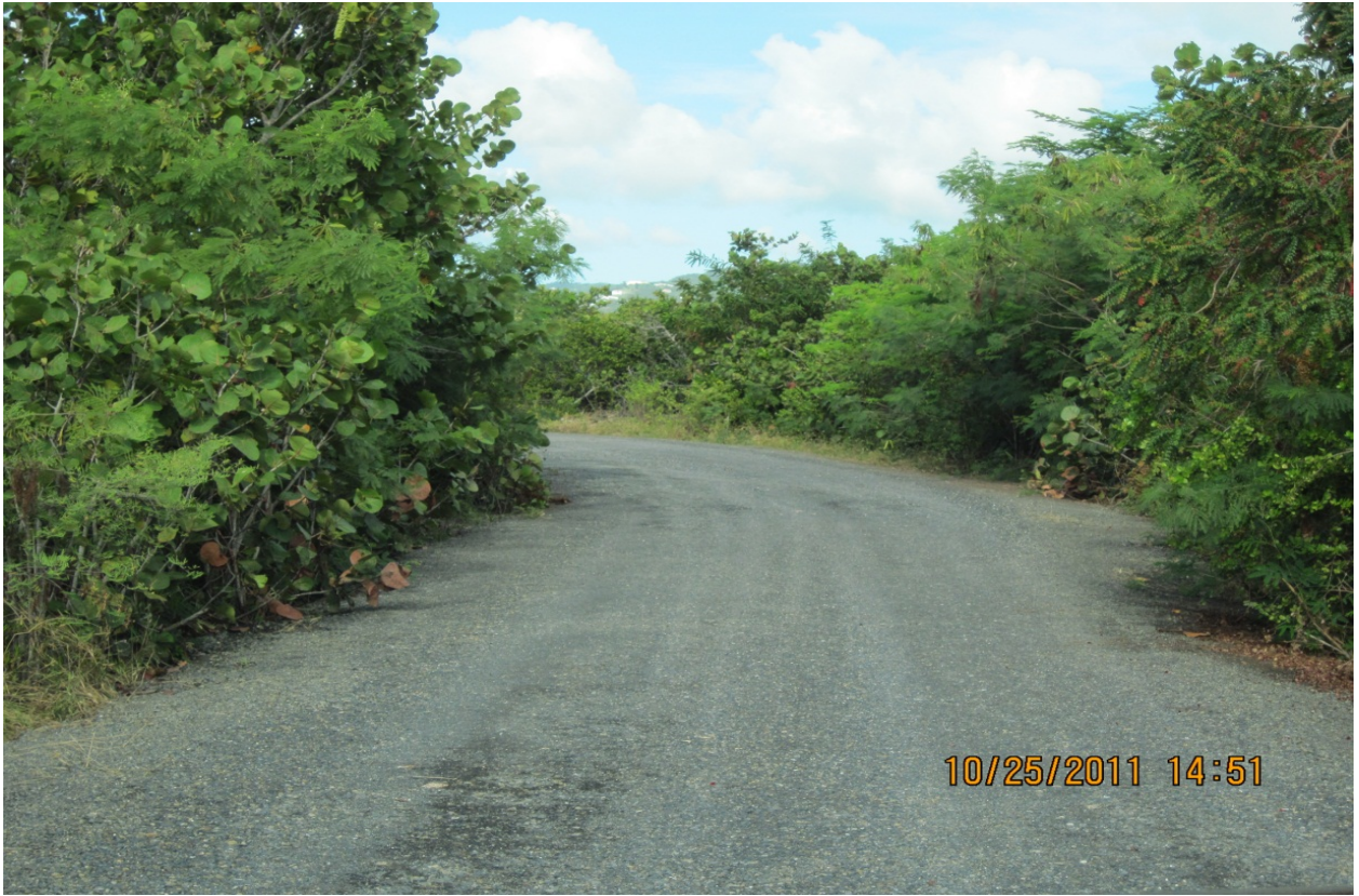
STATION 95+00 OF TRANBERG ROAD AFTER REHABILITATION
