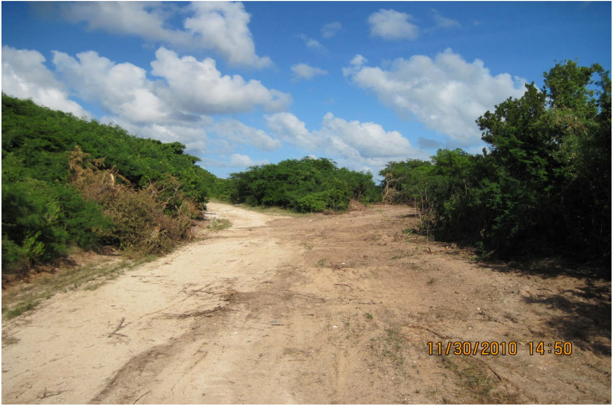
STATION 20+00 OF TRANBERG ROAD BEFORE REHABILITATION
