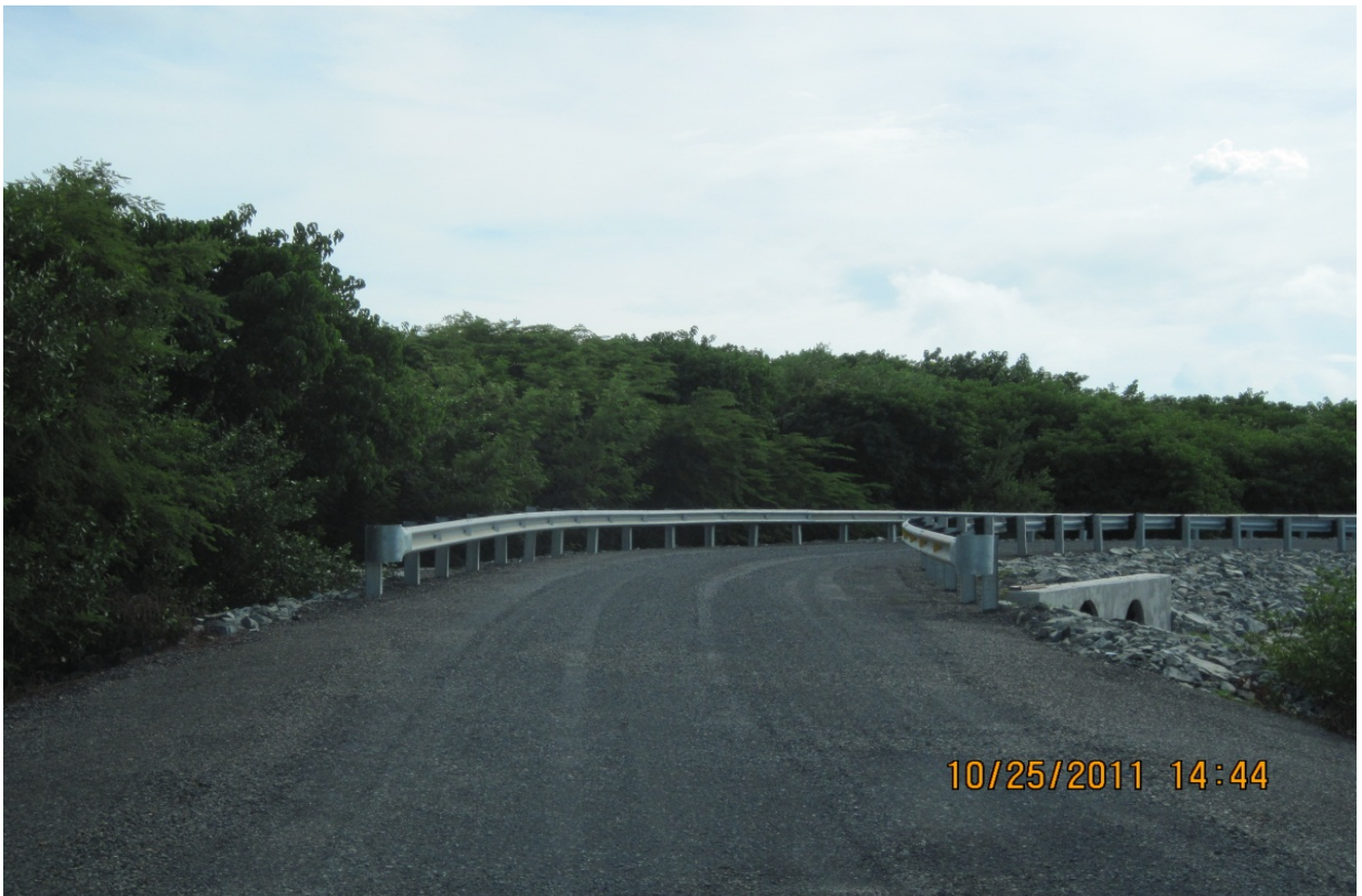
STATION 36+00 OF TRANBERG ROAD AFTER REHABILITATION
