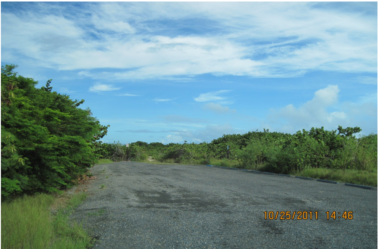
NEW PARKING AREA ON ROUTE 901, STATION 68+00
