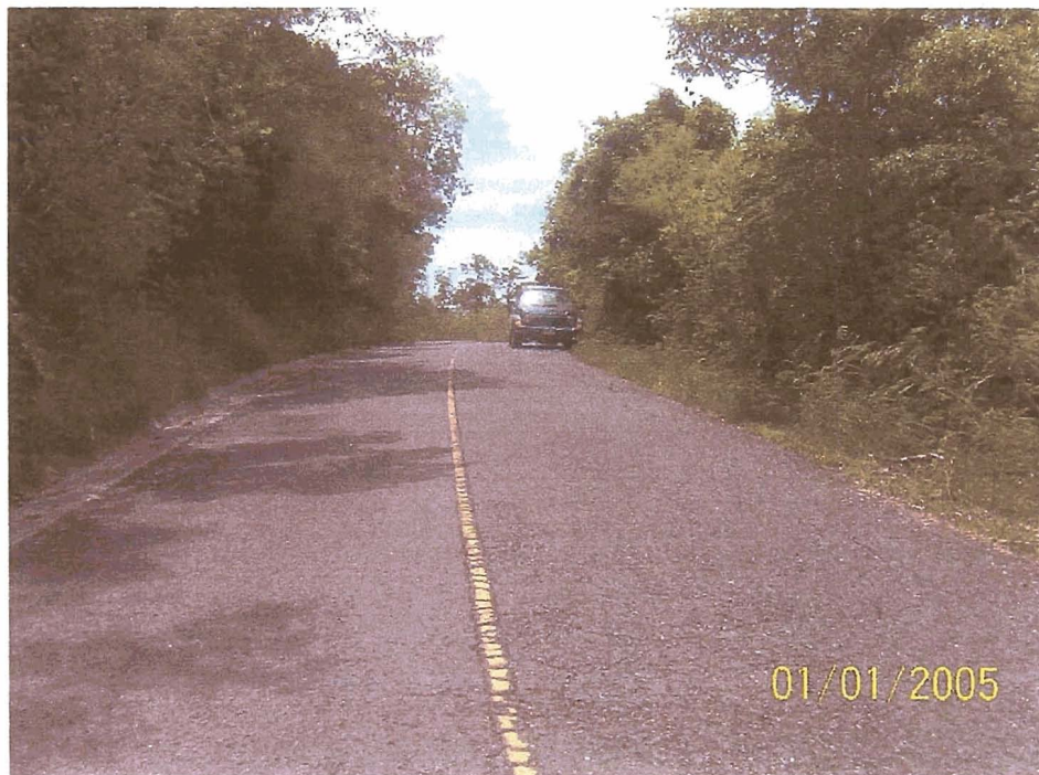
PRA VIIS 100(2) SITE # 11 (PENN POINT DROP OFF) EXISTING CONDITIONS PRIOR TO CONSTRUCTION Photo taken looking west from end of realignment toward curve at top of hill
