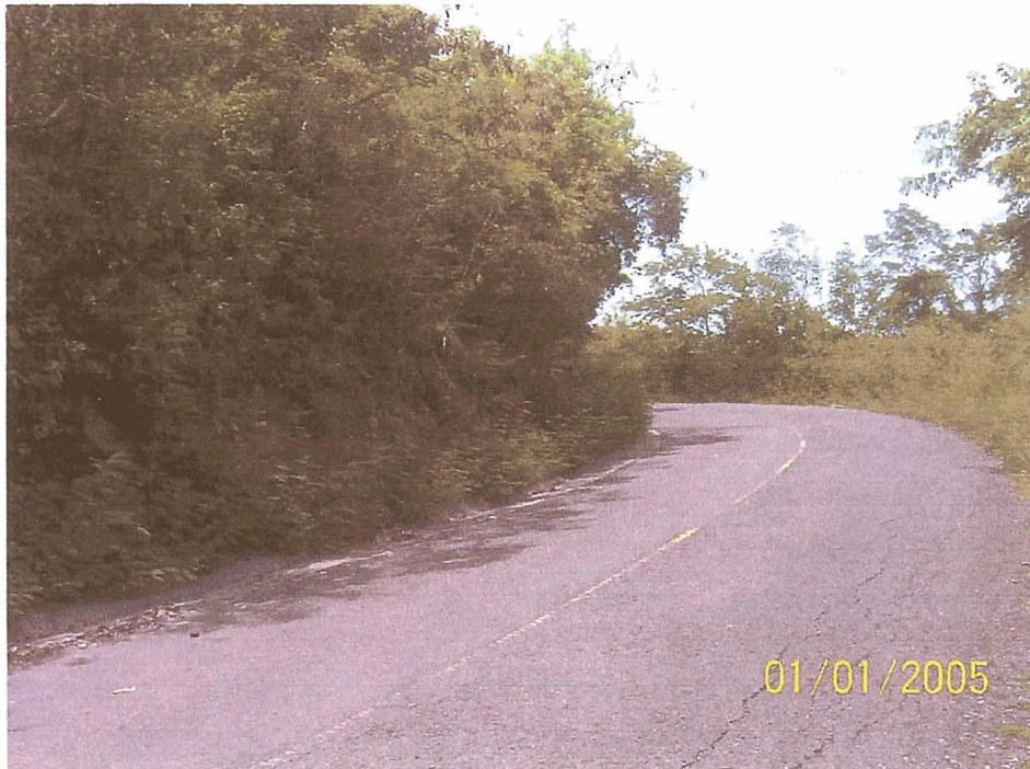
PRA VIIS 100(2) SITE # 11 (PENN POINT DROP OFF) EXISTING CONDITIONS PRIOR TO CONSTRUCTION Photo taken looking west toward end of realignment around curve
