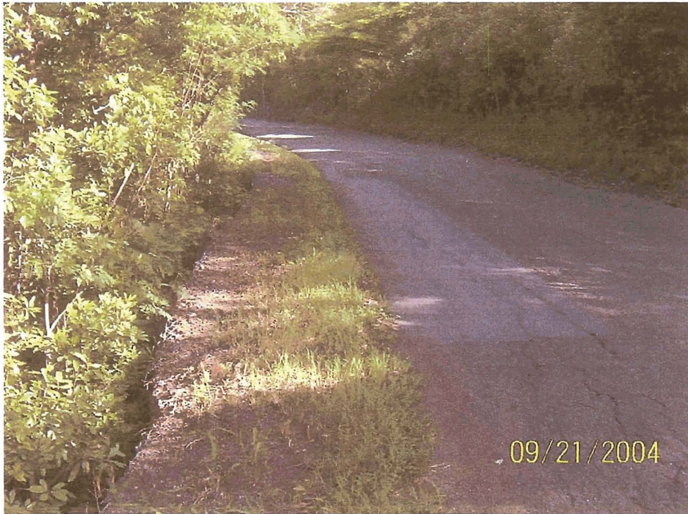
PRA VIIS 100(2) SITE # 2 EXISTING CONDITIONS PRIOR TO CONSTRUCTION Photo taken looking condition of gabion baskets to be removed and replaced
