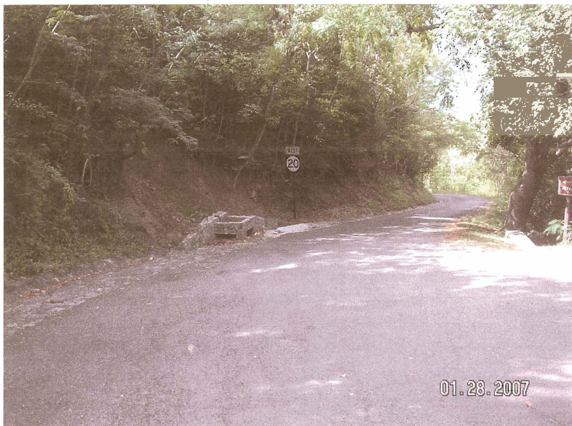
PRA VIIS 100(2) SITE # 13 AS BUILT CONDITIONS Photo taken looking toward inlet and culvert replaced.
