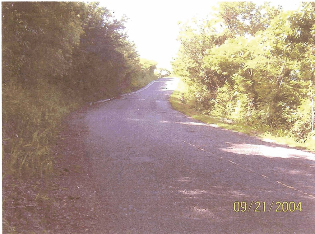
PRA VIIS 100(2) SITE # 2 EXISTING CONDITIONS PRIOR TO CONSTRUCTION Photo Take looking from east end of site toward west end at top of hill
