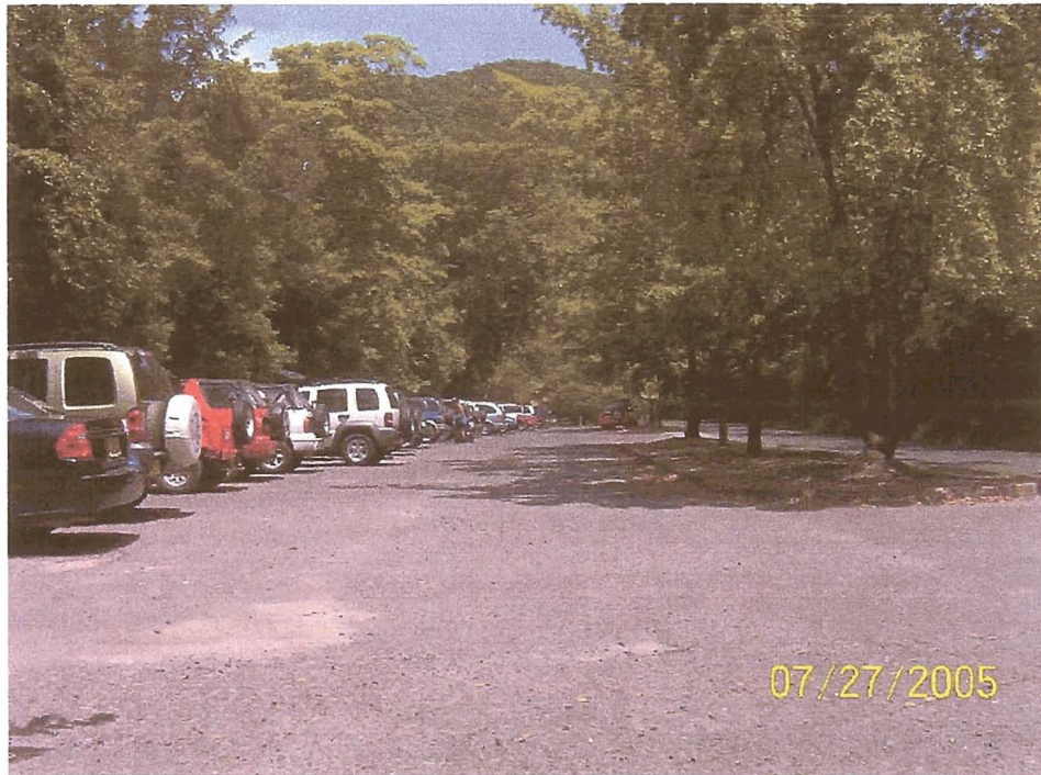
PRA VIIS 100(2) SITE #3 (HAWKSNEST PARKING AREA) EXISTING CONDITIONS PRIOR TO CONSTRUCTION Photo taken looking center of parking site toward west end
