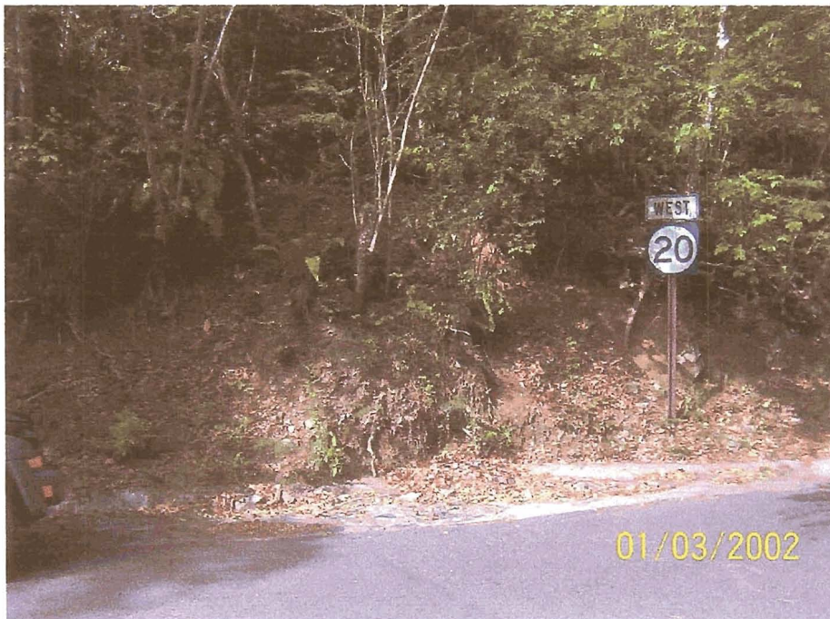
PRA VIIS 100(2) SITE # 13 EXISTING CONDITIONS PRIOR TO CONSTRUCTION Photo taken looking toward existing inlet and culvert replaced
