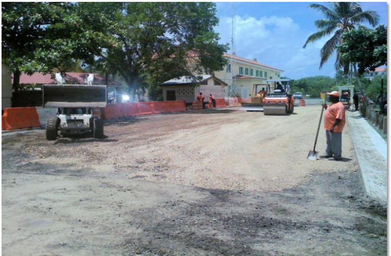
NPS PARKING LOT RECONSTRUCTION AFTER TROPICAL STORM OTTO (SCHEDULE D)
