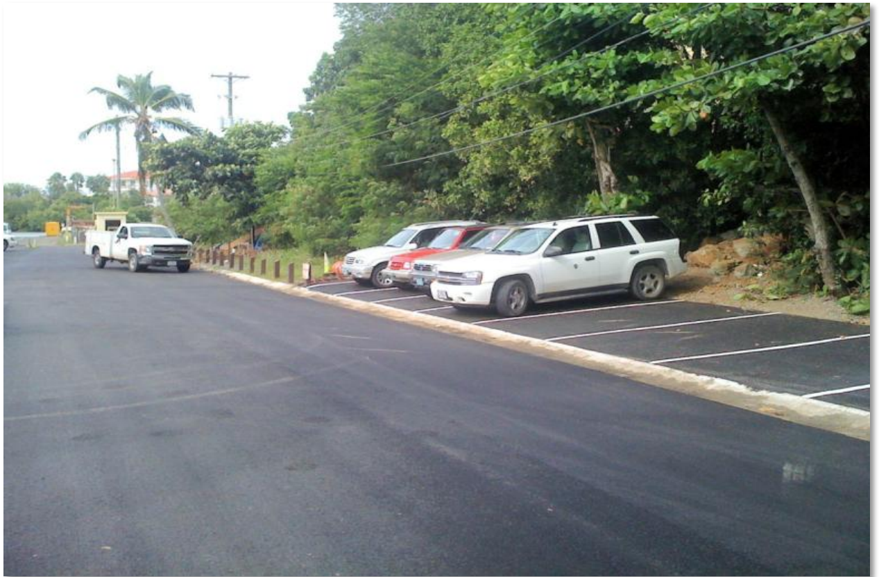
PAVED NPS HEADQUARTERS PARKING LOT WITH PARKING EXTENSION
