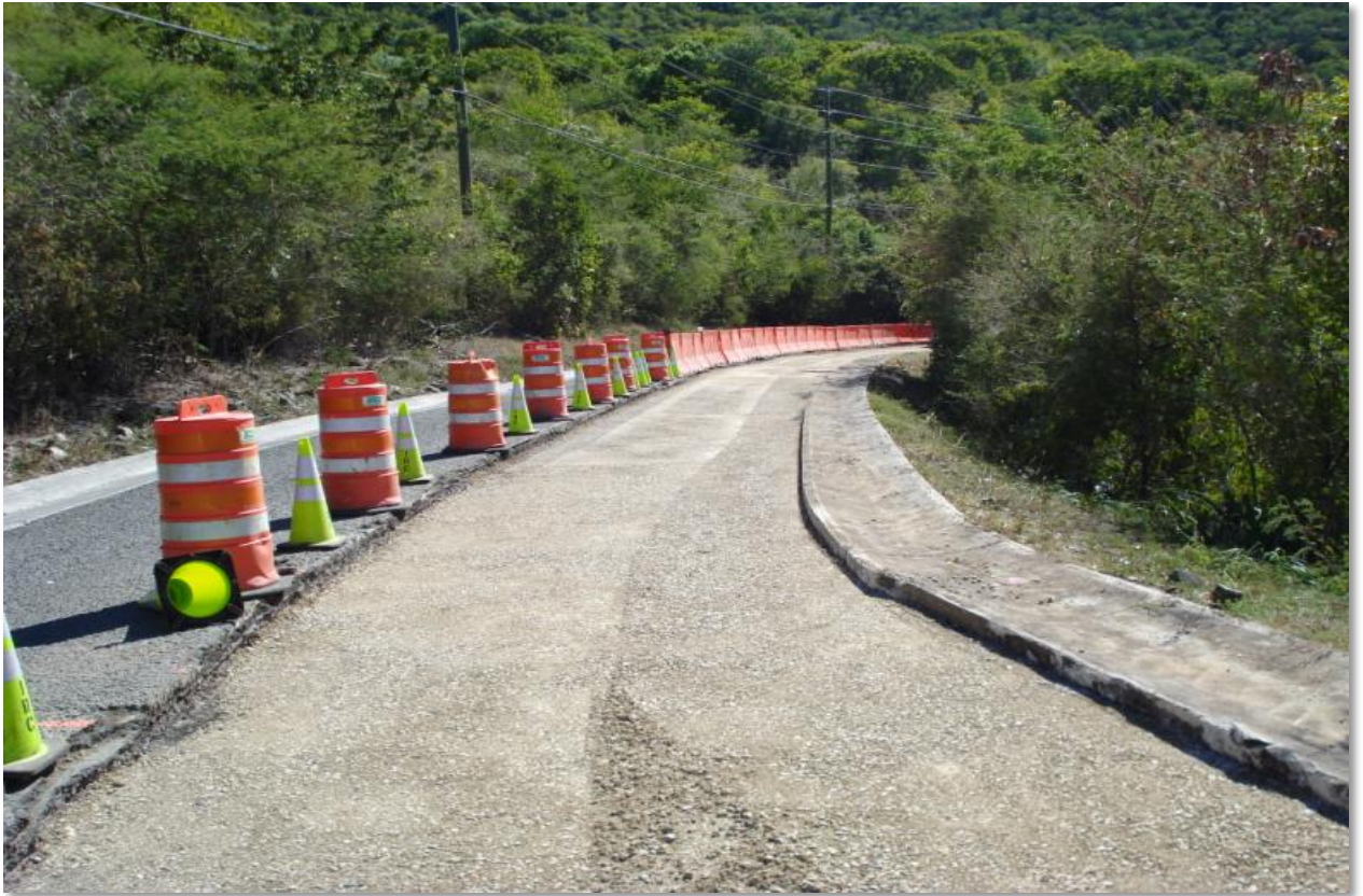
AGGREGATE BASE PLACEMENT FOR EDGE STABILIZATION AT STATION 106+00 (SCHEDULE A)
