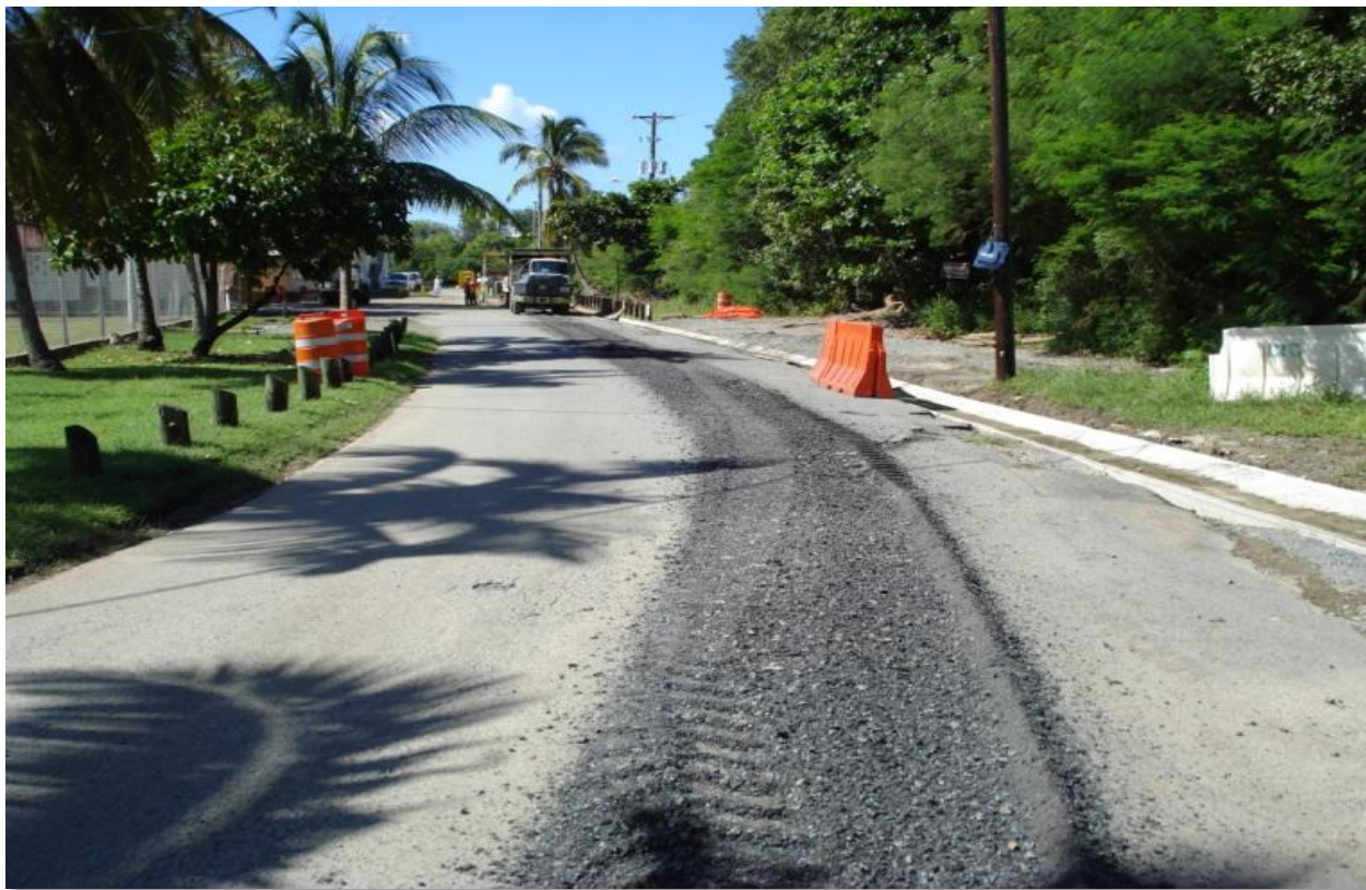
NORTH SHORE ROAD (ROUTE 10A) TOWARDS NPS HEADQUARTERS PARKING LOT DURING CONSTRUCTION
