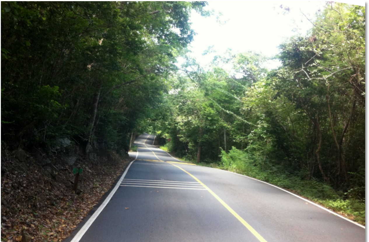
THERMOPLASTIC RUMBLE STRIPS AT STATION 246+00
