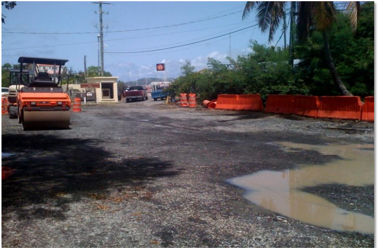
MILLING AT NPS HEADQUARTERS PARKING LOT (SCHEDULE D)
