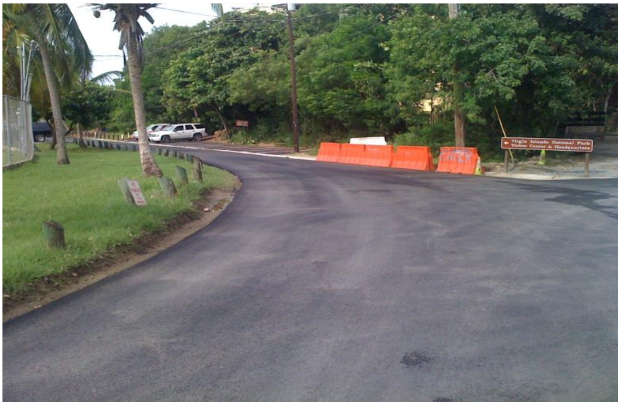
PAVED NORTH SHORE ROAD (ROUTE 10A) TOWARDS NPS HEADQUARTERS PARKING LOT AREA AFTER CONSTRUCTION
