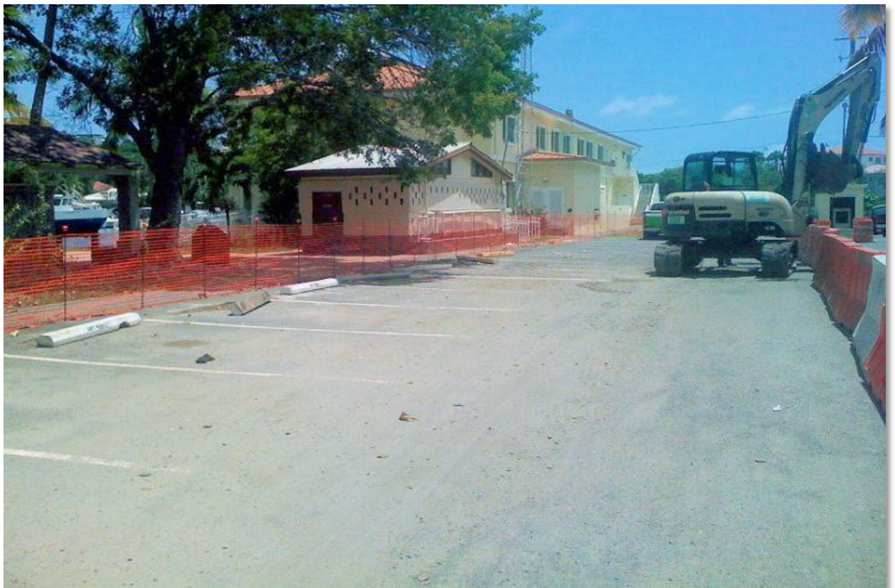
NPS HEADQUARTERS PARKING LOT PREPARATION (SCHEDULE D)
