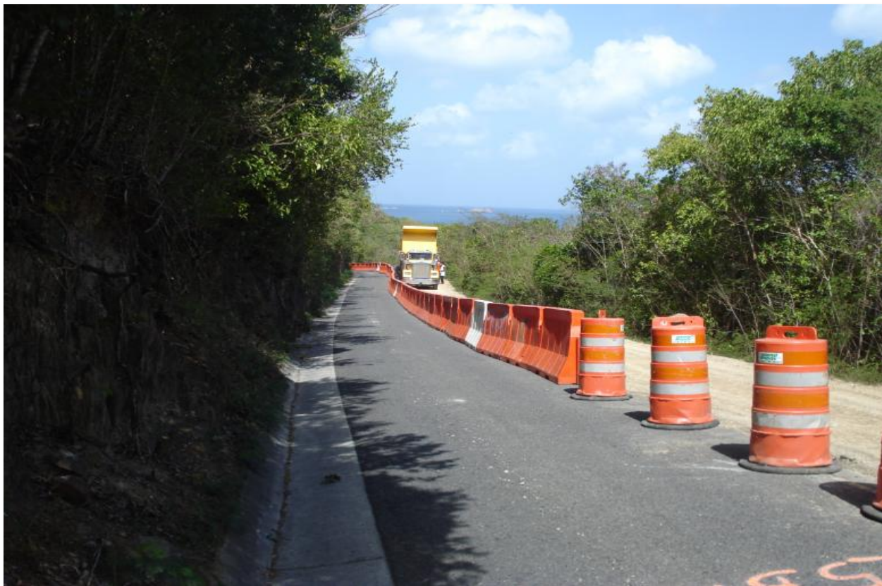
EDGE STABILIZATION AT STATION 253+62 (SCHEDULE B)
