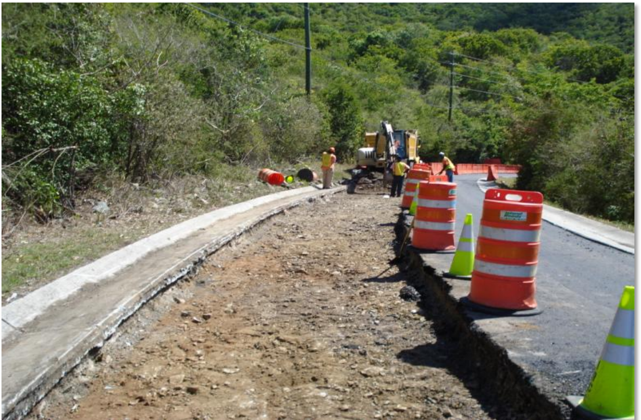
ROADWAY EXCAVATION AT STATION 107+00 (SCHEDULE A)
