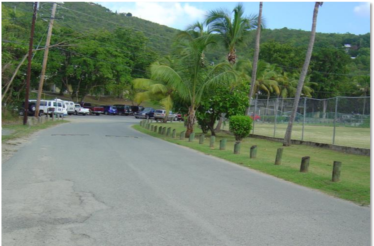
NORTH SHORE ROAD (ROUTE 10A) TOWARDS NPS HEADQUARTERS PARKING LOT BEFORE CONSTRUCTION
