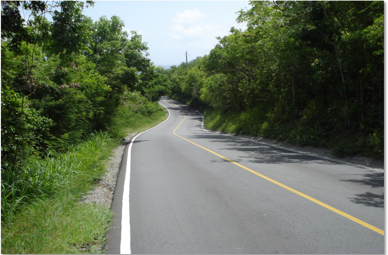
ADDITIONAL EDGE PAVEMENT MARKINGS AT STATION 119+00
