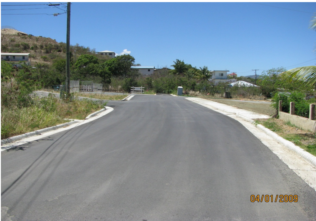
LINE 32 - PHASE COMPLETED
