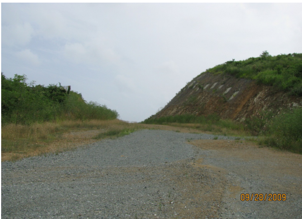
CUT C - LOOKING EAST AT STATION 79+00 COMPLETED FOR THIS PHASE
