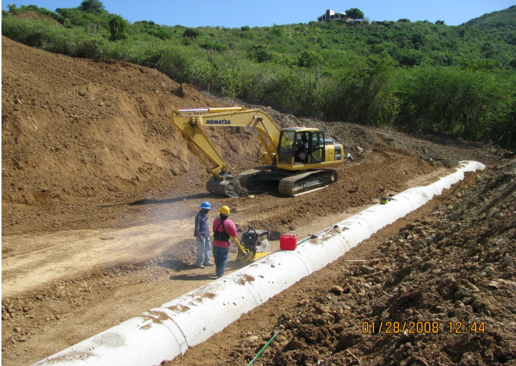
STATION 86+00 BACKFILLING AND COMPACTING 42-INCH RCP
