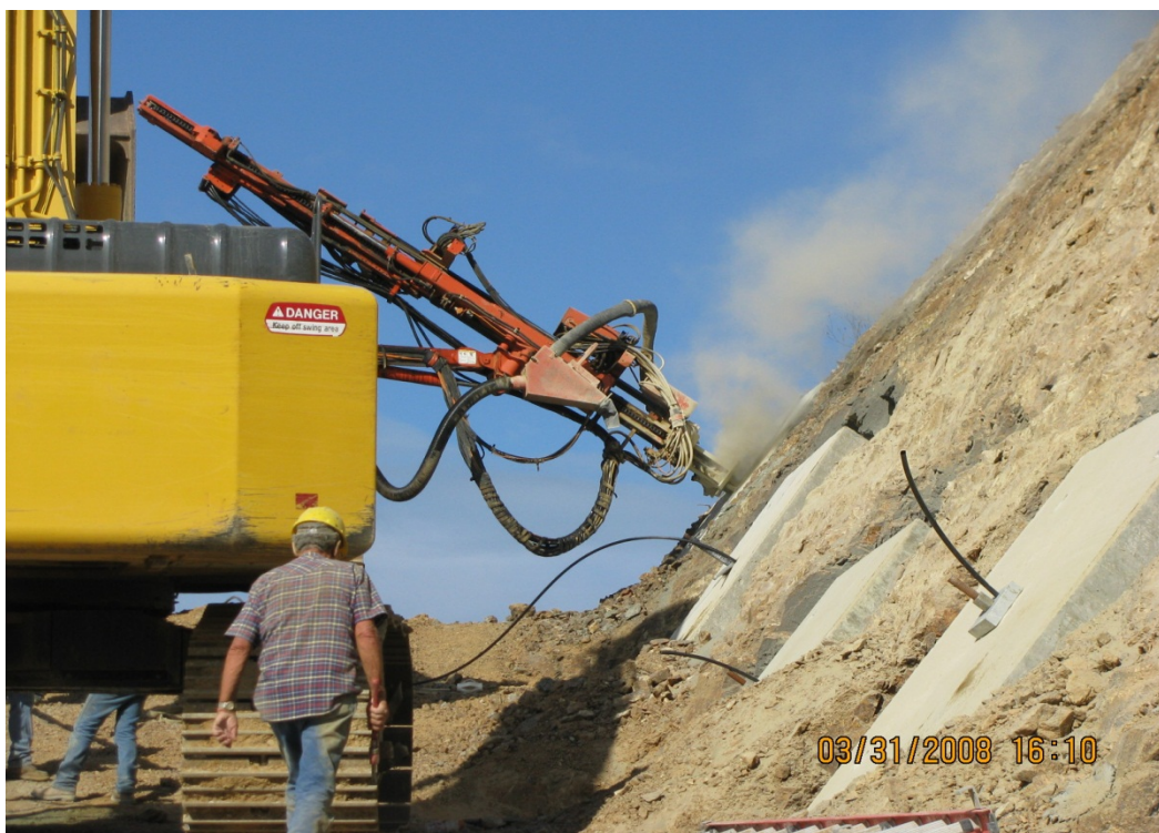
CUT C - STATION 82+50 INSTALLING ANCHOR BLOCKS, BOLTS, AND GROUTING
