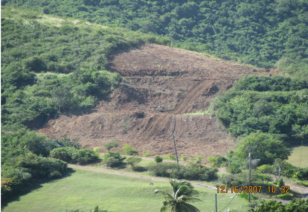
CUT B - CLEARED, BEGINNING OF THE CONSTRUCTION AT STATION 98+00
