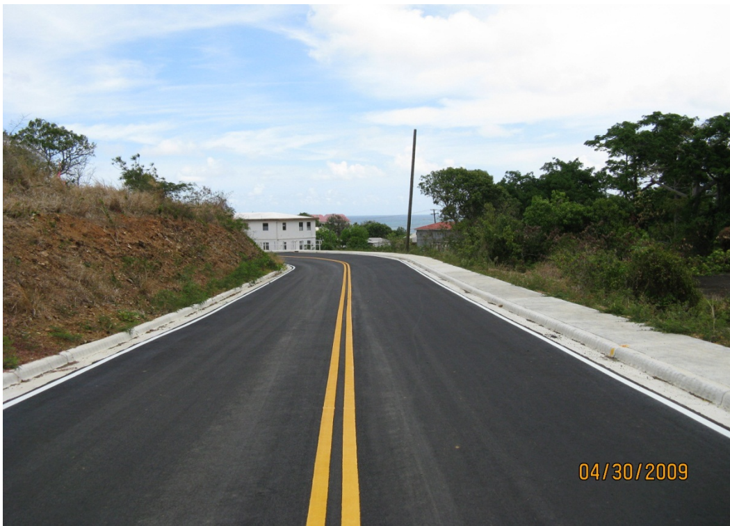
LINE 20 - STATION 3+50 KINGS CROSS STREET COMPLETED
