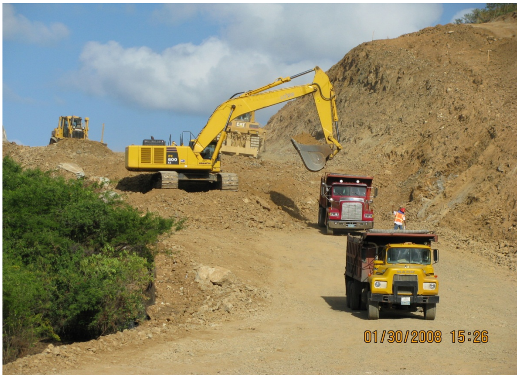
CUT C - LOOKING EAST AT STATION 80+00 EXCAVATION
