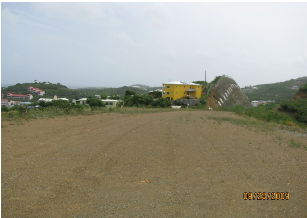
STATION 86+00 FILL AREA BETWEEN CUT B AND CUT C LOOKING EAST COMPLETED FOR THIS PHASE
