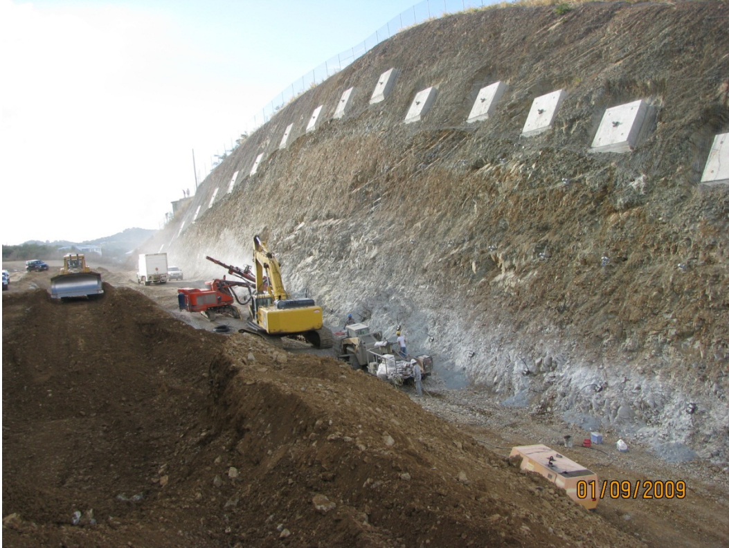
CUT B - STATION 94+00 EXCAVATION, DRILLING, AND INSTALLING ROCK BOLTS
