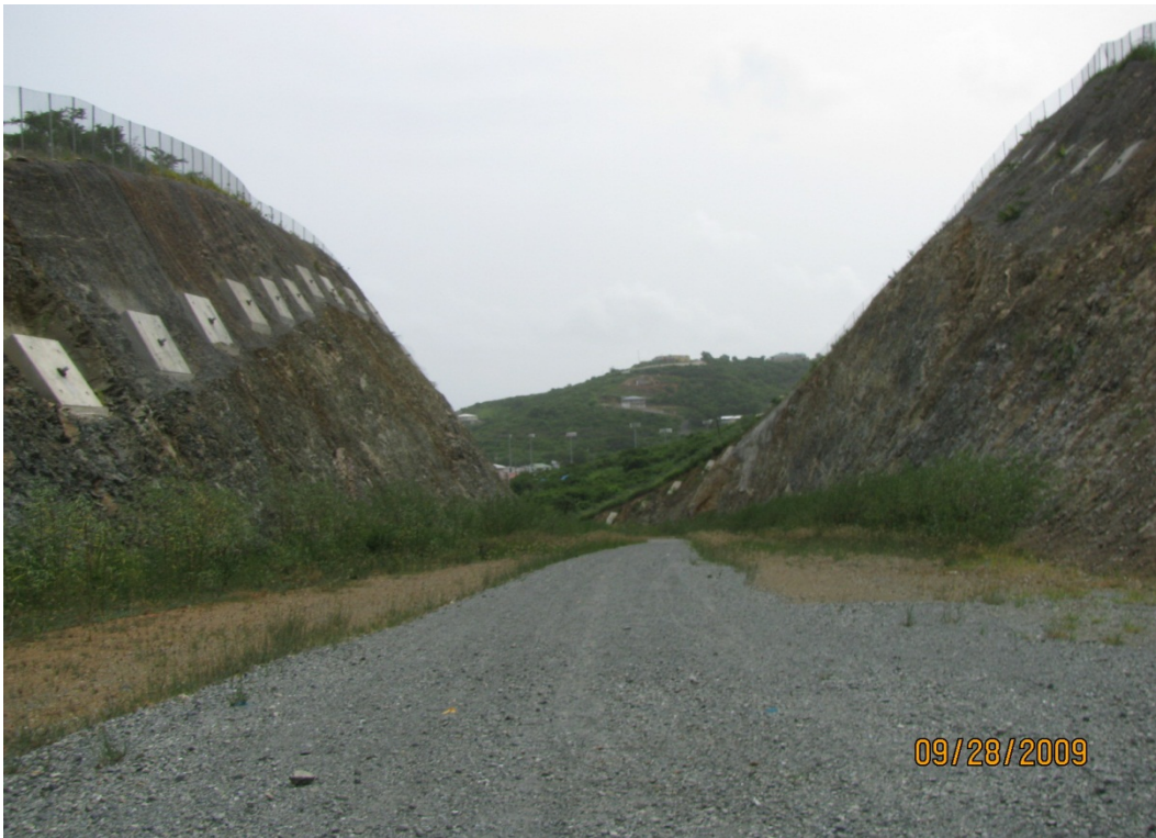
CUT B - LOOKING EAST AT STATION 88+00 COMPLETED FOR THIS PHASE
