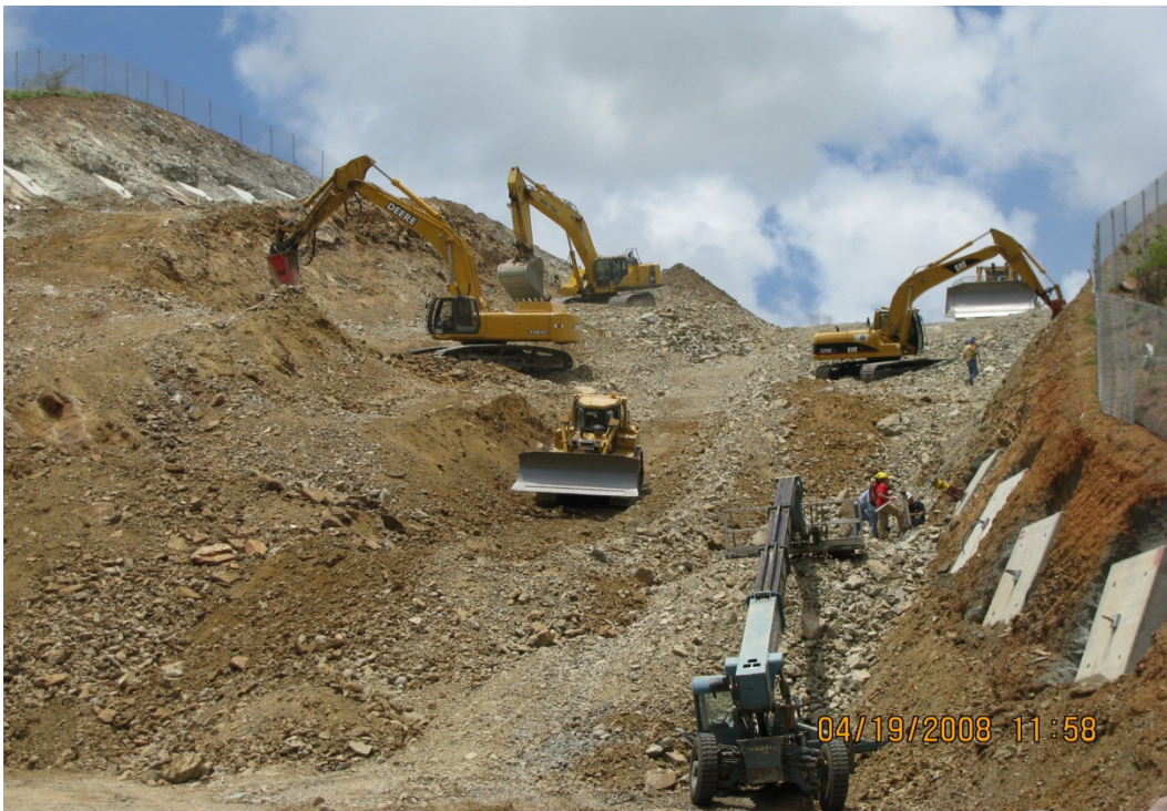
CUT B - EXCAVATION AND TESTING OF GROUND ANCHORS AT STATION 95+50
