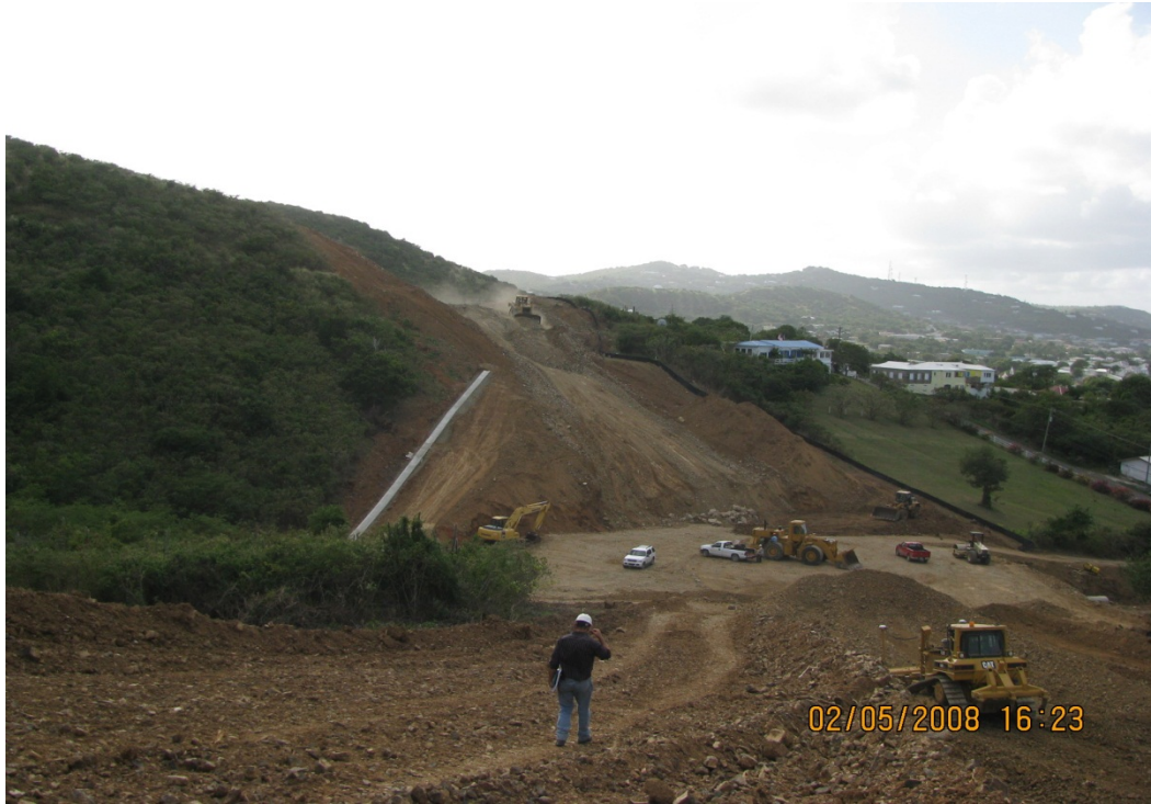
EXCAVATING FROM BOTH CUT B AND CUT C TO FILL AREA OF STATION 86+00
