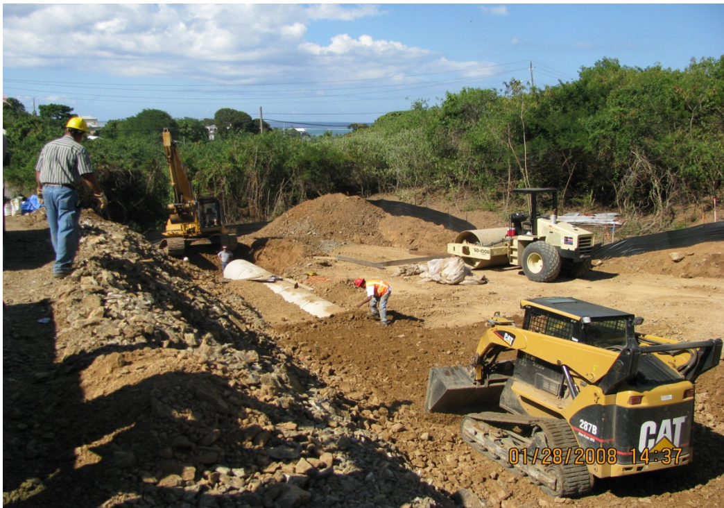
STATION 86+00 INSTALLING AND BACKFILLING 42-INCH RCP
