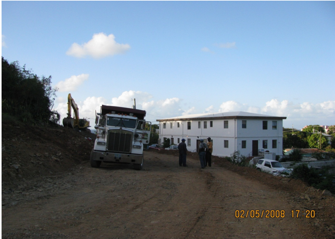
LINE 20 - KINGS CROSS STREET EXCAVATION FOR NEW ROAD ALIGNMENT
