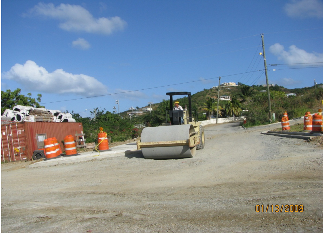
LINE 32 - COMPACTING AGGREGATE BASE PRIOR TO PAVING
