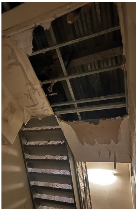
Figure 4 of 5: Charlotte Kimelman Cancer Institute (CKCI) Flying debris punctured the roof membrane during the 2017 hurricanes causing water infiltration resulting in interior damages and mold.
