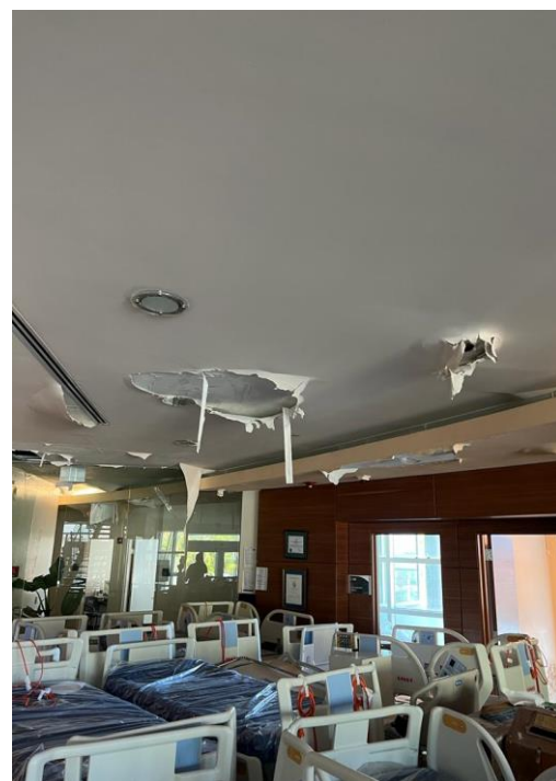
Figure 4 of 5: Charlotte Kimelman Cancer Institute (CKCI) Flying debris punctured the roof membrane during the 2017 hurricanes causing water infiltration resulting in interior damages and mold.
