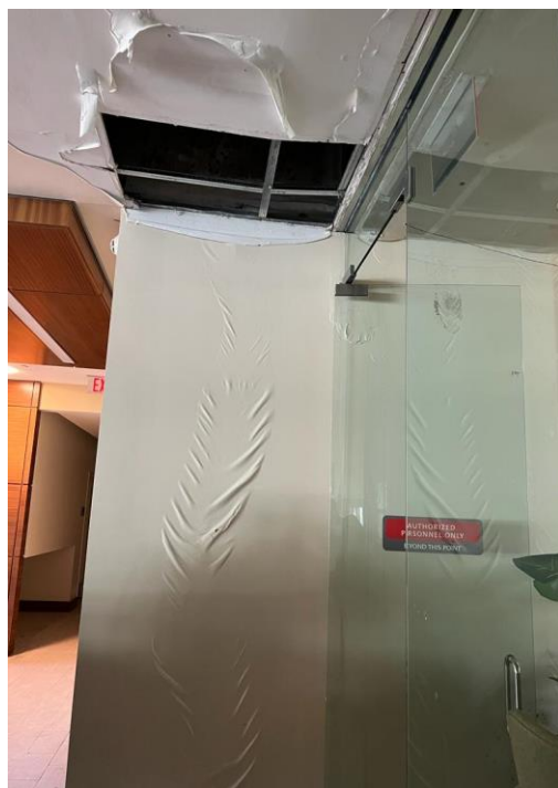
Figure 4 of 5: Charlotte Kimelman Cancer Institute (CKCI) Flying debris punctured the roof membrane during the 2017 hurricanes causing water infiltration resulting in interior damages and mold.
