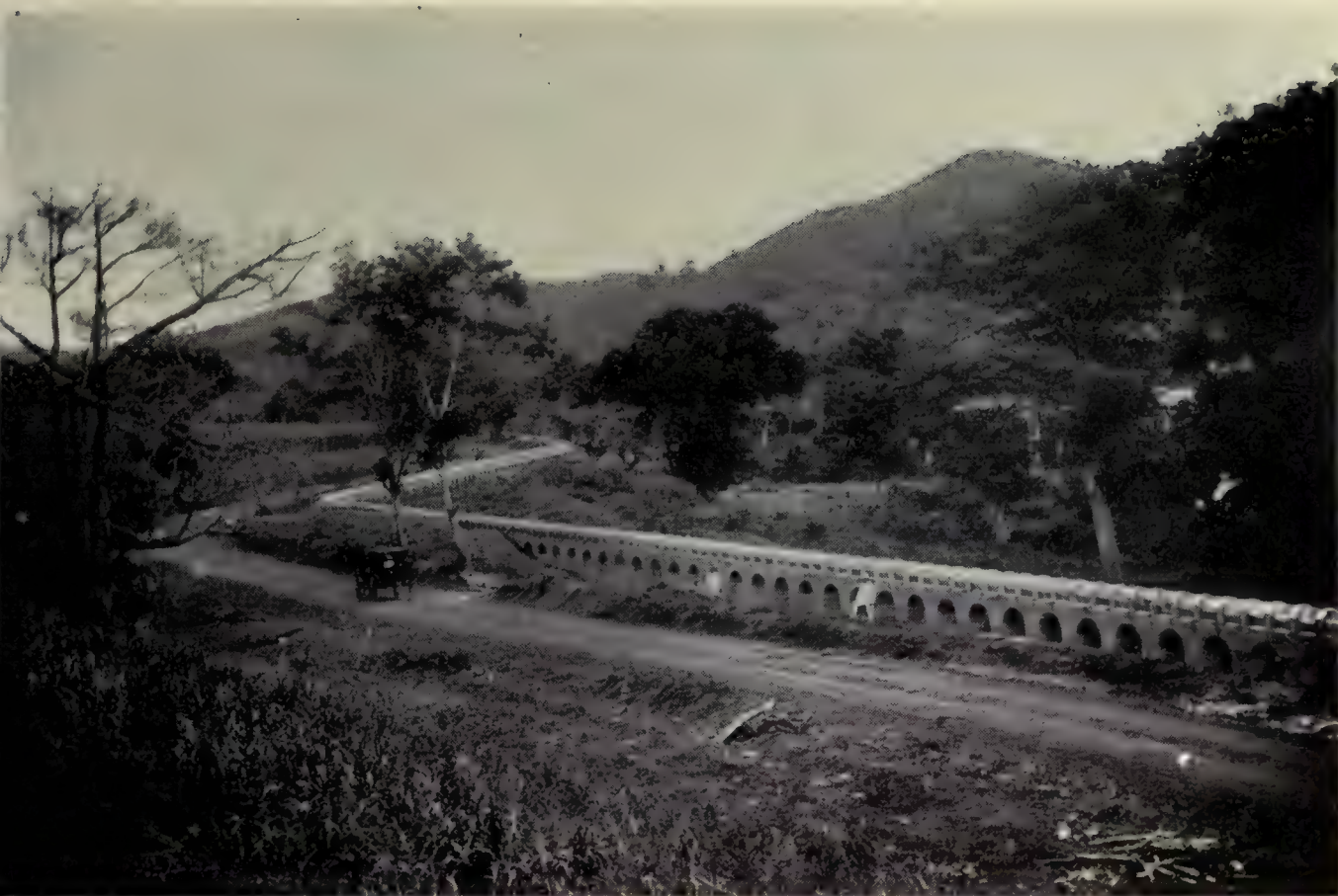
Water Aqueducts for Irrigation, St. Croix
