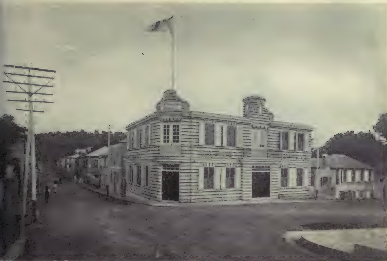
Cable Office, St. Thomas
