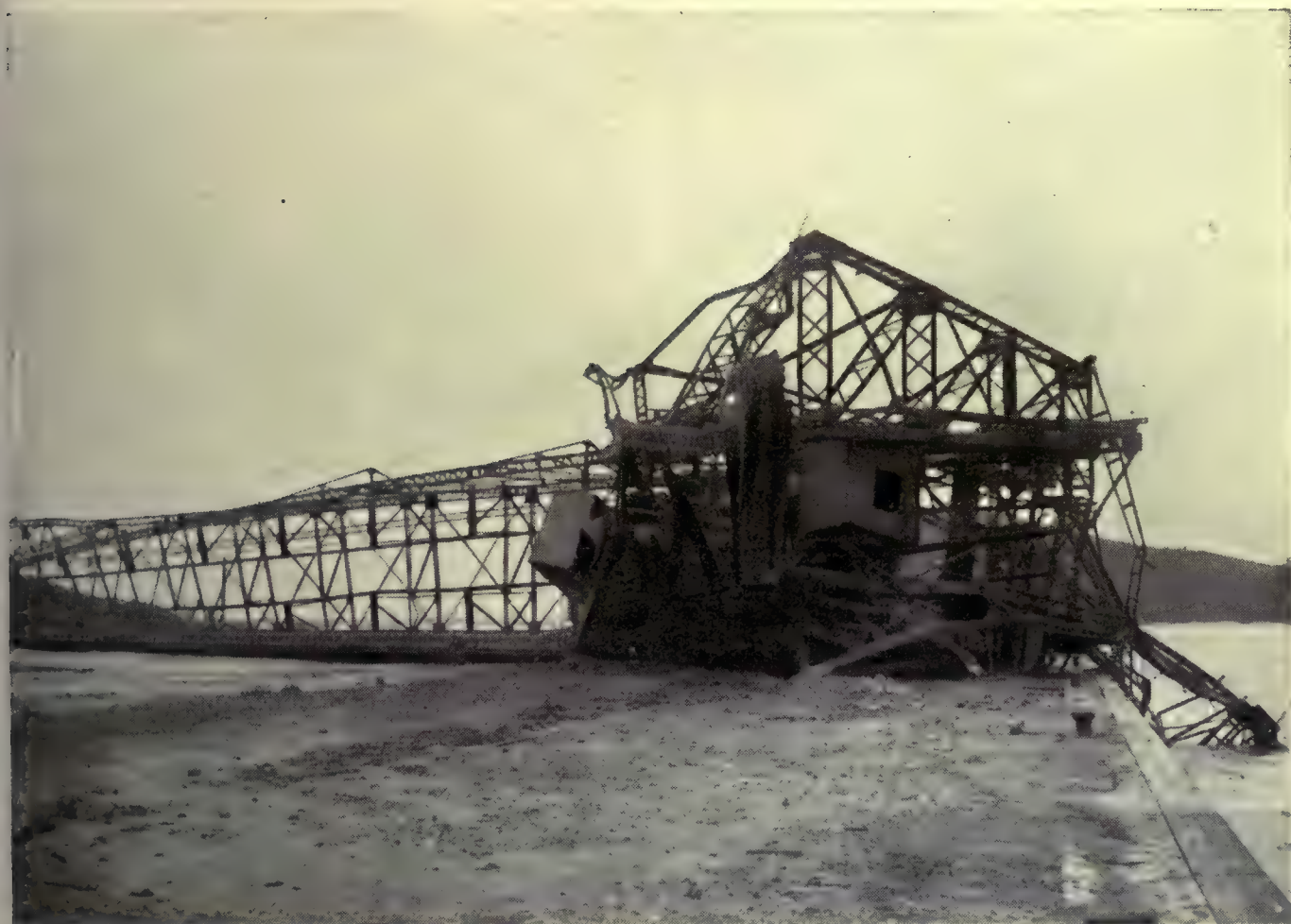
Huge Coal Crane Laid Low by Hurricane
