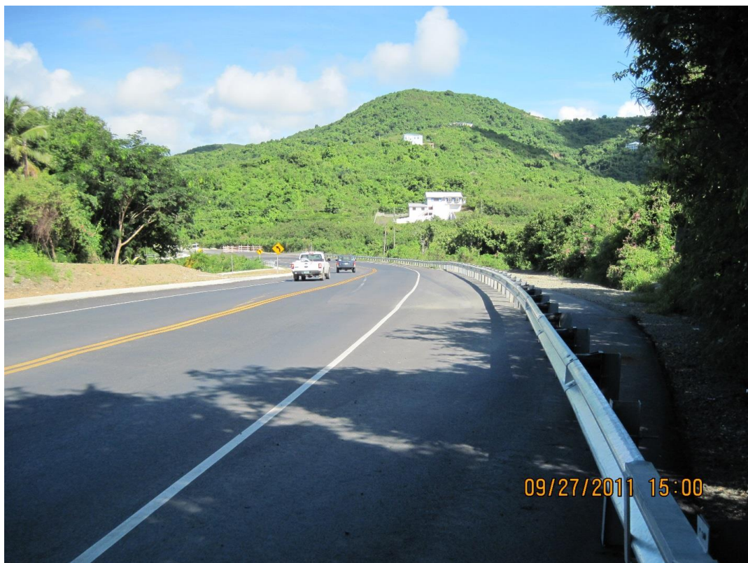
Looking north, newly paved section of Bypass, approximate Station 32+00
