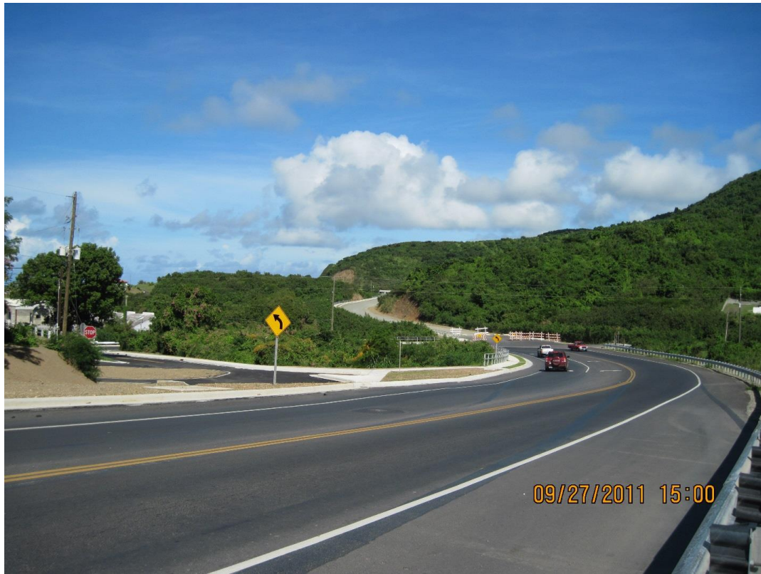
Looking north, newly paved section of Bypass. Parking area for historic site is on left.
