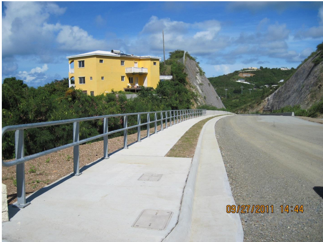
Looking north along the Bypass alignment, new aggregate base, curb, sidewalk, safety rails, etc.
