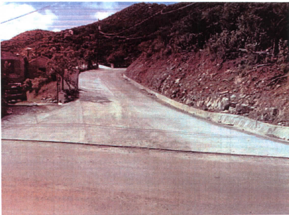
Project VINH 107(3), 108(1) Top photo shows existing conditions. Bottom photo shows As Built conditions. Photo taken of Route 108 at the Intersection of with Route 107.
